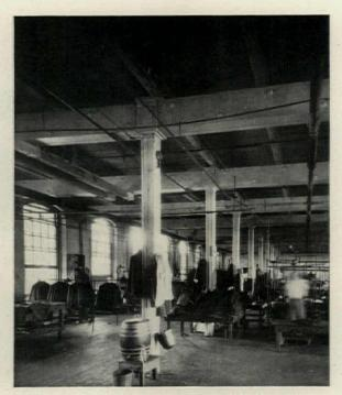
Interior of Clothing Factory, Erected 30 Years Ago, Showing Valuable Lighting Space Lost Above Windows Due to Type of Construction Then Prevalent
