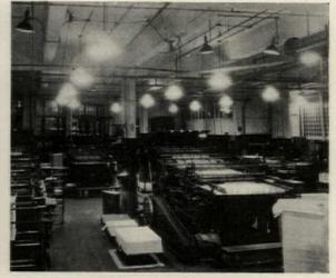
Color printing. Press room. General illumination. 300-watt clear lamps, diffuser. Spacing 12 x 12'. Lamps 12' above floor. Ceiling 14'. Illumination level 18 foot-candles. Projector type equipment with 200-watt daylight lamps. Color identification unit at inspection table. Waverly Press, Baltimore
