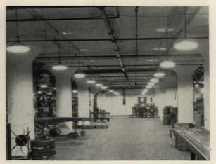
Hardware manufacturing. Blanking punch presses. 150-watt white bowl lamp, dome reflector. Outlets 10 x 10'. Lamps 8' 6" above floor. Ceiling 10'. Walls and ceiling white. Illumination level 12 foot-candles. Russell & Erwin Co., New Britain, Conn.
