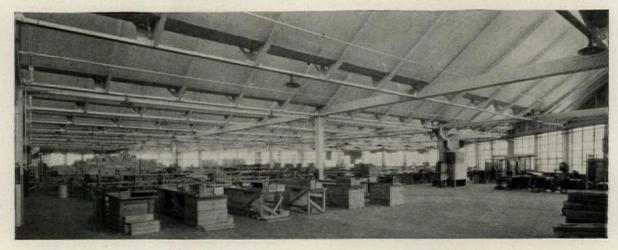
Interior of Modern Radio Manufactory of Atwater Kent Manufacturing Company, Using Super-span Sawtooth Skylight Showing Reflecting Value of Light Colored Roofing Material on Slope of Adjoining Sawtooth
