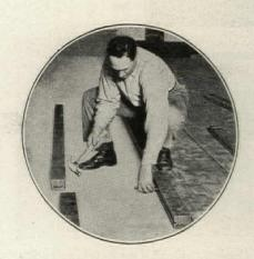
Bloxonend lays rapidly and can be installed in old plants with but slight interference to daily operations.
