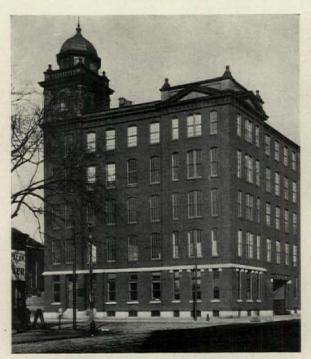
Clothing Factory, Erected 30 Years Ago. Wall and Window Spaces of Equal Width; 15 feet, 9 inches Story Height; 68 feet, 8 inches Wide
