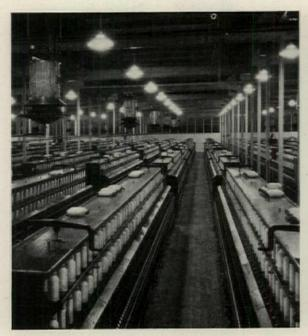
Textile mill. Spinning. 300-watt clear lamps, diffusing globes. Outlets spaced 14 x 21'. Lamps 12' above floor, ceiling 14'. Ceiling white, walls principally glass.
