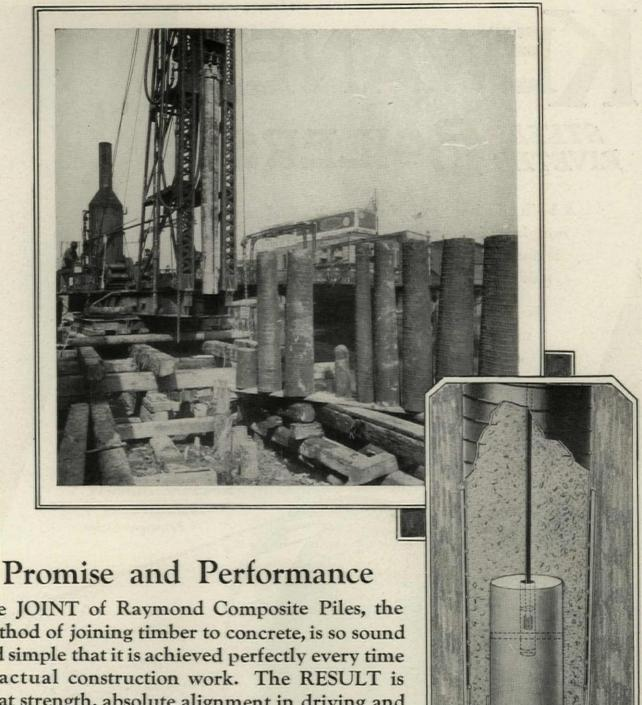
The JOINT of Raymond Composite Piles, the method of joining timber to concrete, is so sound and simple that it is achieved perfectly every time in actual construction work. The RESULT is great strength, absolute alignment in driving and assurance of perfect results in every one of these extra long piles.
