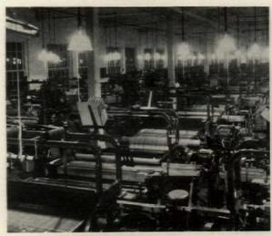
Silk mill. Weaving. 200-watt lamps, prismatic bowl reflectors. Outlets 6' centers in weaver's alley, 12' centers in rear alley. Lamps 9' above floor. Ceiling 13', ceiling white, walls white. Illumination level on work 25 foot-candles; on back of looms 6 foot-candles.
