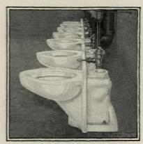
Showing a Battery of Universal Closets before the partition separating pipe chamber from toilet room is erected.
