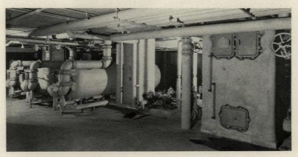
Hot Water Storage Heaters in Background. Boiler Feed Water Heater in Foreground
