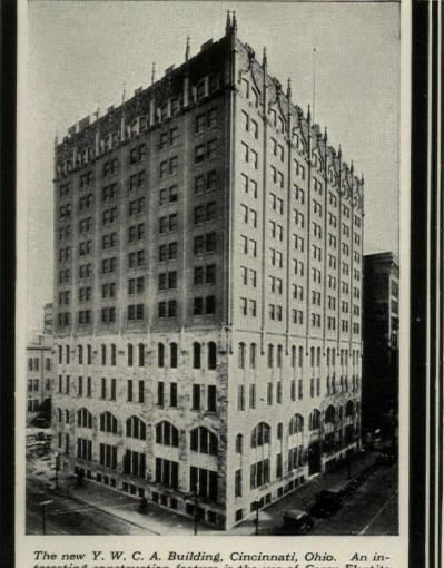
The new Y. W. C. A. Building, Cincinnati, Ohio. An interesting construction feature is the use of Carey Elastite Asphalt Plank, applied over a section of the Carey Builtup roof—an ideal roof promenade. —Rendigs, Panzer & Martin, Architects, Cincinnati, Ohio. F. B. & A. Ware Associate Architects, New York.
