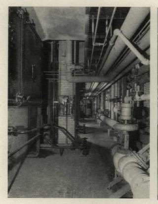
Rear of Boiler Room, High-pressure Steam Header
