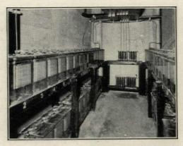
This reliable 60-cell Exide Battery protects general lights and exit lights to the extent of 28000 watts in new Atlantic City Convention Hall. The small Exide Battery in the background operates the fire alarm system.
