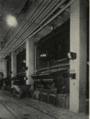
View of Boilers Showing Semi-automatic Stokers
