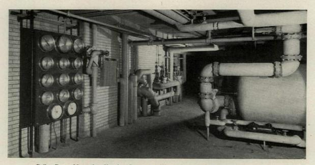
Boiler Room Mezzanine Showing Steam and Water Gauge Board, Recording Gauges and Water Pressure Reducing Valves
