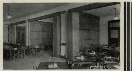
**CIRCLE** A Folding Partitions are a complete improvement over any folding partitions on the market. Mechanically operated by roller chains—not ropes or cable—hence the drive is positive. Patented hanging method insures easy operation. A special scaling system at floor, walls and ceiling effectively stops noise, odors and light. Doors are thoroughly insulated against sound.
