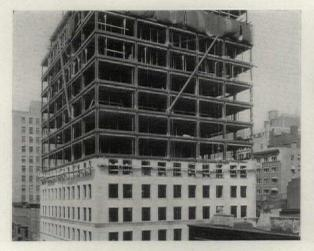
Type of Framing Suited to a Two-way Floor System. Necarsulmer & Lehlbach, Architects
