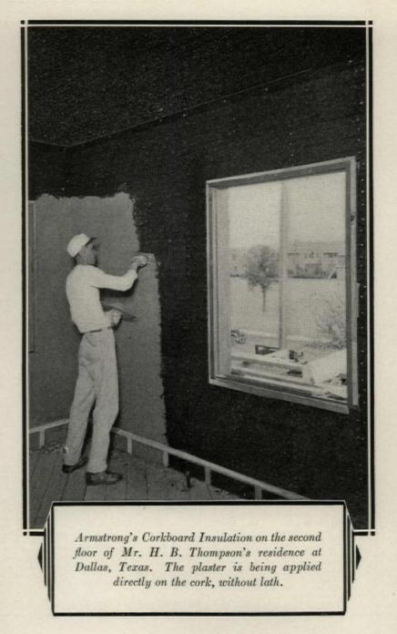
The full value of insulation, from both the comfort and the investment standpoints, is realized only when ample thickness is used. Two inches of Armstrong's Corkboard for the roof and at least one and a half inches for the walls is the most economical insulation in returns per dollar of cost. Armstrong Cork & Insulation Company, 900 Concord Street, Lancaster, Pa.; McGill Bldg., Montreal; 11 Brant St., Toronto, 2.
