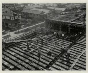
Metal Tile or Permanent "Tin Pans" Ready for the Pouring of the Concrete on a School Building in New Orleans
