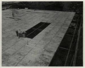
A Large Roof Area of Pre-cast Concrete Slabs Laid Over Railroad Yards in Hoboken
