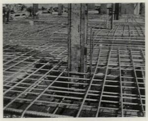
Typical Arrangement of Reinforcement for the Twoway System of Girderless Construction; the Steel Column Cores Are Used Only Through the Lower Stories of This Warehouse
