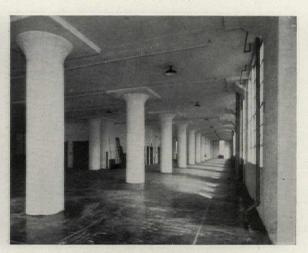
Typical Reinforced Concrete Girderless Floor Construction with Drops Over Columns and Half Drops at Walls. Cass Gilbert, Architect
