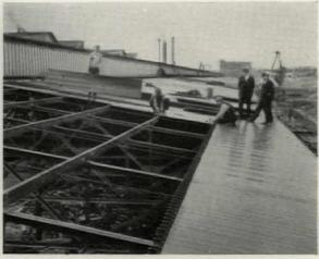
A Steel Deck Being Laid Over a Structural Steel Frame On An Ohio Factory
