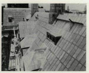
Short Span Gypsum Tile Laid Over a Structural Steel Frame on a Dormitory for Yale University
