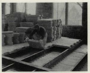
Pre-cast Gypsum Floor and Ceiling Blocks Used with Light Weight Rolled Steel Sections
