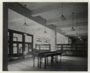
Typical Reinforced Concrete Beam-and-slab Construction as Designed for a New York Post Office.
