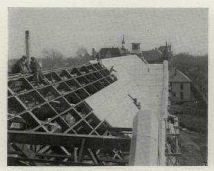
Gypsum Tile Being Placed Over a Structural Steel Frame on a College Building in Illinois
