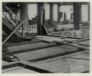
Wire Fabric in Place for the 4-inch Cinder Concrete "Arches" on an Office Building in New York
