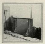
Rear of spandrel casting showing anchors attached
