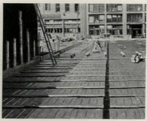
Removable Pans in Place on a San Francisco Garage; a "Bridging Joist" is Provided Along the Center Line of the Span
