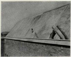
These Two Views Illustrate the Use of Reinforced Cinder Concrete Supported by a Structural Steel Frame.
