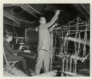
An Early Form of Nicholls Heat Flow Meter Used in Testing Roof
