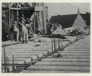
Concrete Rib Construction with Gypsum Block Used As Fillers on a Building in Baltimore
