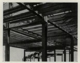
Light Weight Rolled Steel Sections Used with a Structural Steel Frame
