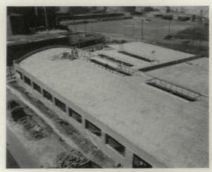
Gypsum Poured in Place Over a Thin Sheet of Compressed Gypsum Formed This Roof Surface
