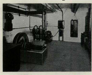
A YORK Refrigerating Machine may be installed at any convenient location in a building, and the refrigeration piped to various points where it is required.
