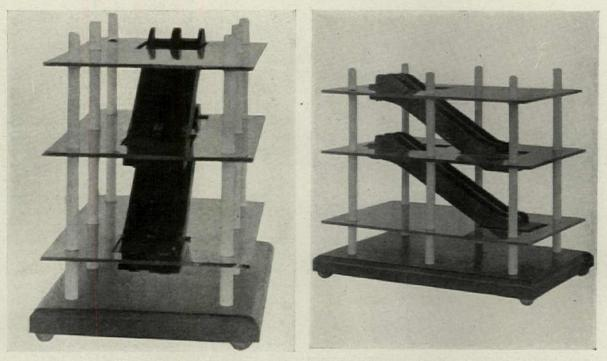
Model Showing Parallel Arrangement of Escalators in Center of Bay
