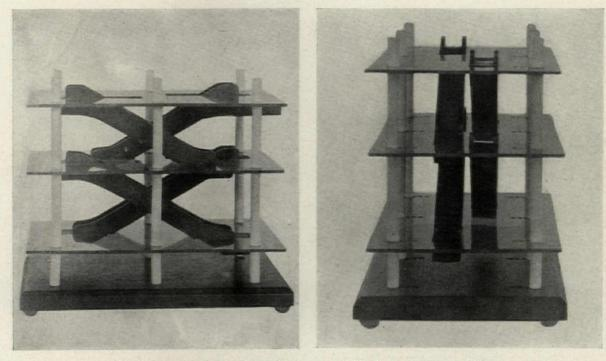
Model Showing Criss Cross Arrangement of Escalators in Center of Bay
