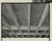
Note the clean-cut, good-looking joists when Meyer Steelforms are used. Meyter Steelforms are installed and removed by a trained organization. A nominal rental charge based on continued re-use of the starty steel forms covers installation and removal.
