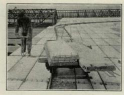
Method of tying Gypsteel Roof Slabs to give roof definite, computable, structural strength
