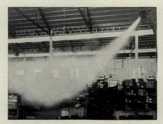
Another 5 Seconds and the heat has spread—along near the floor as far as 75 feet from the heater. Note that all the heated air is forced down into the working area.
