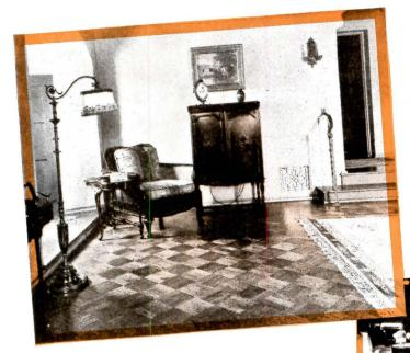
Style, permanence, lowest upkeep cost—combined in a floor of unique beauty. Each block is a complete unit of three or more oak flooring strips, full  $\frac{18}{16}$ <sup>m</sup> thickness, splined together. Laid quickly and easily in EVERBOND, a plastic cement without nails, directly over concrete or wood
