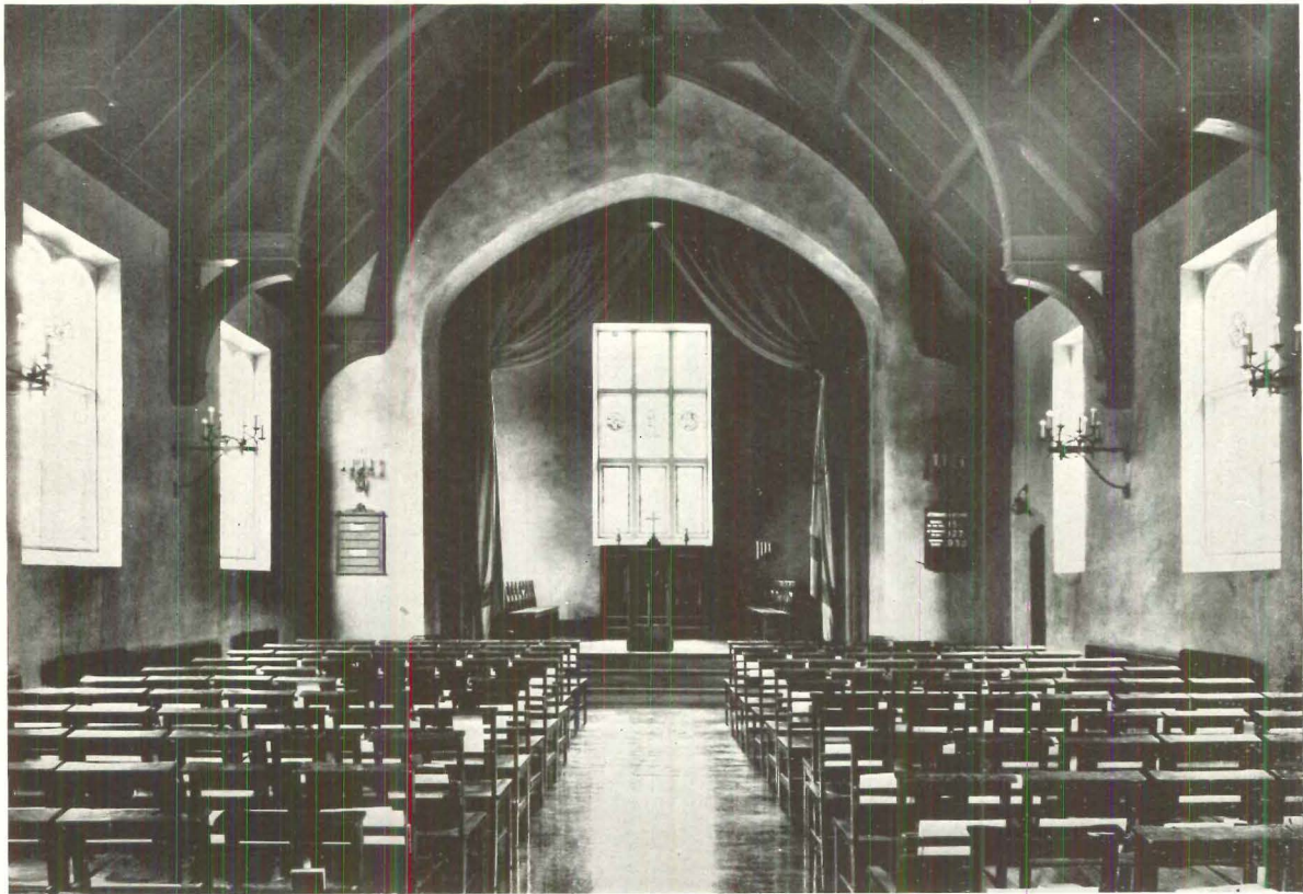
ST. JAMES' COMMUNITY HOUSE, WILMINGTON, N. C. HOBART B. UPJOHN, ARCHITECT
