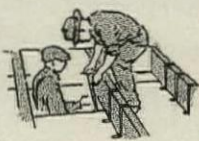
Hanging ceiling slabs
