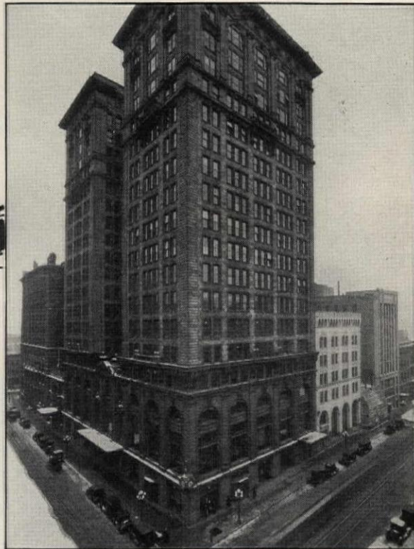
Above: First National- Soo Line Bldg.
