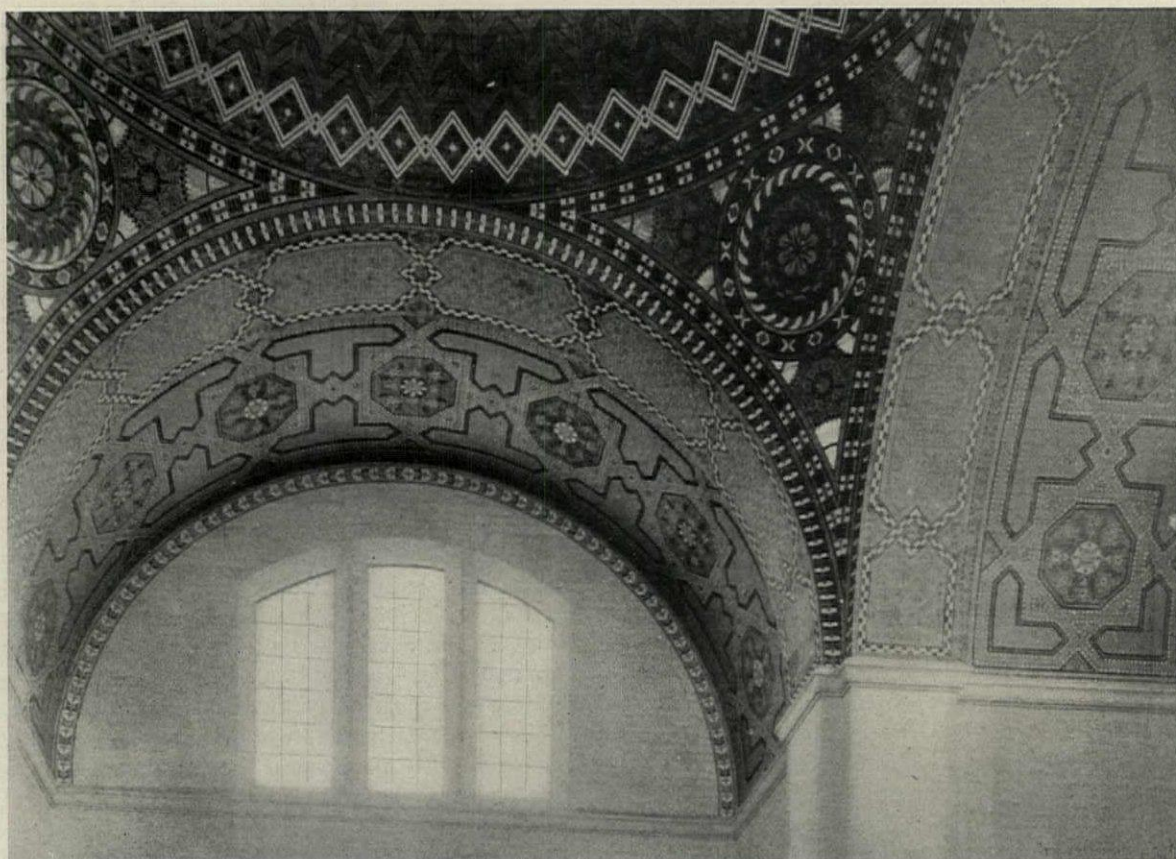
Intricate Stenciling has been Used Effectively on the Monolithic Concrete in the Los Angeles Public Library Bertram Grosvenor Goodhue and Carleton Monroe Winslow, Associated, Architects
