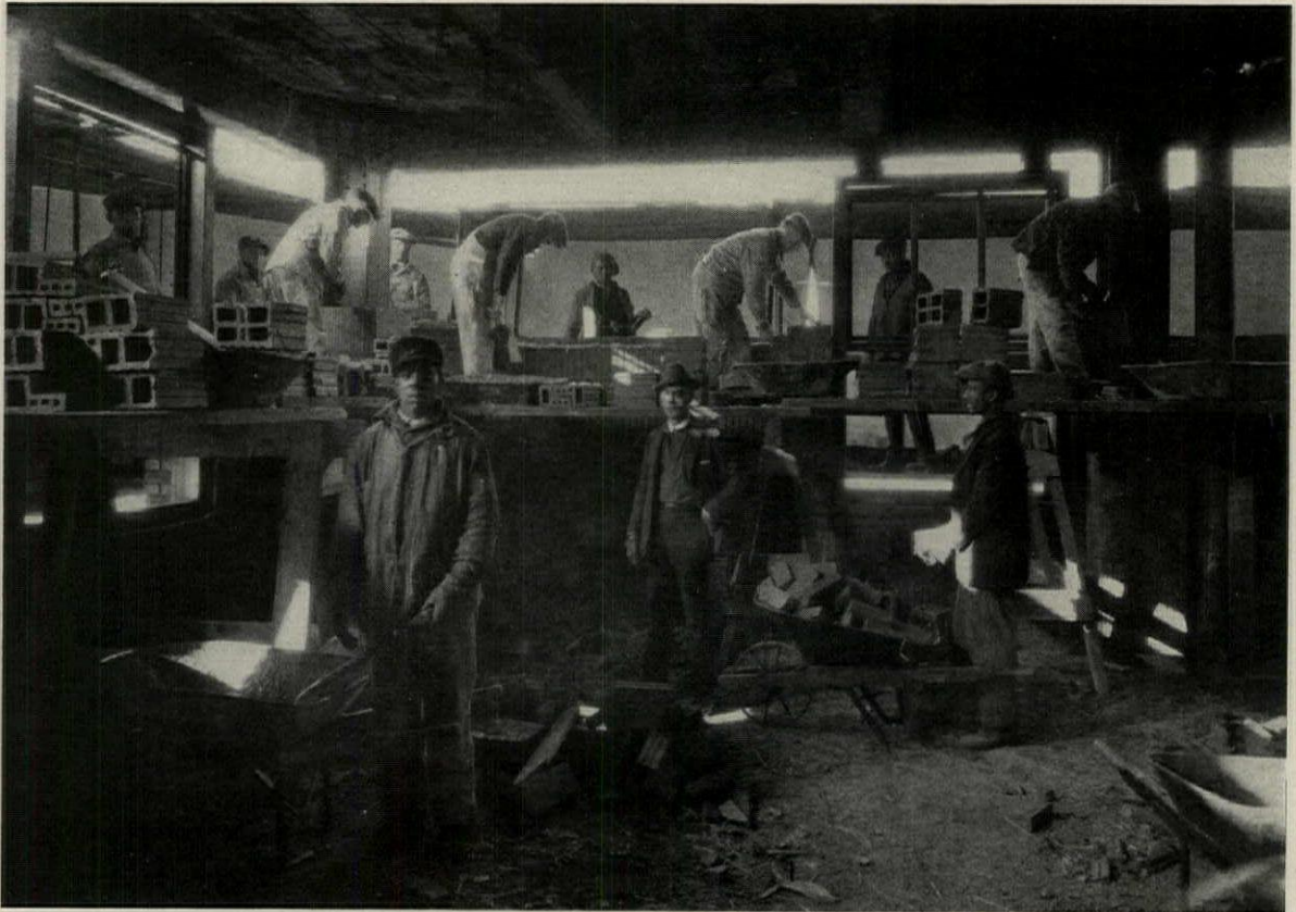
Anti-freezing Compounds and Adequate Cold Weather Precautions Required by the Specifications Permit the Maintenance of High Standards of Craftsmanship and Unchecked Progress
