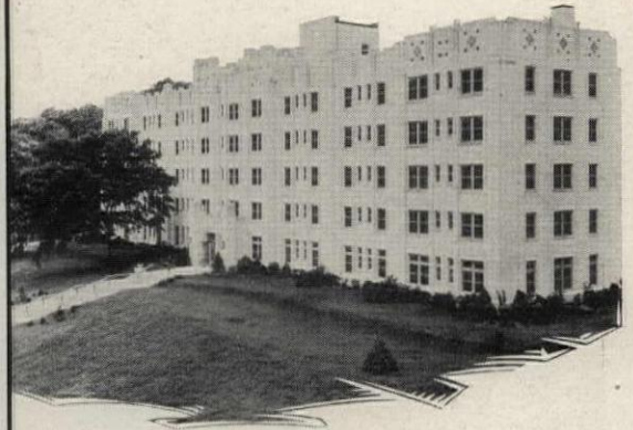
Architect, Henry P. Hess, St. Louis, Missouri
