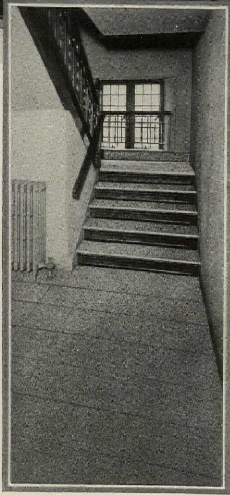
Stairway, hall and stair landings of Alberene Stone at Union Theological Seminary, New York, N. Y. ALLEN N. COLLINS, Boston, Architect.
