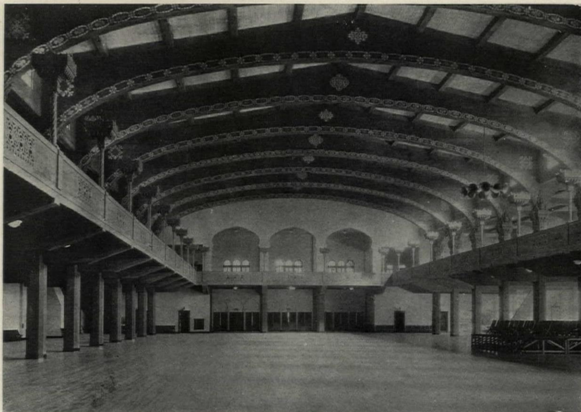
The Concrete Ribbed Ceiling in Al Malaikah Temple, Los Angeles, is Effectively Painted John C. Austin, Architect
