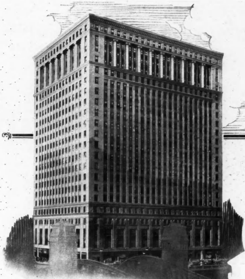
The Builder's Building, Chicago, Illinois, is equipped with American No. 130 Hot Galvanized Sash Chain—over 5 miles of it.
