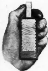
Cross-sectional sample of Compound construction, showing 3/16 inch sawn veneer tongue-and-grooved to core.
