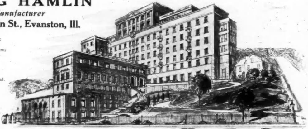
New $2,000,000 Montefiore Hospital, Pittsburgh, Pa., is HAMLINIZED Schmidt, Garden & Erickson, Architects
