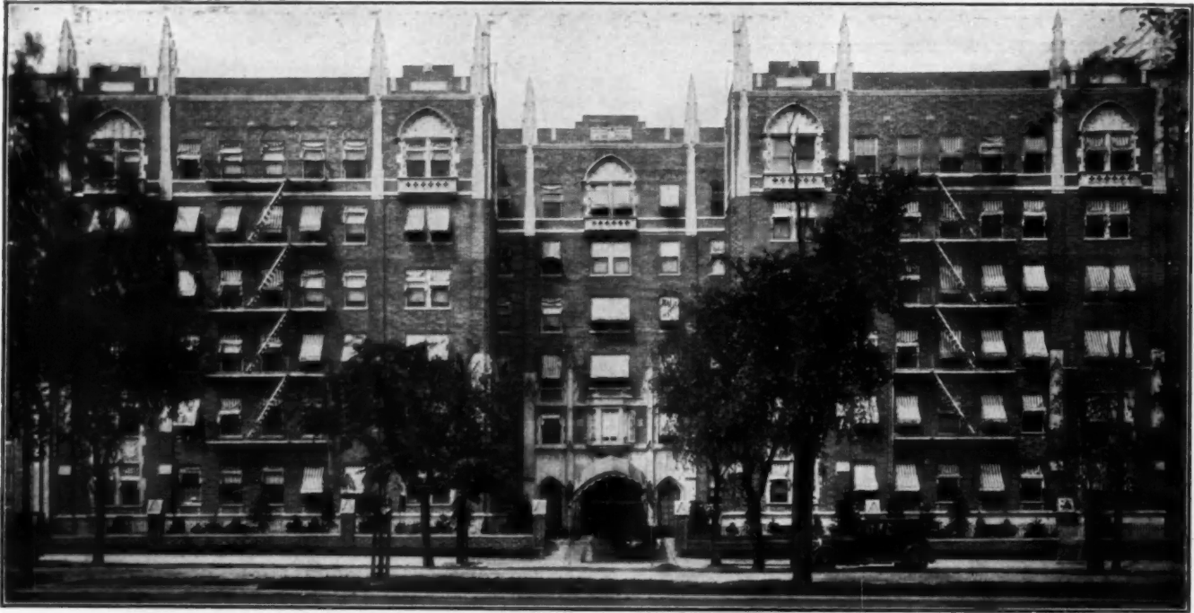
In many of America's finest buildings, of which the attractive Woodrow Wilson Apartments at Brooklyn, N. Y., is a good example, Wheeling Pipe is used. Architects: Shampin & Shampin, Brooklyn, N. Y.; Contractors: E. J. O'Brien & Bro., Brooklyn, N. Y.
