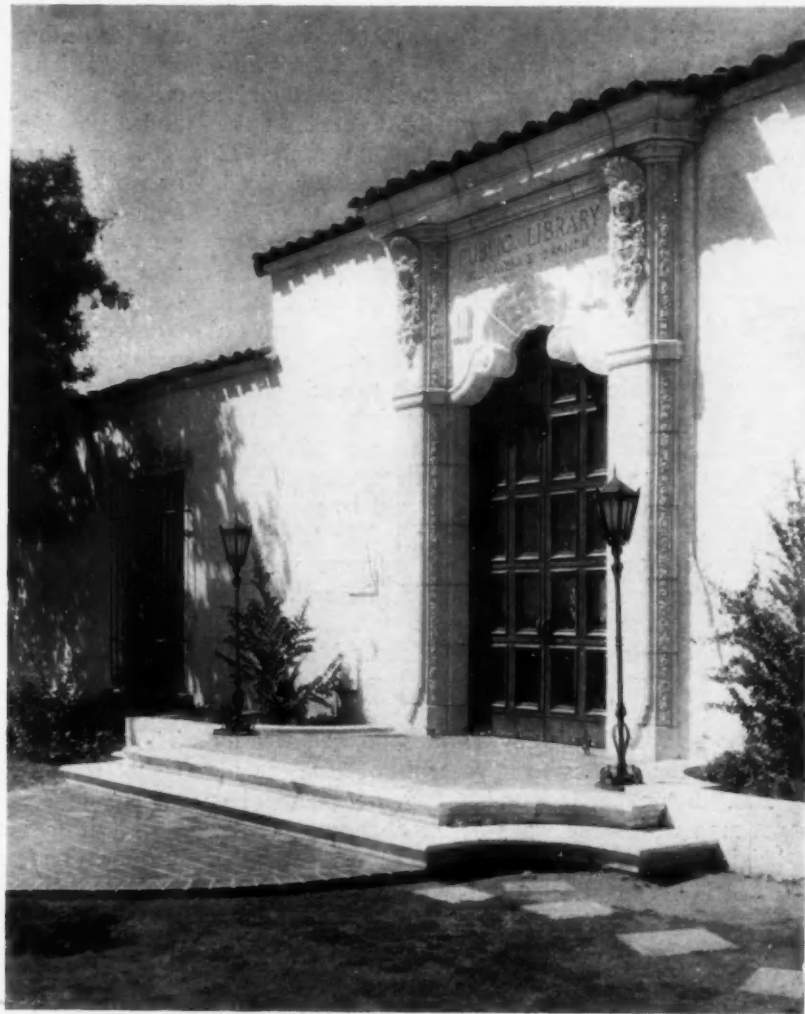
Hill Avenue Branch Library, Pasadena Maraton, Van Pelt & Maybury, Architects
