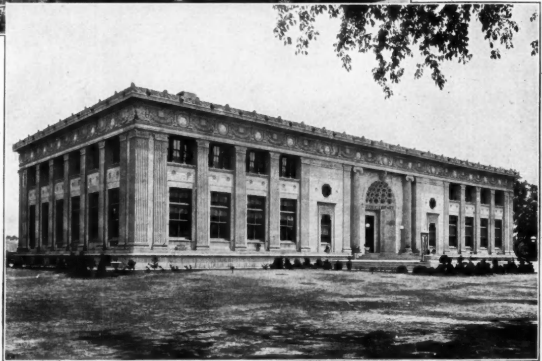
McGregor Library, High- land Park, Detroit. Tilton & Githens, Architects. Built of Gray Indiana Limestone.
