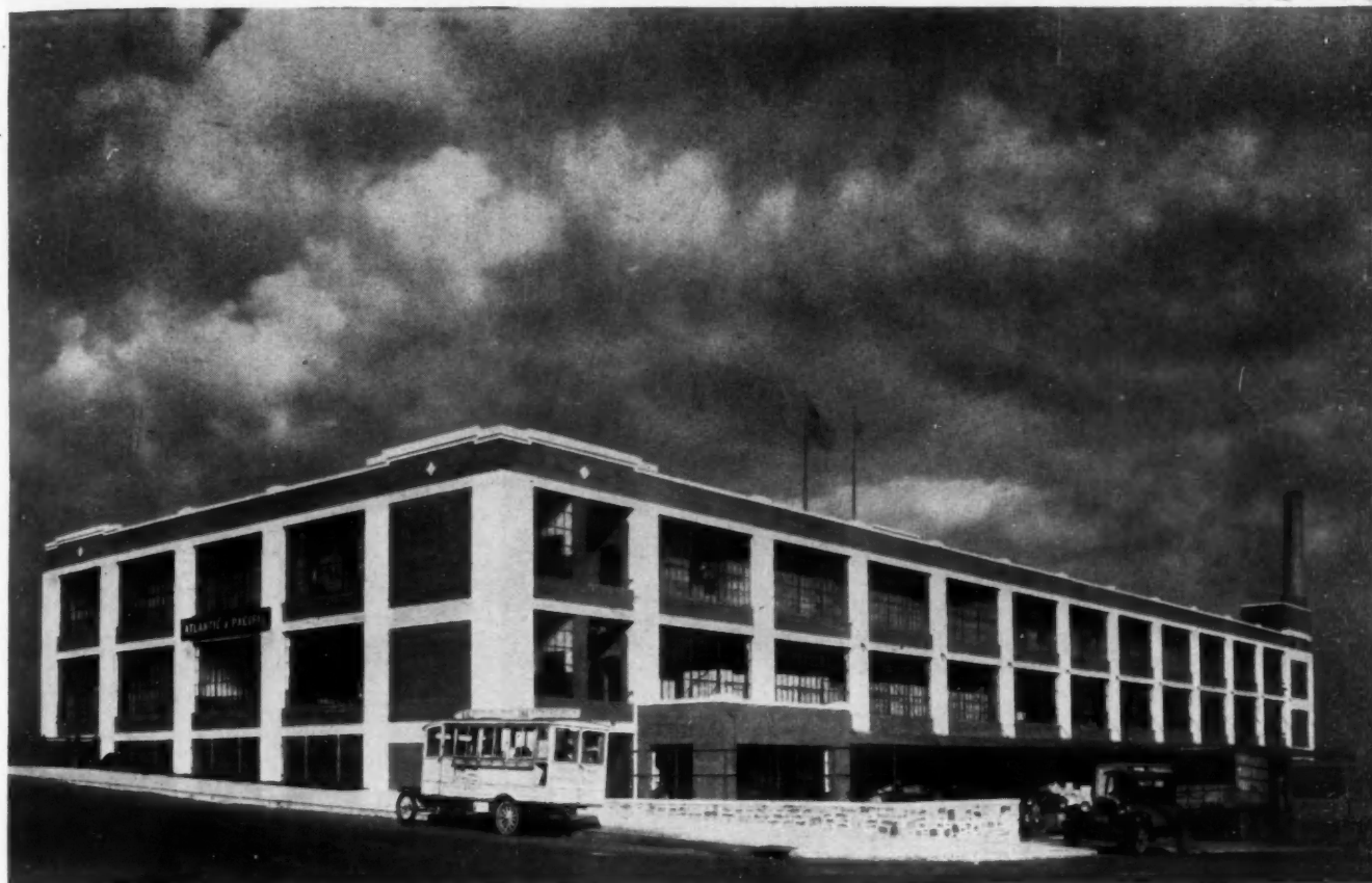
[[ The Philadelphia Warehouse of the Atlantic & Pacific Tea Company— heated by Heggie-Simplex equipment ]]
