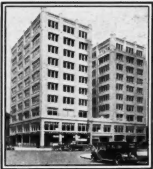
Detroit — Stephenson Building
