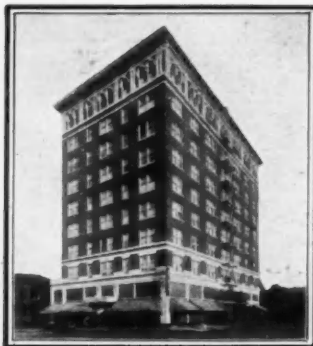
Oakland — Medical Arts Building
