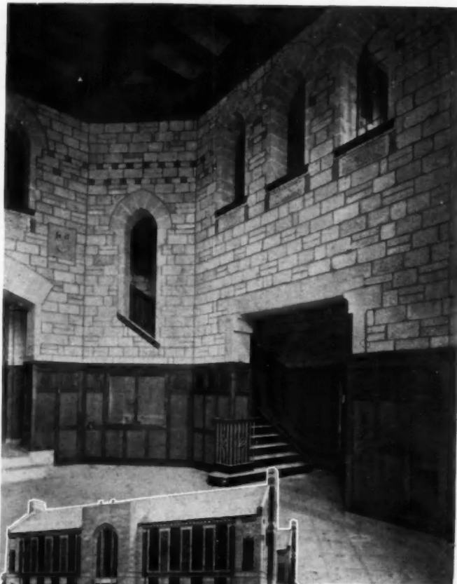
Chemistry Building at Michigan State College, Lansing, Michigan. Architects, Malcolmson and Higginbotham, Detroit, Michigan. Contractor, Fred C. Trier, Saginaw, Michigan.
