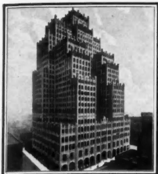
St. Louis — Bell Telephone Building
