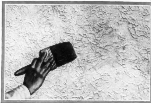
Apply the base coat of Johnson's Liquid Wax Glaze with an ordinary three-inch paint brush.
