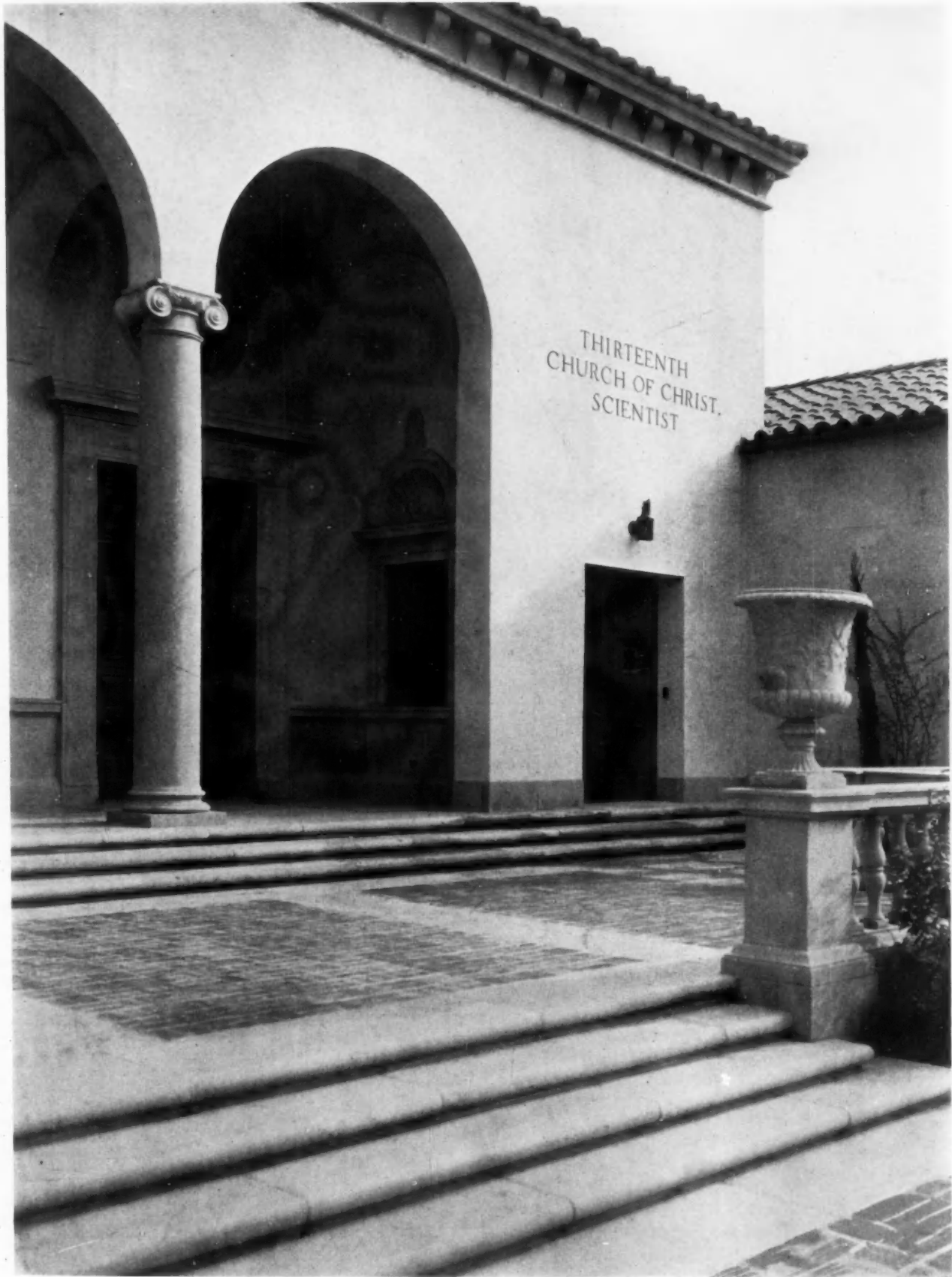
DETAIL OF PORTICO, THIRTEENTH CHURCH OF CHRIST SCIENTIST, LOS ANGELES ALLISON & ALLISON, ARCHITECTS
