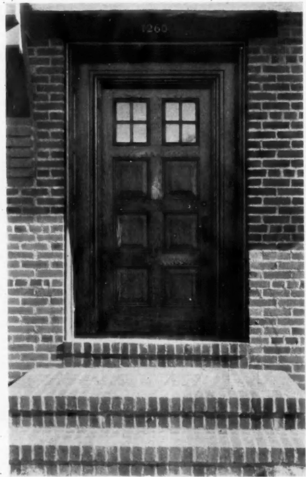
Detail of Entrance.
