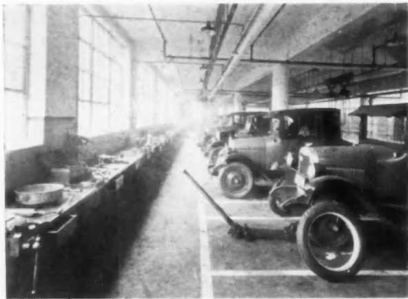
Wall Benches, Chevrolet Workshop, Detroit Albert Kahn, Inc., Architects
