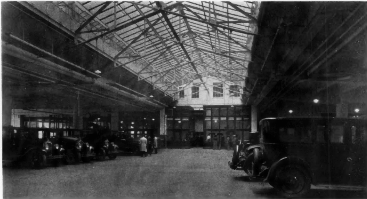
Service Room and Parking Area, Packard Garage, Philadelphia Phillip S. Tyre, Architect
