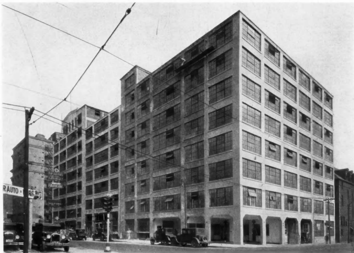
One of the New Buildings for The Detroit Garages, Inc.
