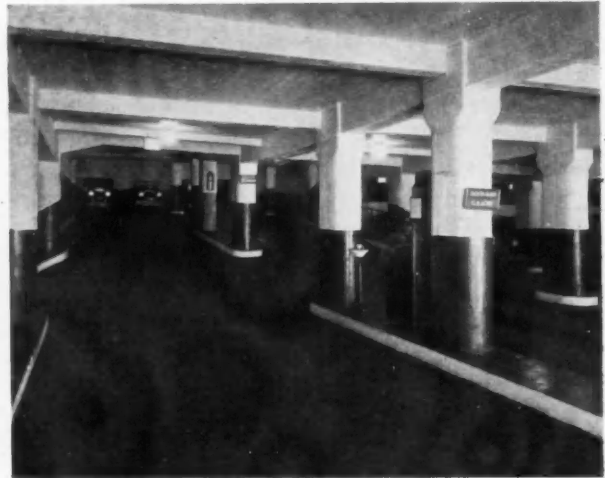
Up and Down Ramp, East Unit Garage
