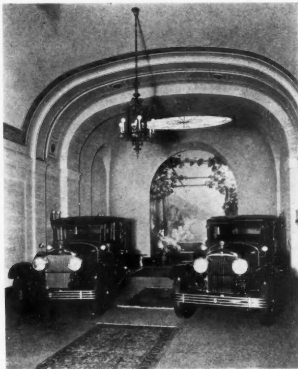
Sales Room, Cadillac Corporation, New York Charles E. Birge, Architect
