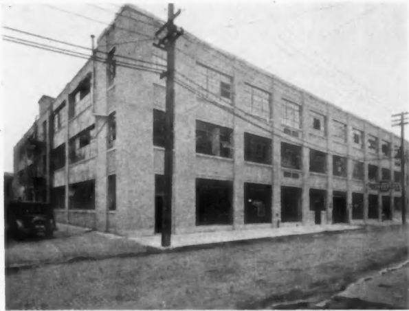
Accessories and Garage Building, Detroit Albert Kahn, Inc., Architects
