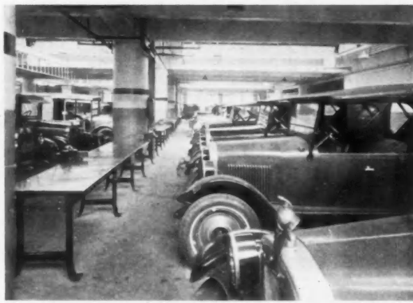
Another View in Chevrolet Workshop, Detroit Albert Kahn, Inc., Architects
