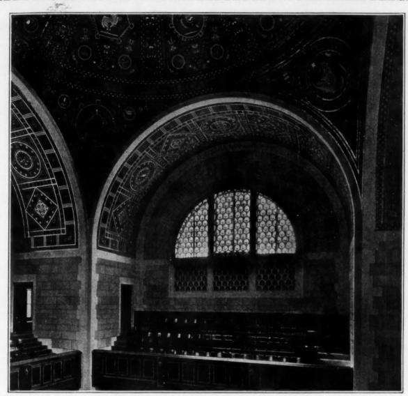
Vault and roof dome of Central Hall of the National Academy of Sciences, Washington, D. C. Guastavino's tile construction with soffit course of Akoustolith sound absorbing artificial stone, Bertram G. Goodhue, Architect
