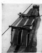
The Van Guilder Wallbuilder shown in place on walls is filled with semi-wet concrete and tamped. Lever indicated by arrow is then lifted, which collapses the center core and expands the outside plates, thereby freeing the concrete on all sides. The wallbuilder is then instantly slid forward.
