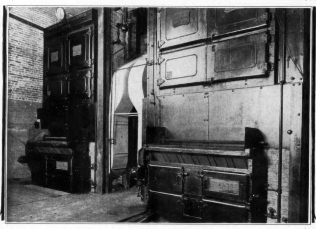
Two "King Coal" automatic mechanical stokers under two 250 hp. Kroeschell Boilers at the Riverside Brookfield High School, Riverside, Illinois.
