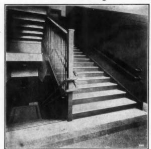
CTAIR treads and landings of Alberene Stone D have a smooth, but "toothed," surface that neither slips nor grips and gives an equally secure footing wet or dry.
