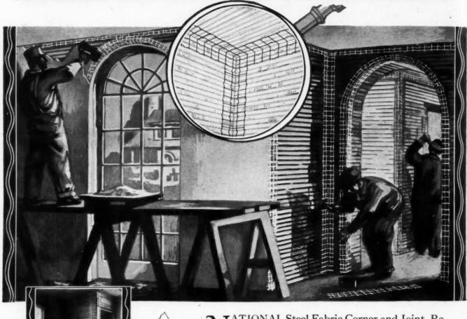
Application of Corner and Joint Reinforcements over wood lath.
