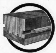
Bloxonend comes in 8 ft. lengths with the Southern Pine blocks dovetailed endwise onto baseboards. Laid directly over the old or new concrete or wood floors.
