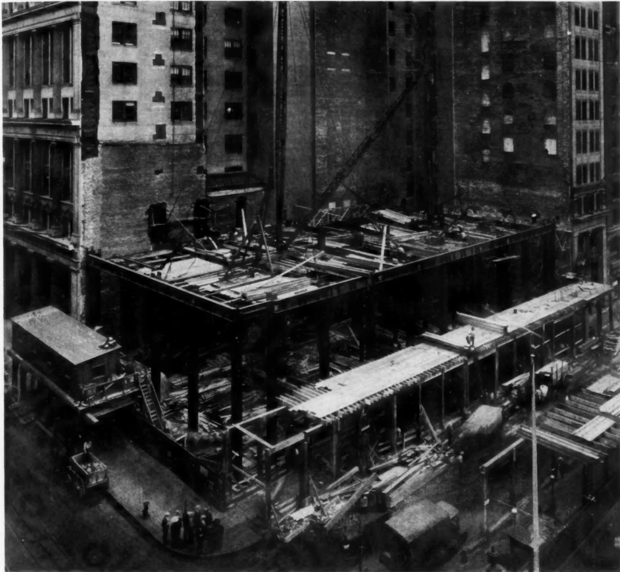
View Showing Holes in Old Wall Where Cantilever Trusses Were Inserted
