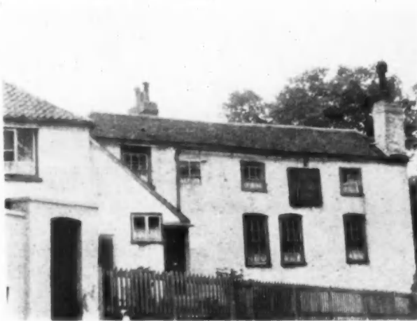
The "Spaniards," from the Highway
