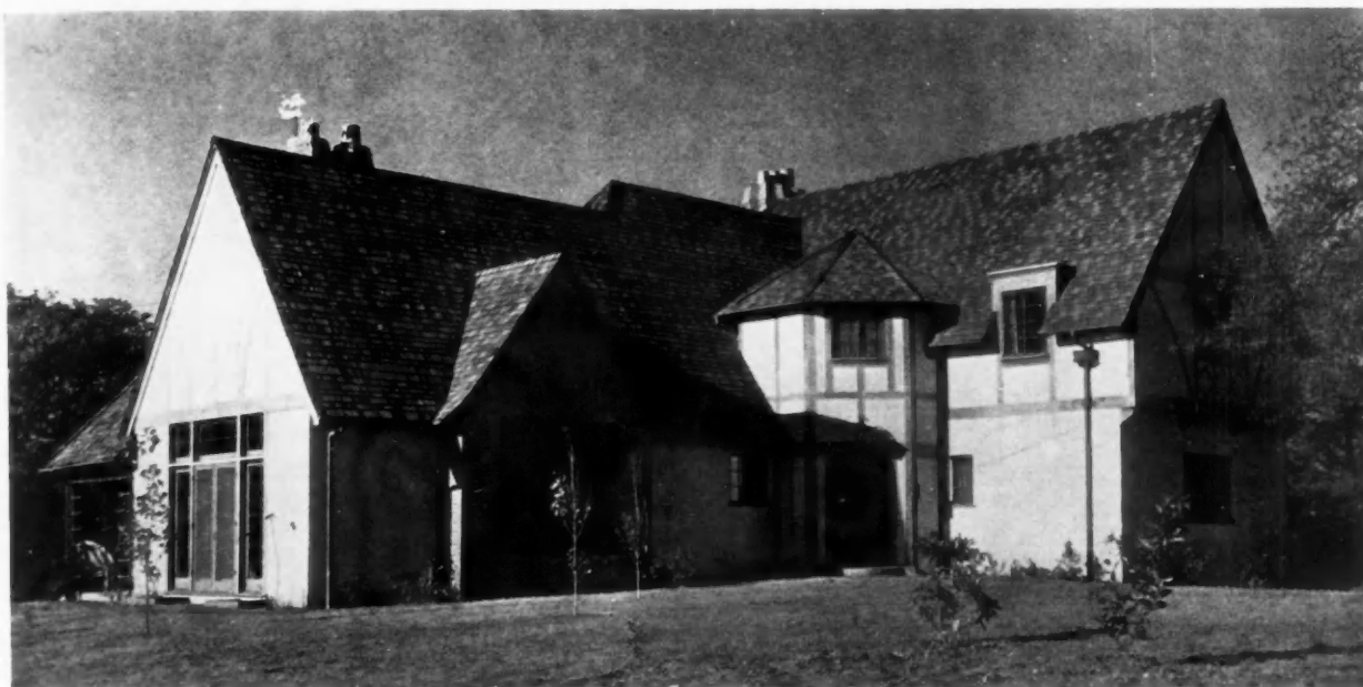
HOUSE OF J. T. PENTON, ESQ., PASADENA KENNETH A. GORDON, ARCHITECT
