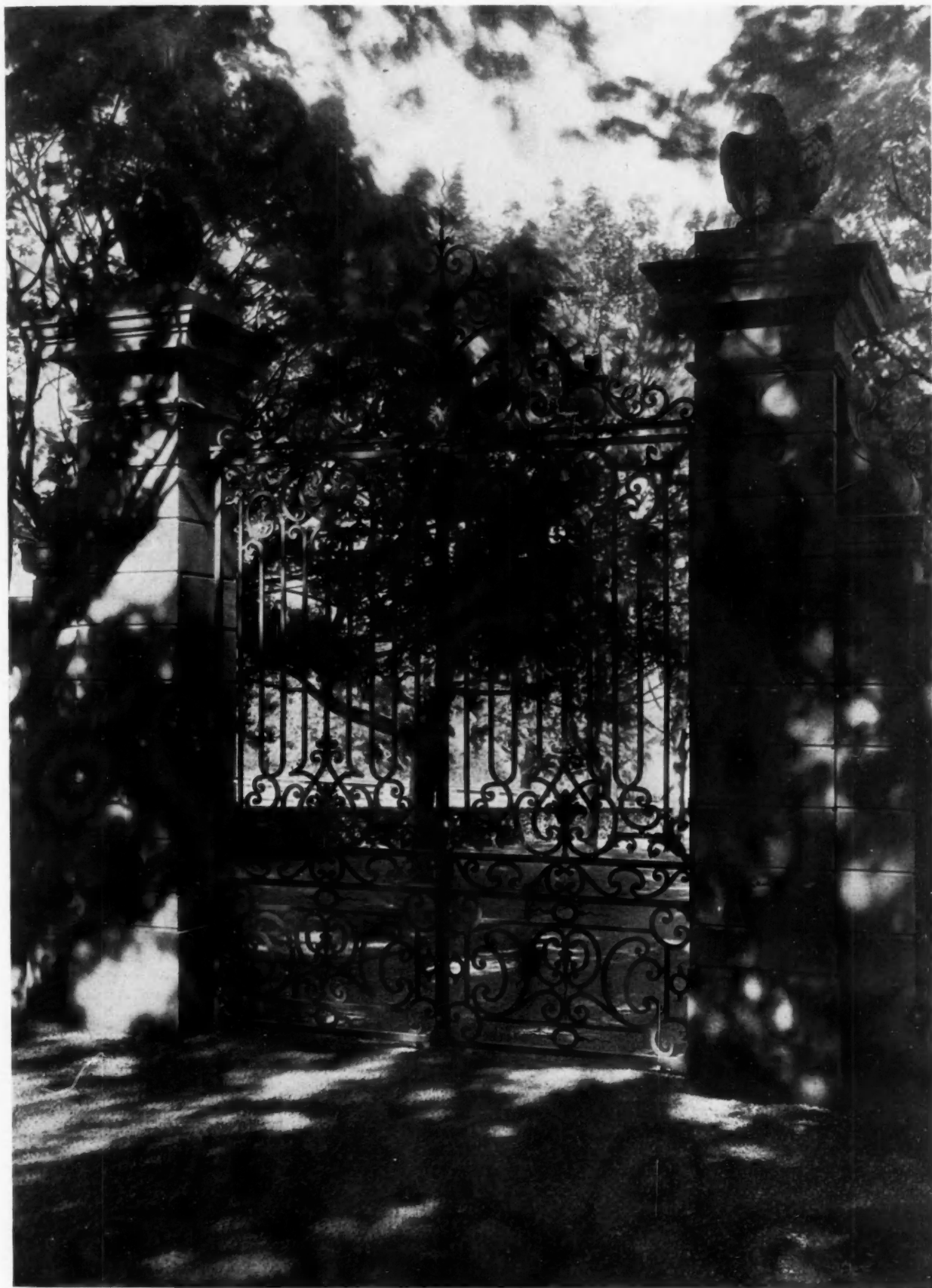
ENTRANCE GATES, ESTATE OF MOSES TAYLOR, ESQ., PORTSMOUTH, R. I. JOHN RUSSELL POPE, ARCHITECT
