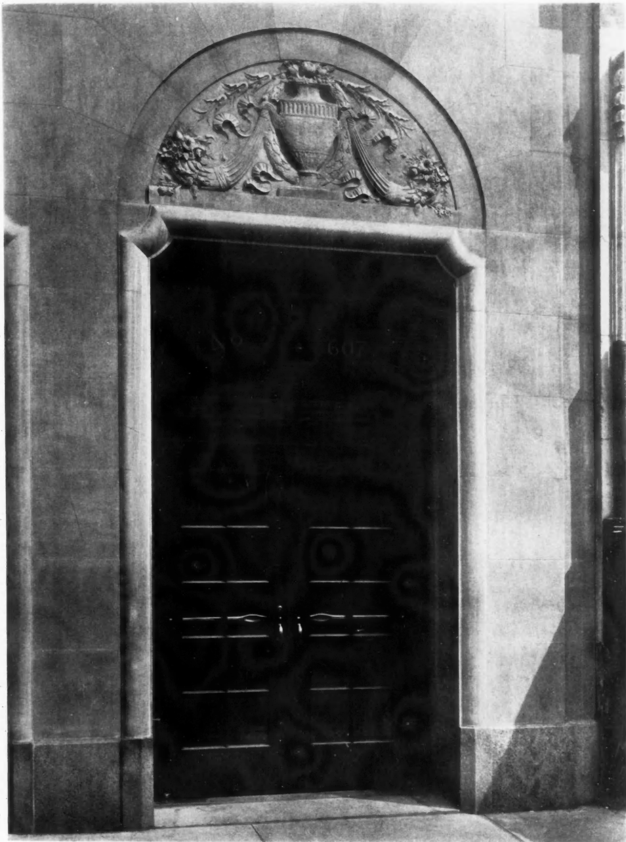
ENTRANCE, JAMES McCUTCHEON & CO. BUILDING, NEW YORK CROSS & CROSS, ARCHITECTS; STARRETT & VAN VLECK, ASSOCIATED
