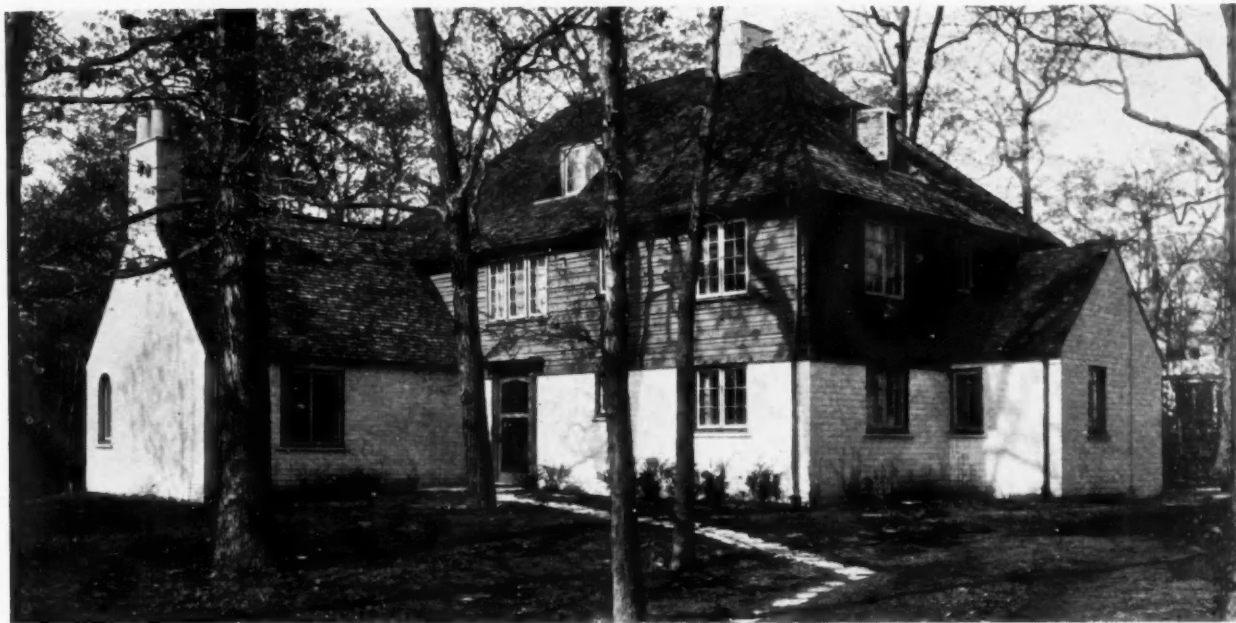
HOUSE OF E. B. BARTLETT, ESQ., WINNETKA, ILL. RUSSELL S. WOLCOTT, ARCHITECT
