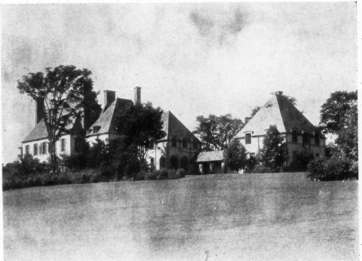
General View, Showing Garage and Servants' Wing
