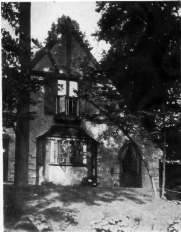
The Entrance Facade
