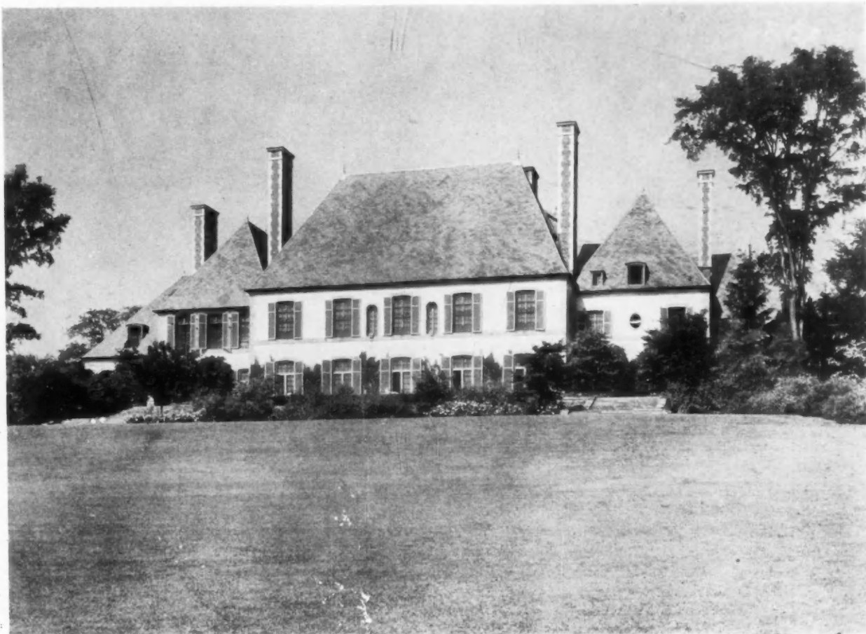
The Garden Facade
