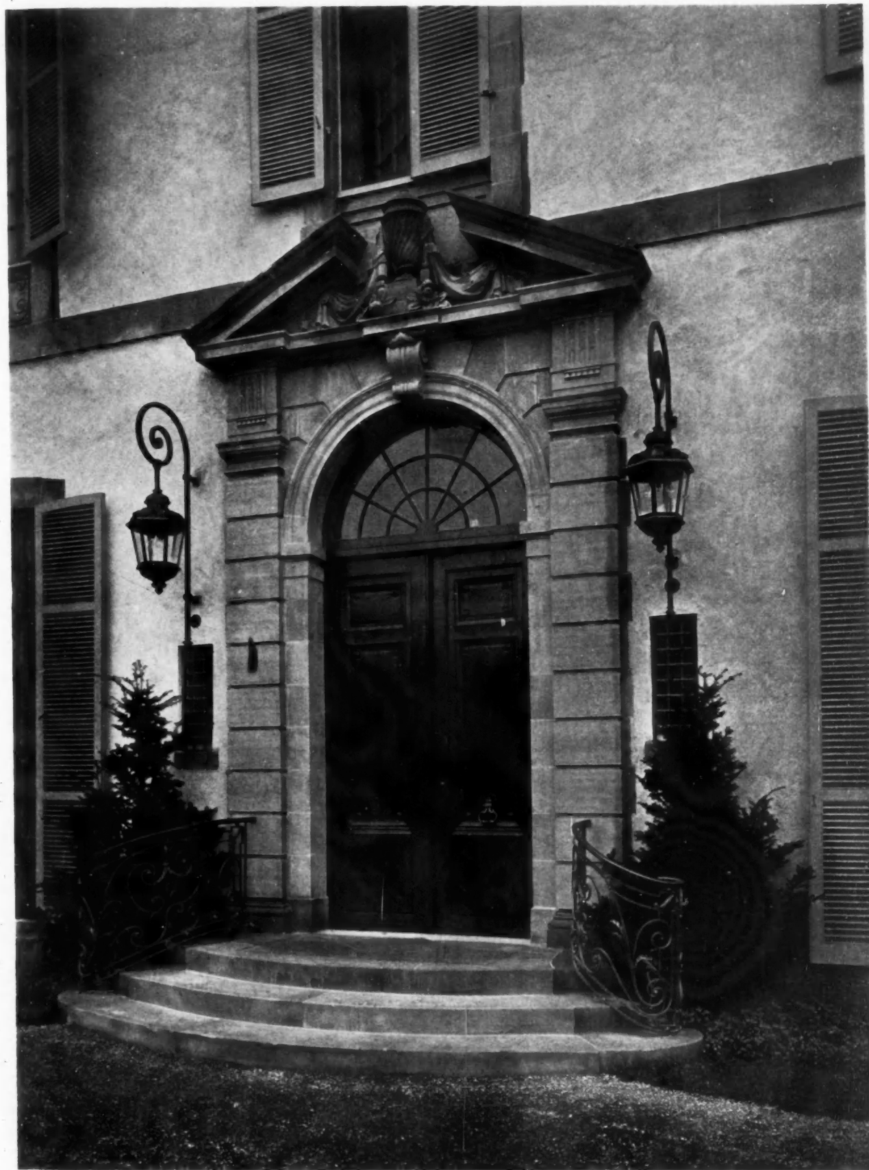
MAIN ENTRANCE, HOUSE OF MOSES TAYLOR, ESQ., PORTSMOUTH, R. I. JOHN RUSSELL POPE, ARCHITECT
