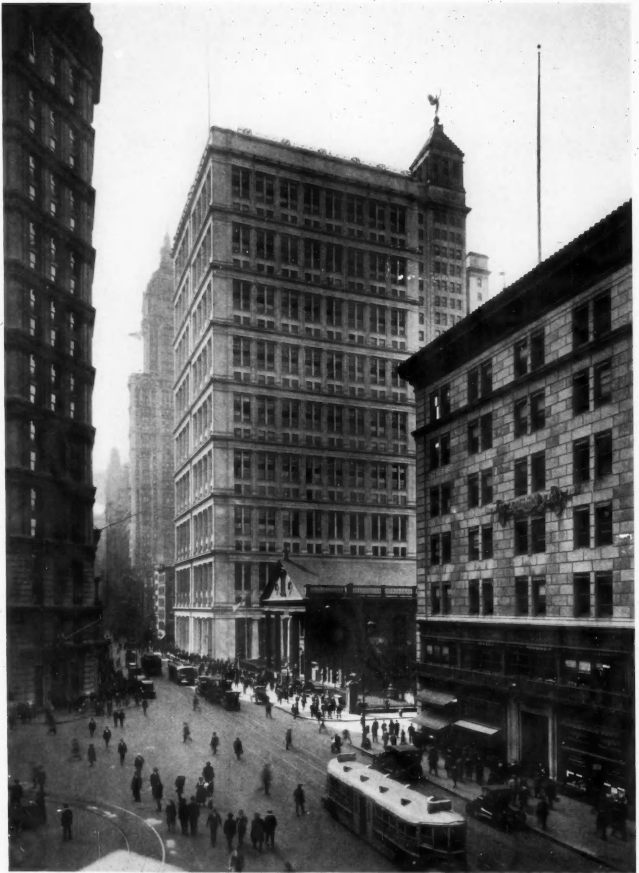
AMERICAN TELEPHONE & TELEGRAPH BUILDING, NEW YORK WELLES BOSWORTH, ARCHITECT
