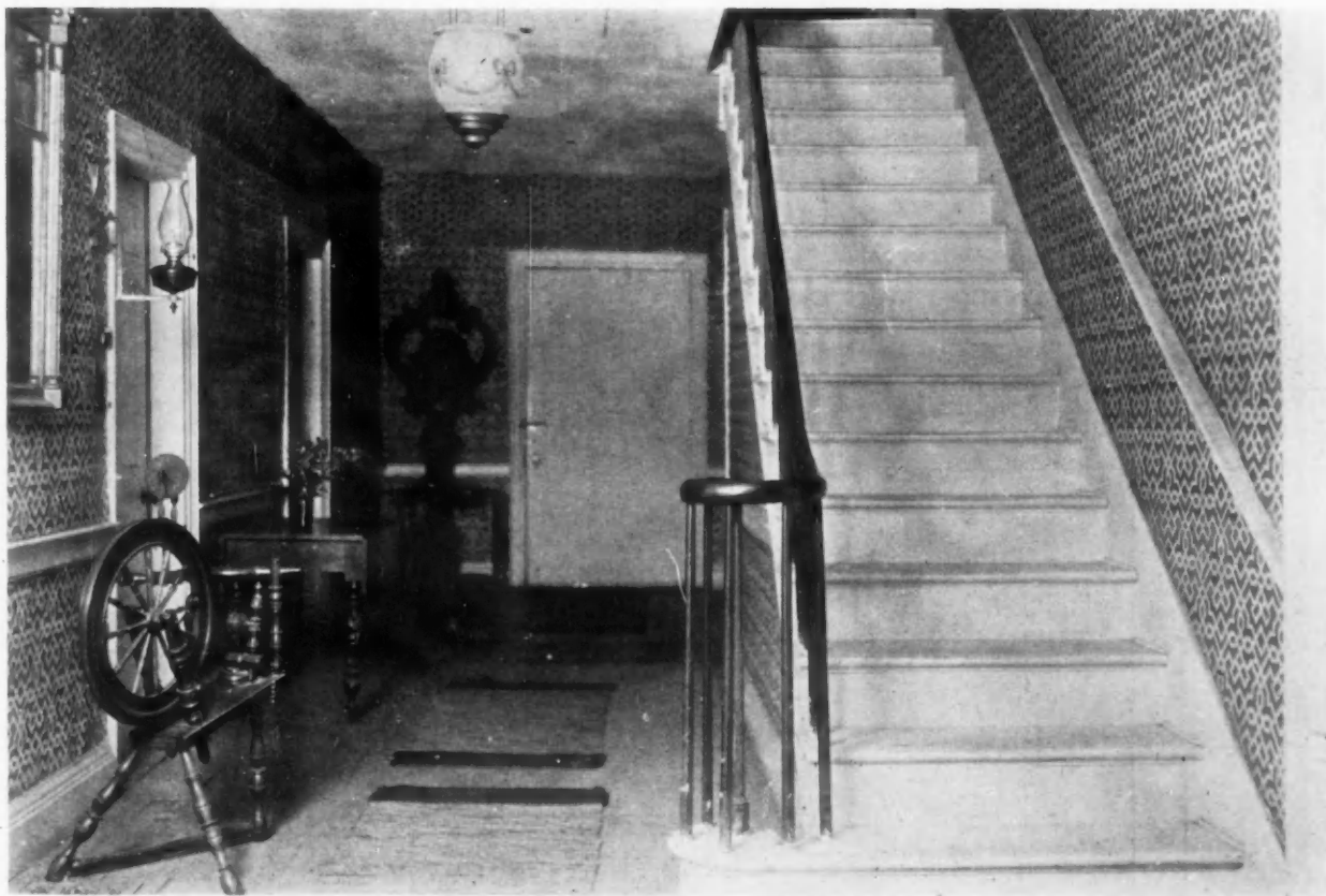
Stair Hall, Taintor Homestead
