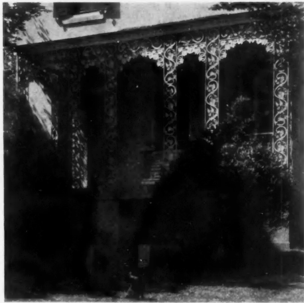
Veranda of Service Wing
