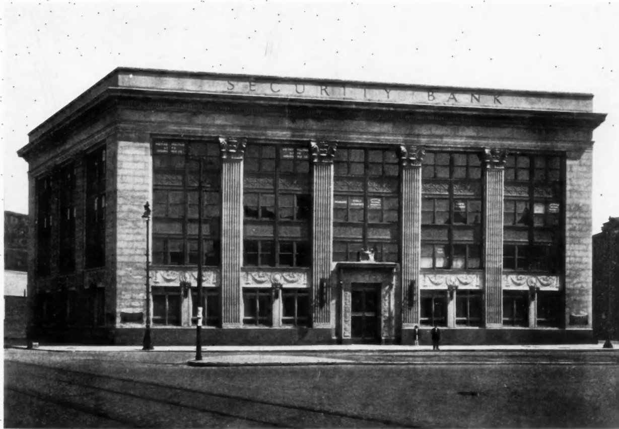
Security Bank of Chicago Childs & Smith, Architects
