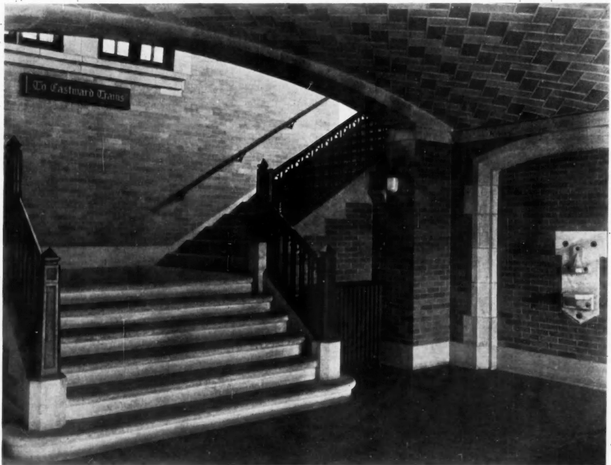
Lobby, Madison Station
