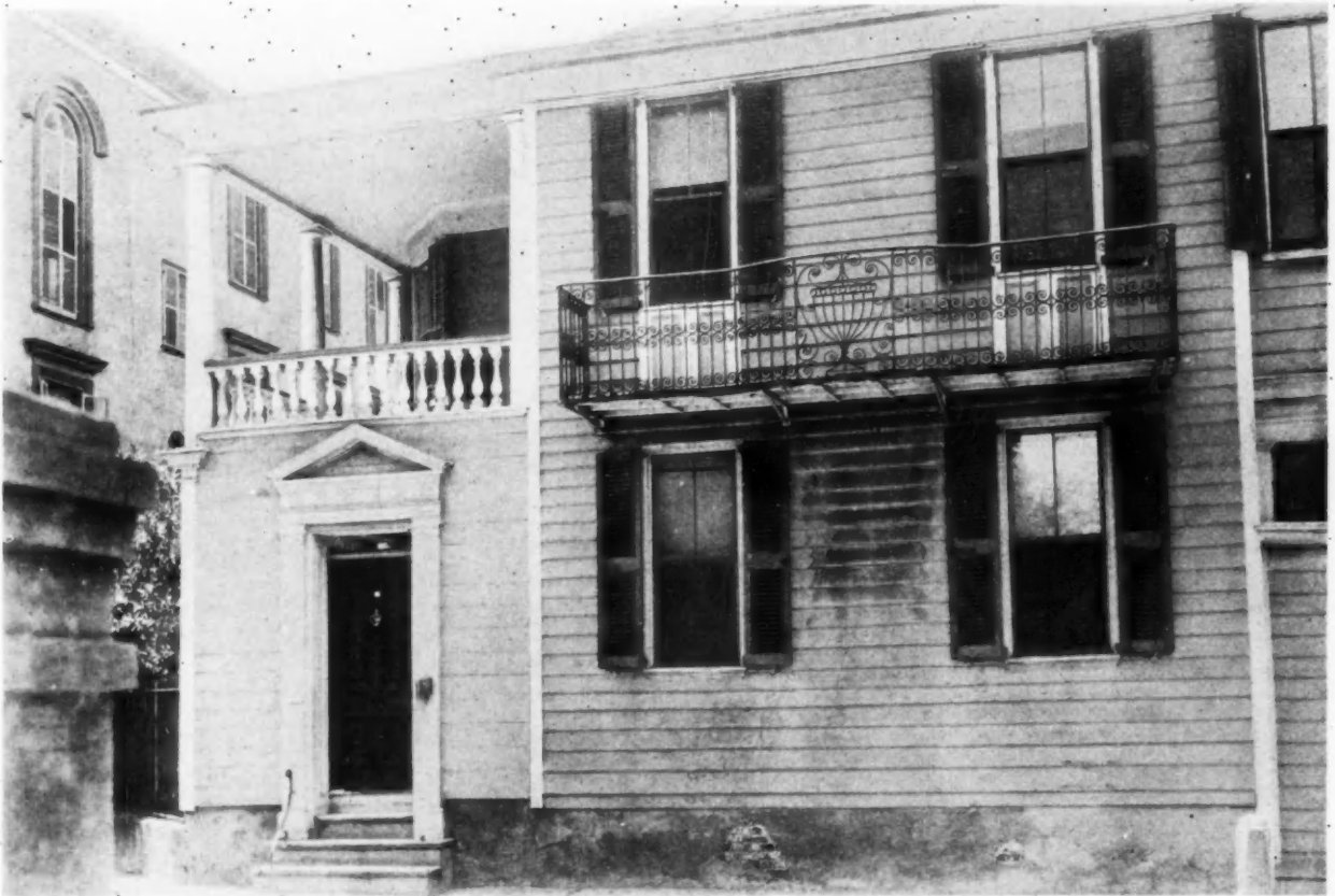
RESET WROUGHT IRON BALCONY; KING STREET, CHARLESTON
