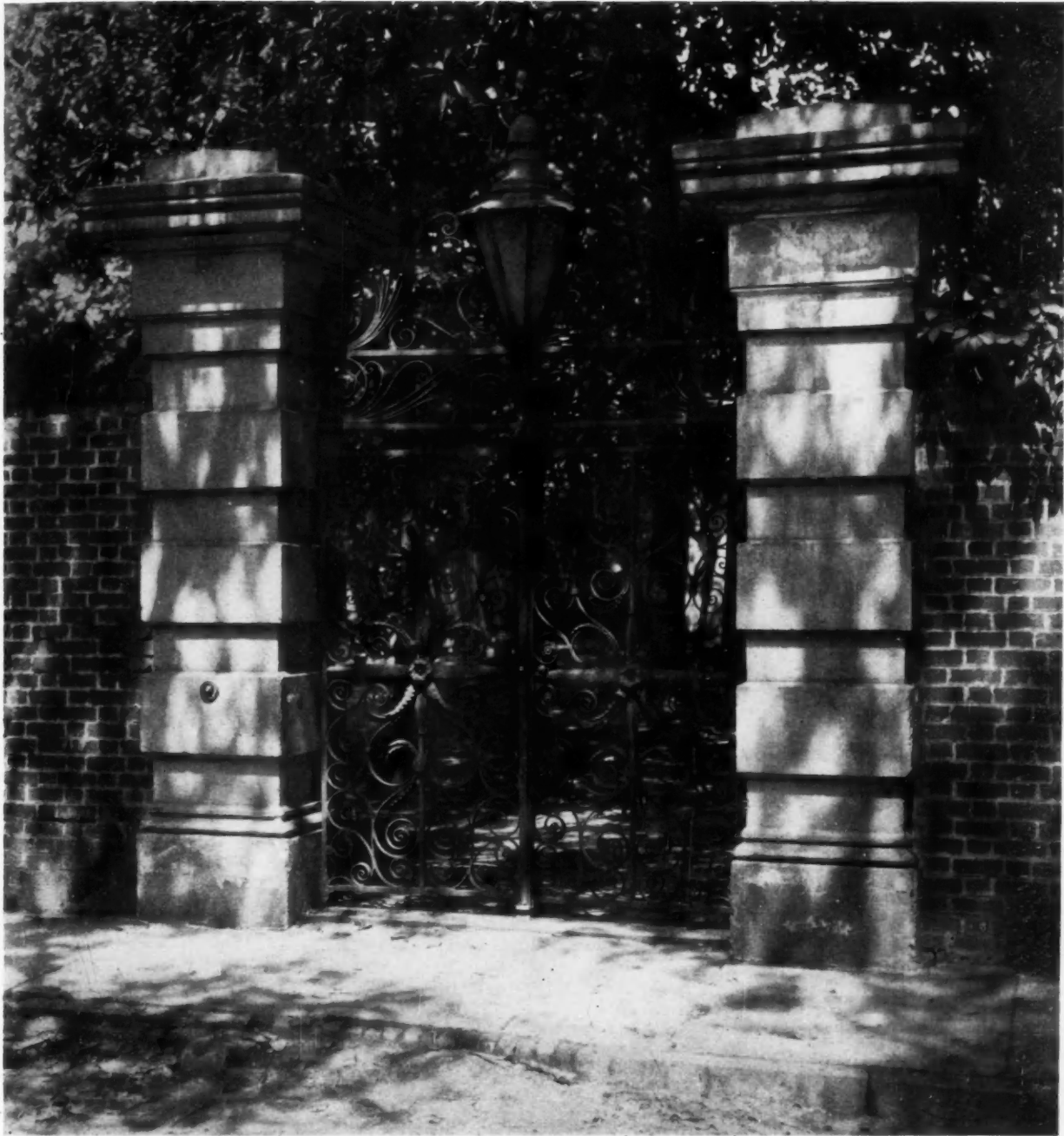
Wrought Iron Gates, Simonton Residence, Charleston. Attributed to Werner and Dothage
