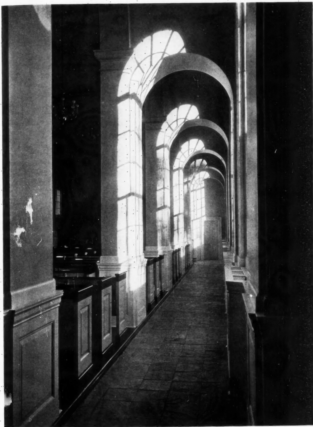
SIDE AISLE; THE VILLAGE CHAPEL, PINEHURST, N. C. HOBART B. UPJOHN, ARCHITECT
