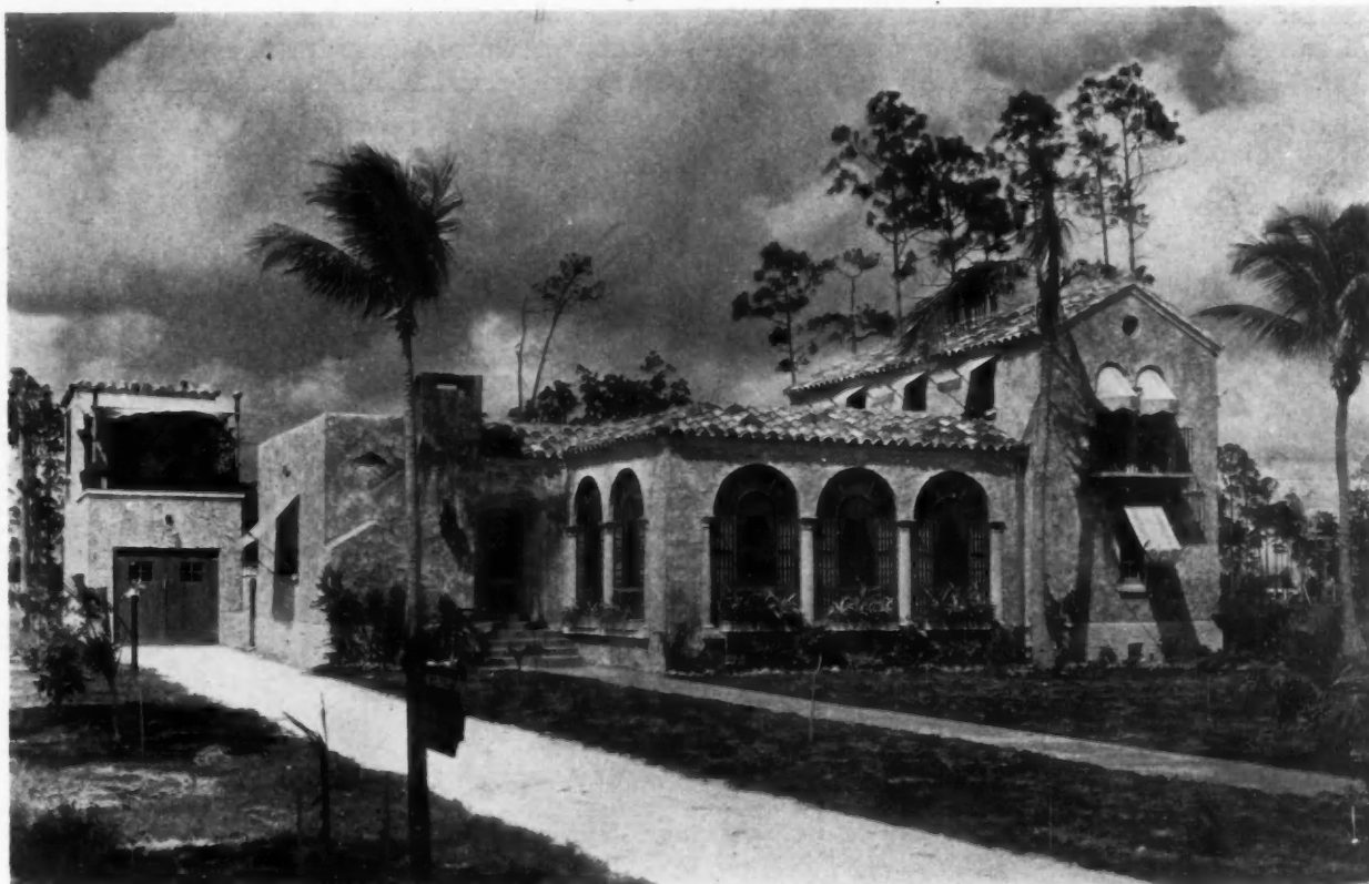
A Building Typical of What Has Come to Be Known as the "Mediterranean Style," Coral Gables
