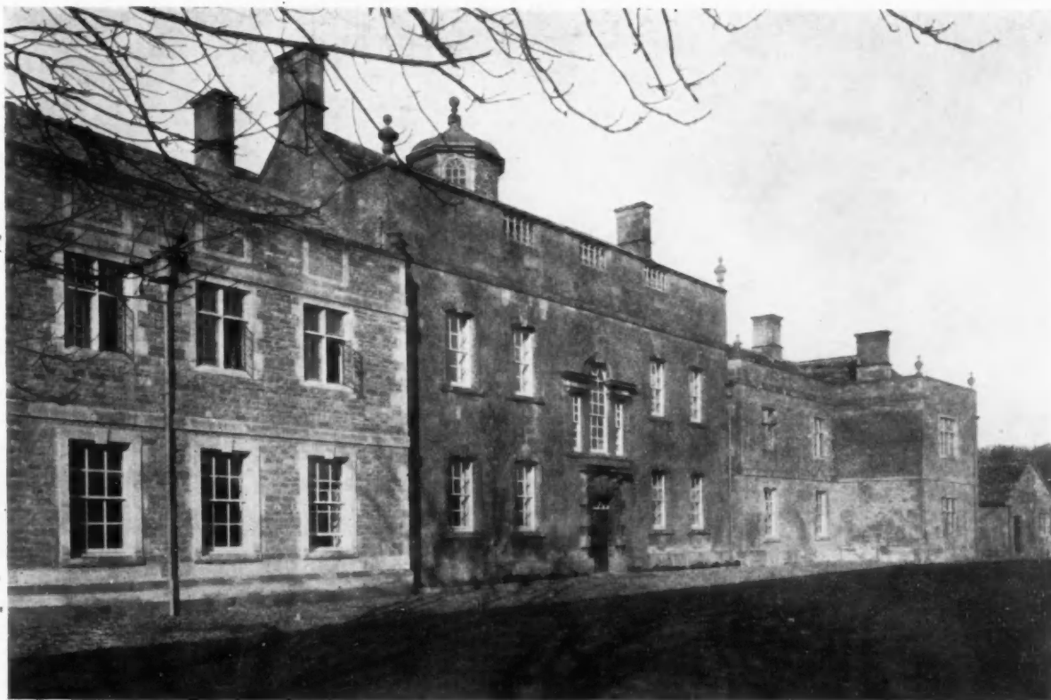
The Garden Facade of Harington House
