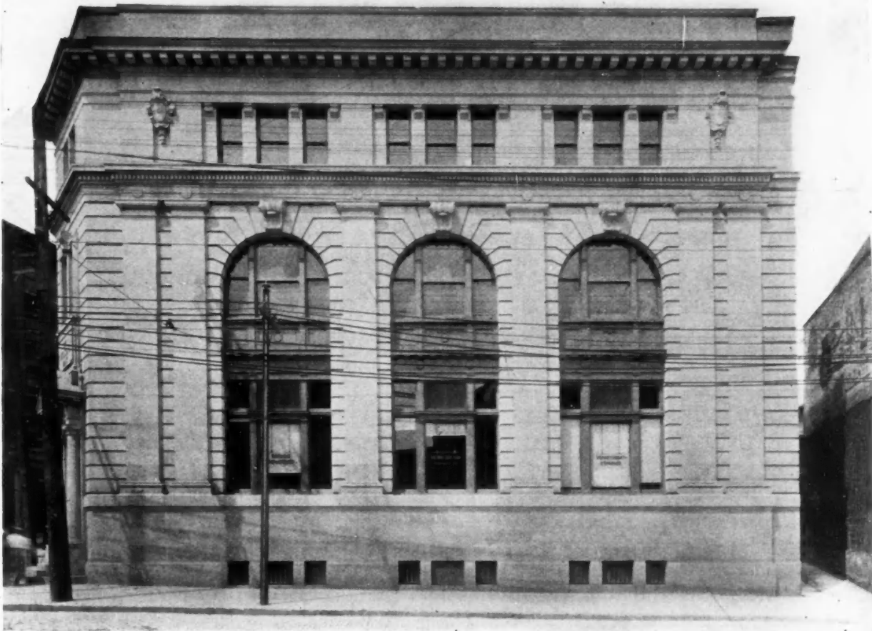
BRANCH OF THE BANK OF MONTREAL, MONTREAL PHILIP J. TURNER, ARCHITECT
