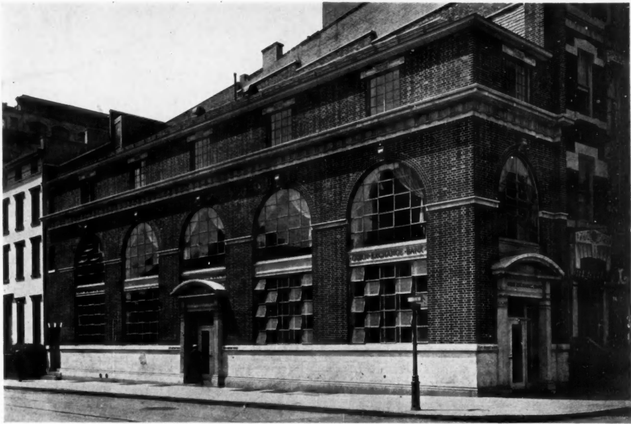
SHERIDAN SQUARE BRANCH, CORN EXCHANGE BANK, NEW YORK S. EDSON GAGE, ARCHITECT
