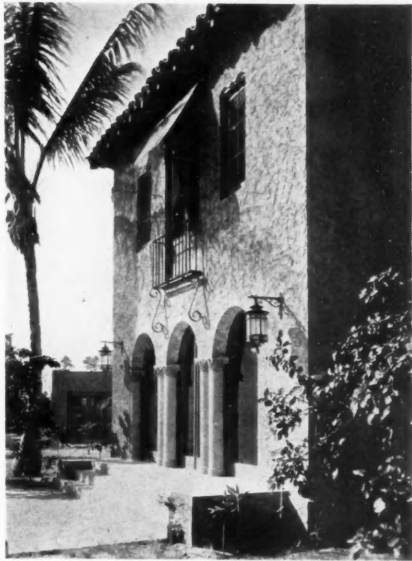
Details of an Entrance Facade, Coral Gables, Fla. An excellent use of textured stucco
