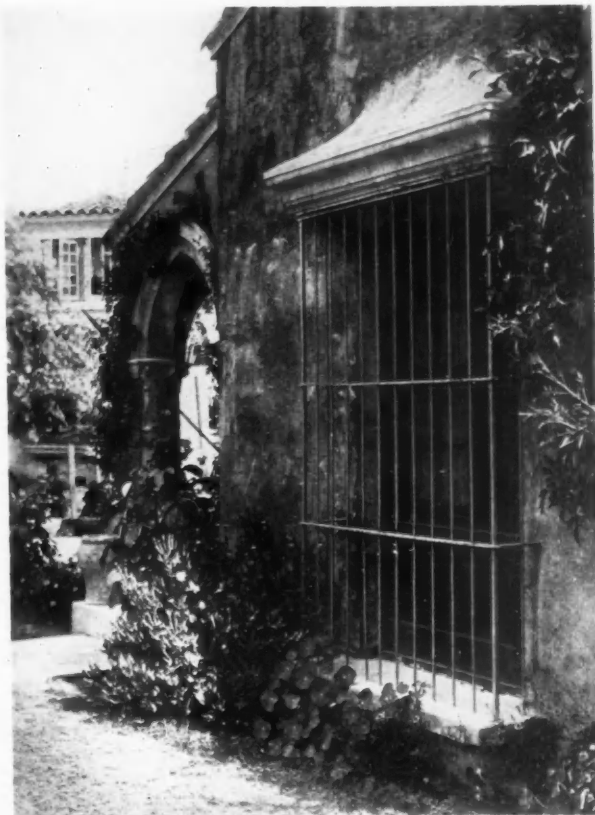
Window with Grille in Spanish Fashion, Coral Gables An excellent use of simple ironwork
