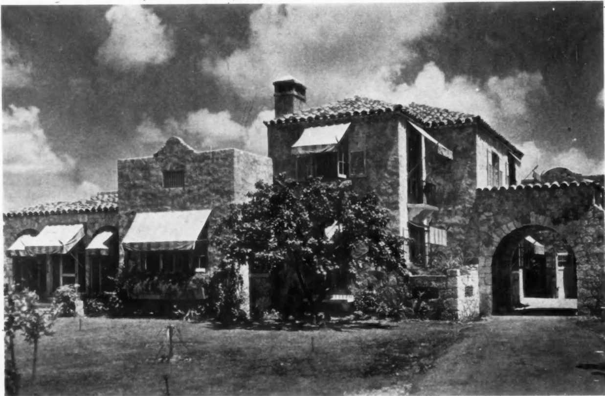
A Typical House at Coral Gables; Built of Stuccoed Tile and Coral Rock
