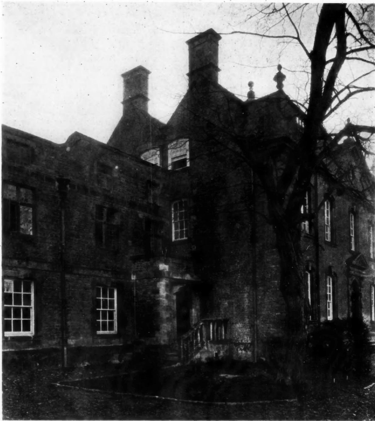
Entrance to Service Wing, Harington House
