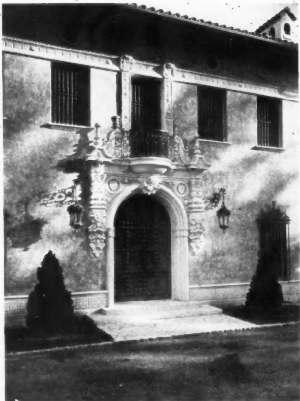
Detail of Entrance, "El Jardin," Coconut Grove, Fla. An adaptation of Plateresque ornament
