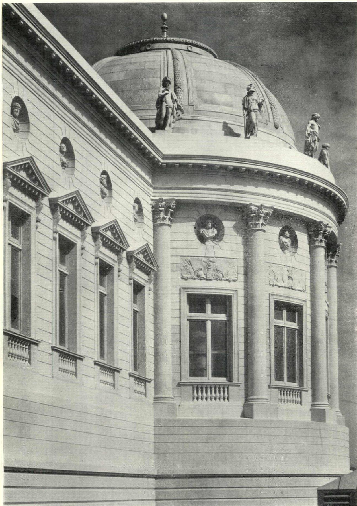
DETAIL, SEMI-CIRCULAR BAY WITH DOME CALIFORNIA PALACE OF THE LEGION OF HONOR, SAN FRANCISCO GEORGE A. APPLGARTH, ARCHITECT
