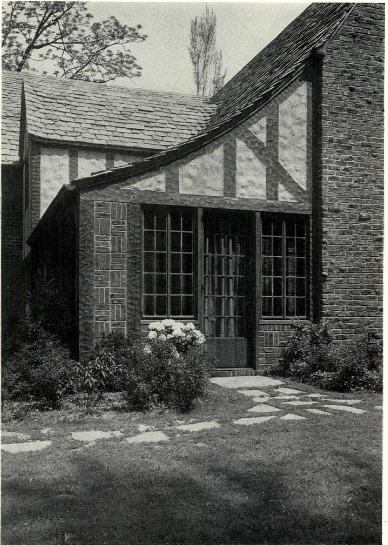
DETAIL, ENTRANCE TO SUN PORCH HOUSE OF J. W. DAY, ESQ., DOUGLASTON, N. Y. FRANK J. FORSTER, ARCHITECT
