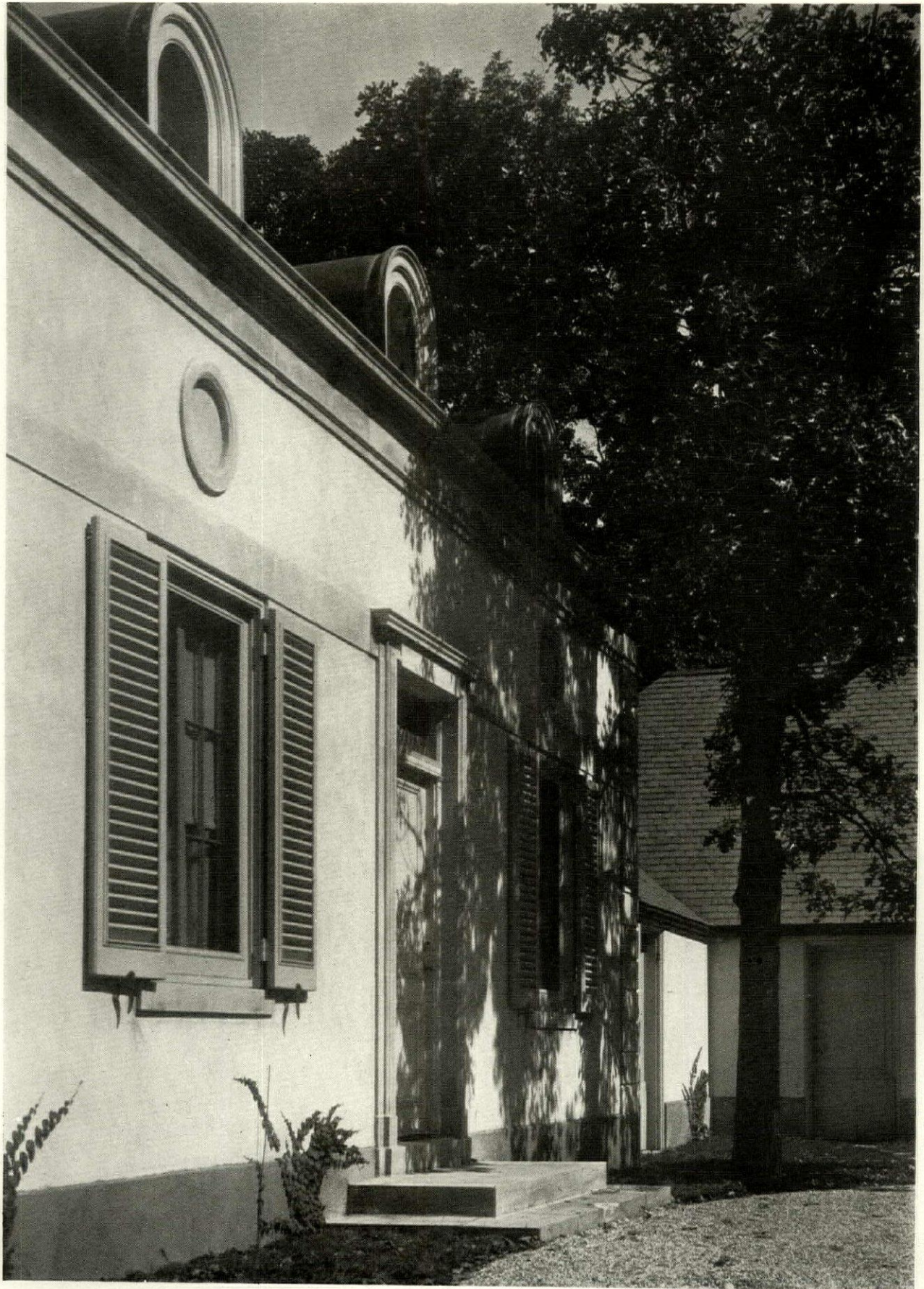
DETAIL, SERVANTS' QUARTERS, HOUSE OF CHARLES FORMAN, ESQ., WINNETKA, ILL. EDMUND B. GILCHRIST, ARCHITECT
