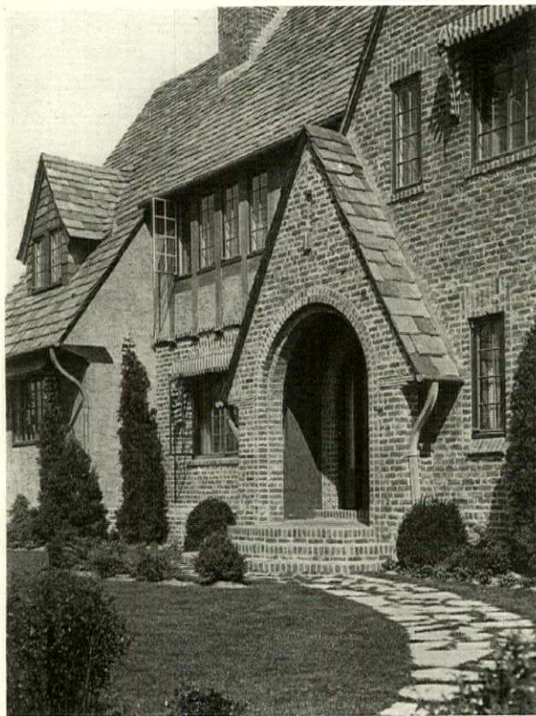
Detail of Entrance
