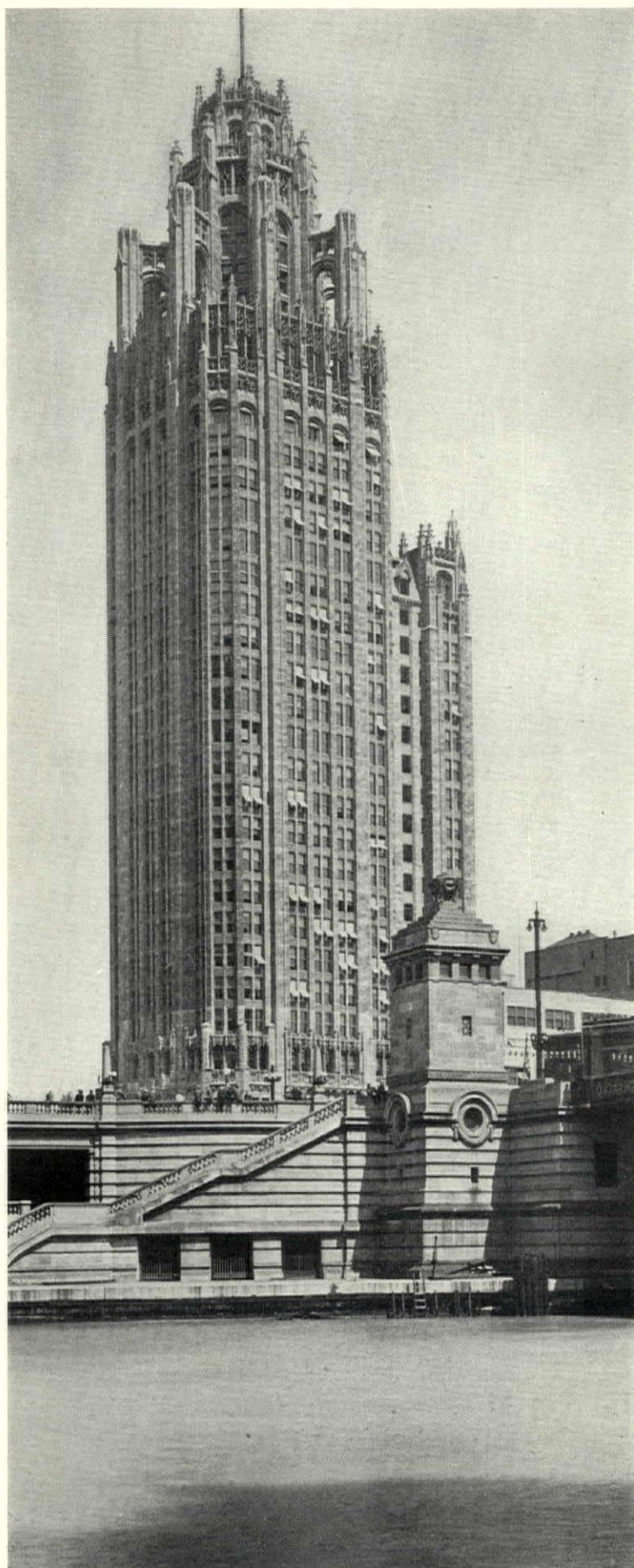
The Tower Rises Majestically Above the Chicago River
