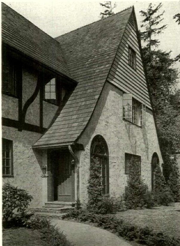
Detail of Entrance
