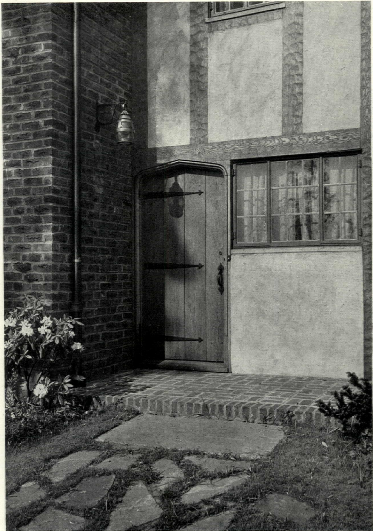
DETAIL, ENTRANCE DOOR HOUSE OF J. W. DAY, ESQ., DOUGLASTON, N. Y. FRANK J. FORSTER, ARCHITECT
