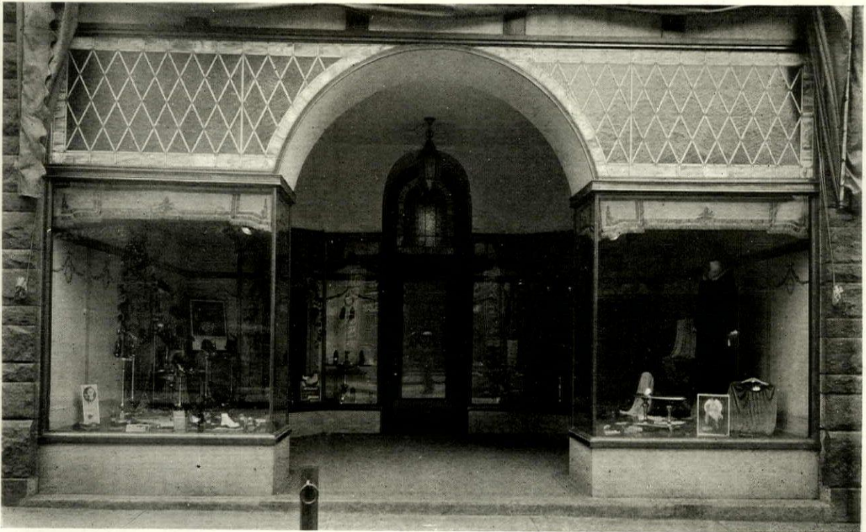
The Morrison Shop, Pittsburgh; Another Example of the Arcaded Type of Shop Front, Which Invites Passers-by to Step in from the Street and Examine Merchandise at Leisure
