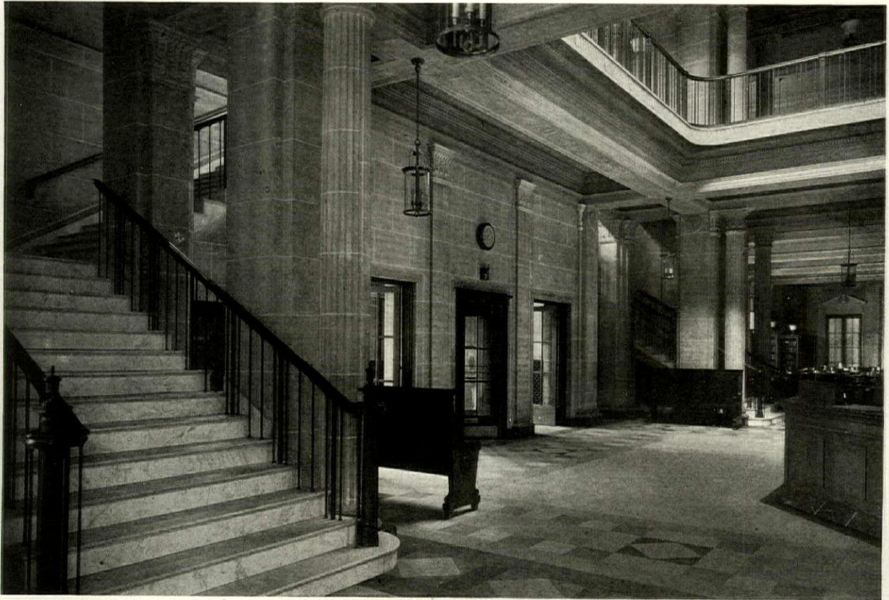
LOBBY, STAIRS AND ENTRANCE DOORS
