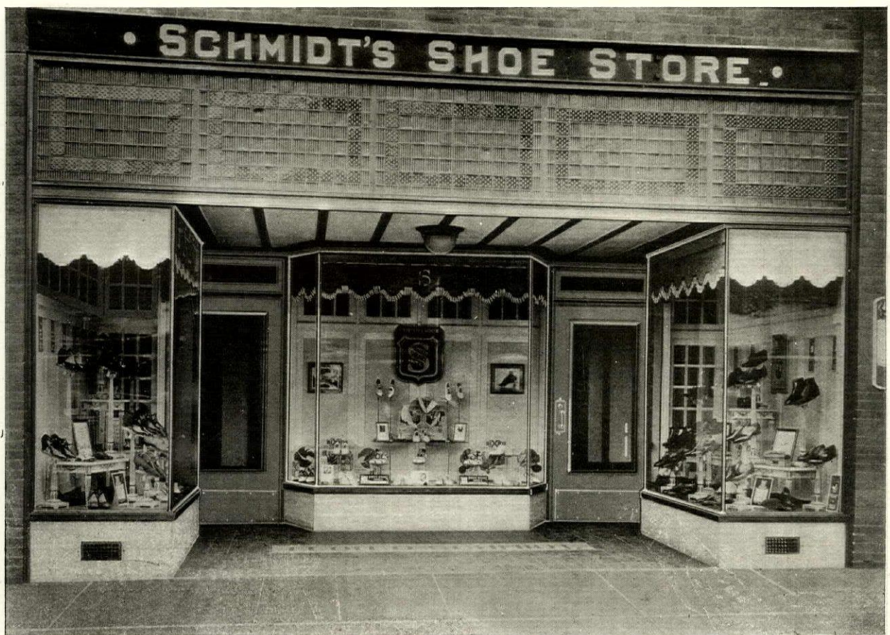
A Treatment Where Two Entrances Are Required
