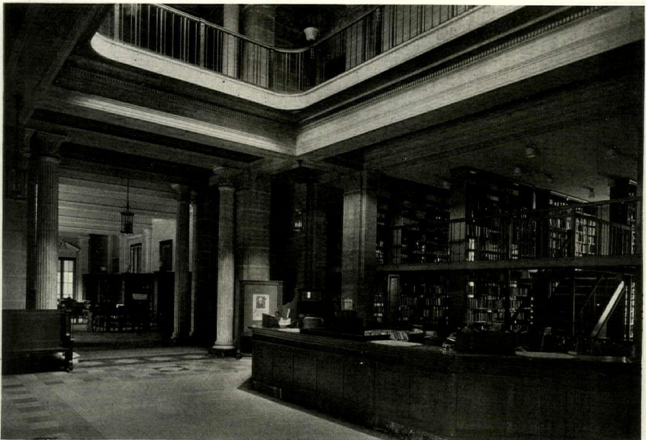
DISTRIBUTION DESK IN LOBBY
