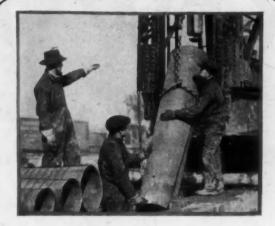
—that's one section of a spirally reinforced steel shell for a Raymond Concrete Pile—every Raymond Concrete Pile is poured into a spirally reinforced tapered steel shell and the shell is left in the ground.
