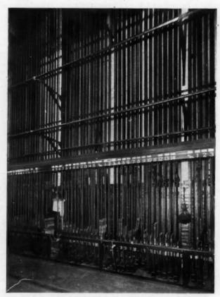
Typical Installation of a Counterweight System
