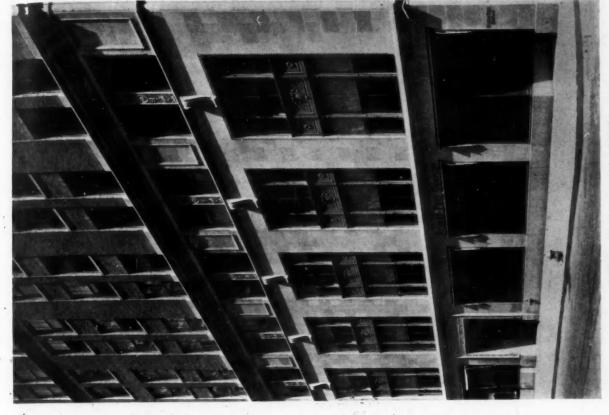
Con-Of the Westinghouse struction: steel frame; furnished from Building the walls are limestone and brick; cast reinforced concrete floors. Heat and elec-GROUND FLOOR PLAN public service stations. iron decorations. tricity
