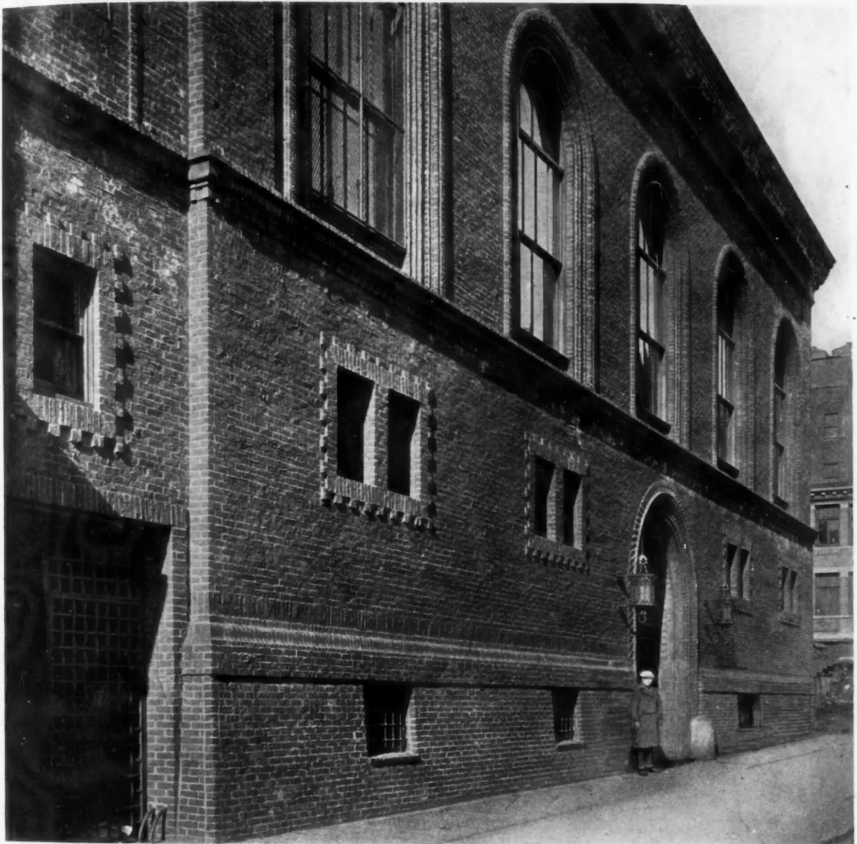
MAIN FRONT ON SECOND STREET
