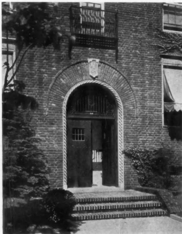
Entrance Doors, "Linden Court," Show Fine Detail
