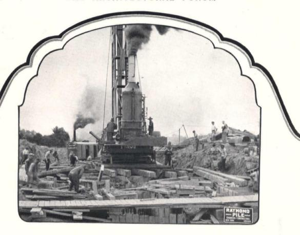
The one thing you must be certain of in a concrete pile foundation is that every pile is perfect . . . hence the importance of remembering that every Raymond Concrete Pile is protected by a spirally reinforced steel shell—and the shell is left in place in the ground.
