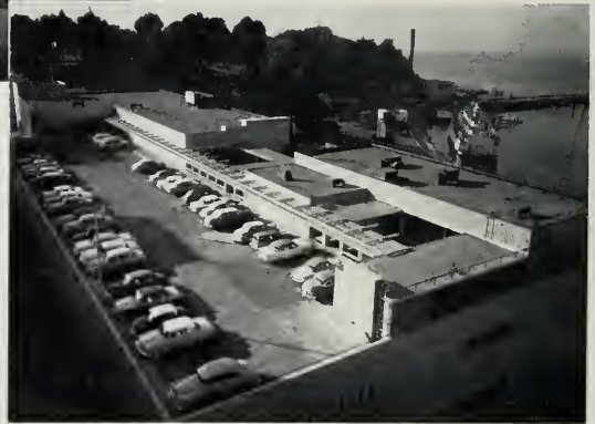
Roof Parking Area, Cafeteria, and Assembly Hall
