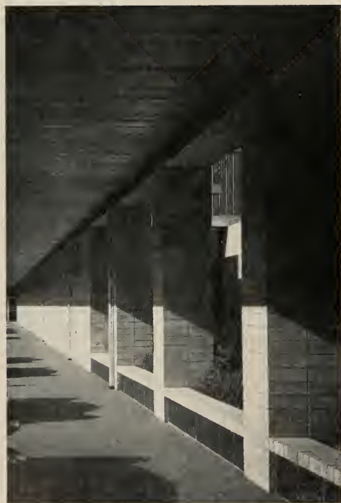
Detail—Covered Walkway to Third Floor Entrance, Eastman Kodak Building Kitchen & Hunt, Architects
