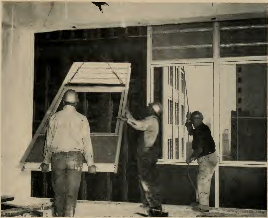
Maximum flexibility for expansion and contraction during thermal changes is made possible by split mullians. Note the studs far fastening into angle clips in upper left of frame.
