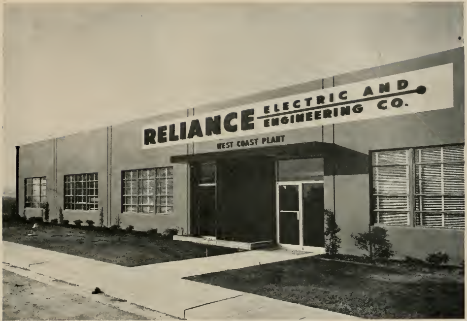
RELIANCE ELECTRIC & ENGINEERING COMPANY'S new West Coast assembly plant and distribution center . . . the 40,000 square foot plant was one of the first to be constructed in the Millsdale Industrial Park where Associated Construction and Engineering Company has been one of the most active builders. George Jennings, Engineer.
