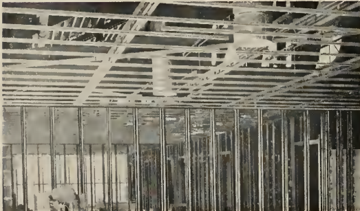
LIGHTSTEEL was used for all interior partitions and ceilings in the office area.
