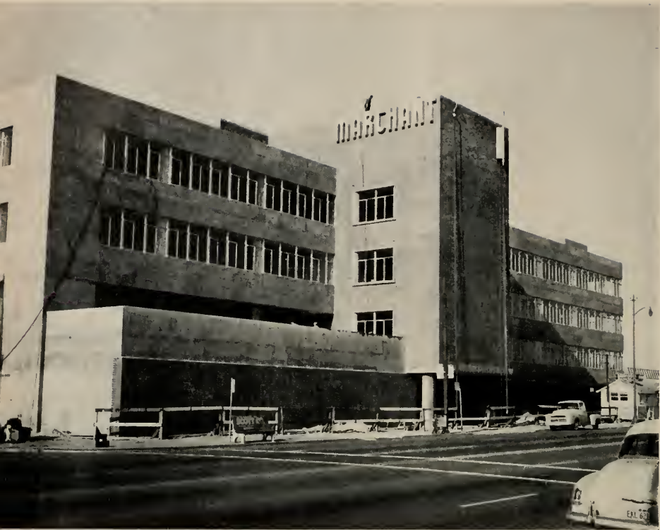
NEW PLANT NEARING COMPLETION
