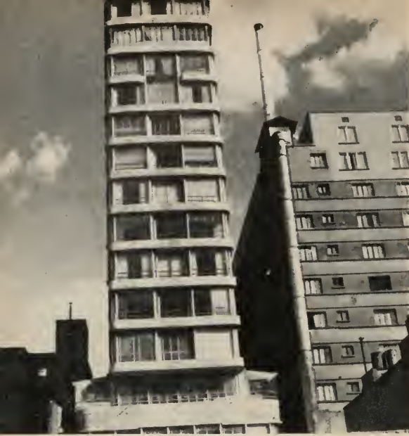
13-STORY concrete structure near Reforma Hotel—note slenderness of building. No damage observed.
