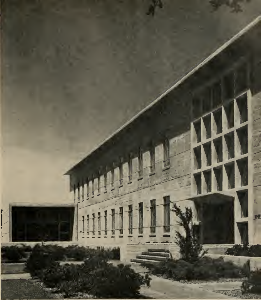
WM. CLEMENT AMBROSE, Architect, Fellow, A.I.A. (Wm. Clement Ambrose and Eldridge T. Spencer, Architects)
