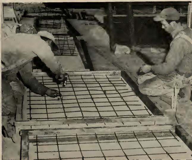
Forming Tilt-up wall panels
