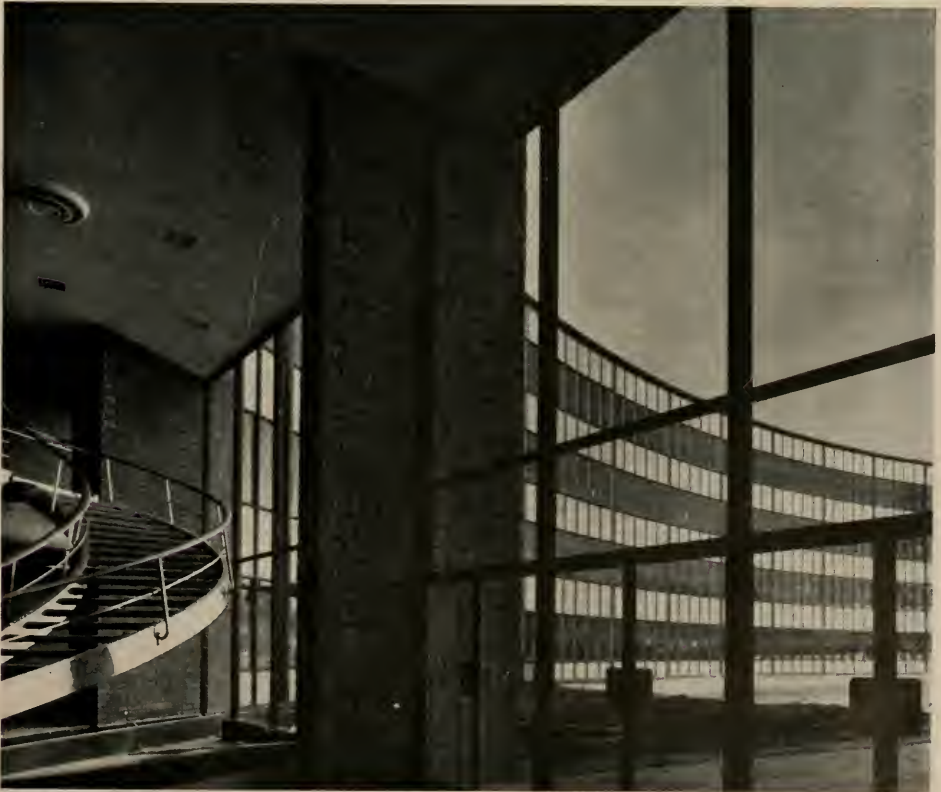
BUILDING'S principal entrance . . . attractive and inviting.
