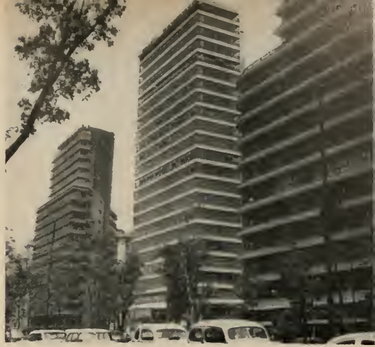
20-STORY Reforma No. 69 building on left settled four inches and suffered slight exterior damage. Center is 25-story Reforma No. 51, steel frame structure, no damage observed. American Embassy, at right, suffered considerable 15th and 16th floor damage.
