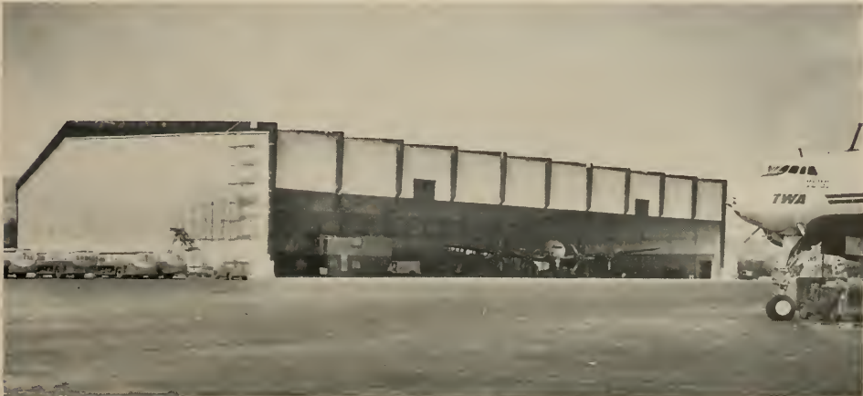
PORTION OF NEW HANGAR nearing completion.
