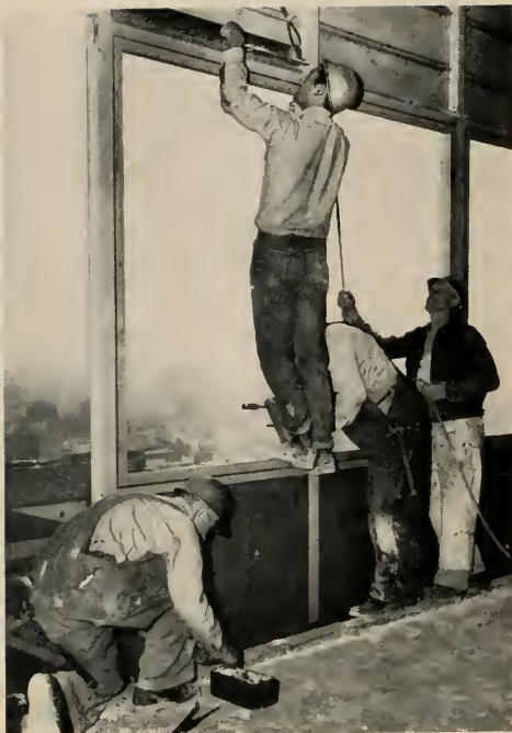
Inside Setting: No scaffolding. Note interior back-up.
