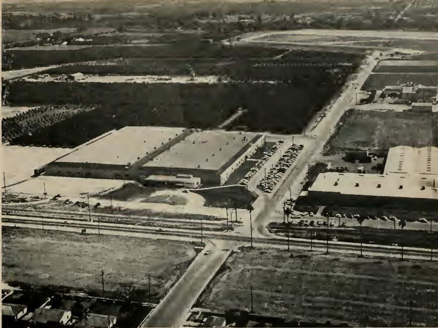
NEW MARATHON PAPER COMPANY plant at Modesto, California. Built by Associated Construction and Engineering Company. Simpson & Stratta, Engineers.
