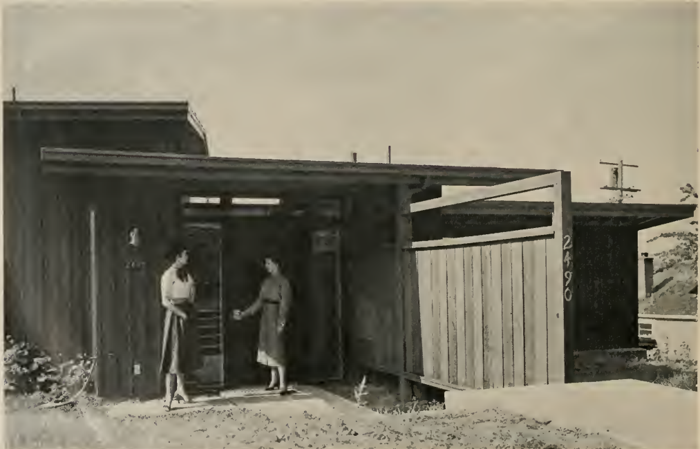
ROOF OVERHANG in combination with focussing solid cedar screen calls attention to this charming entrance door framed in glass.
