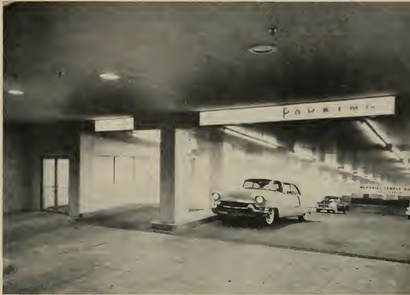
MAIN RAMP of the Garage on California Street extends down several floors and has a capacity of 500 cars.
