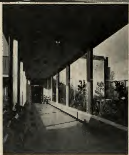
GLAZED PASSAGE WAY from cafeteria to general offices through the attractive roof garden.
