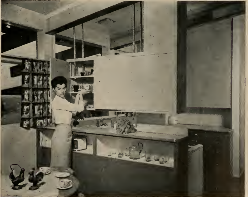
L-SHAPED SUSPENDED CABINET and storage peninsula separate kitchen and breakfast room in the Eugene, Oregon, home.
