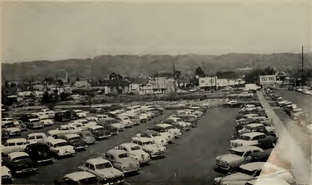
SITE . . . as it appeared prior to start of new construction, partially used as parking area. Berkeley hills in background.
