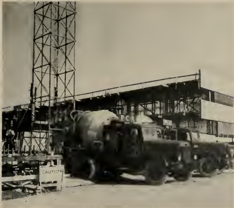
READY-MIX concrete trucks supply more than 35,000 cubic yards of concrete.
