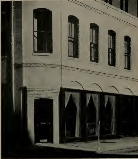
Wurster, Bernardi & Emmons, A.I.A. Architects, remodeled above. View shows "The Days," furniture, first showroom of Jackson Square to open.
