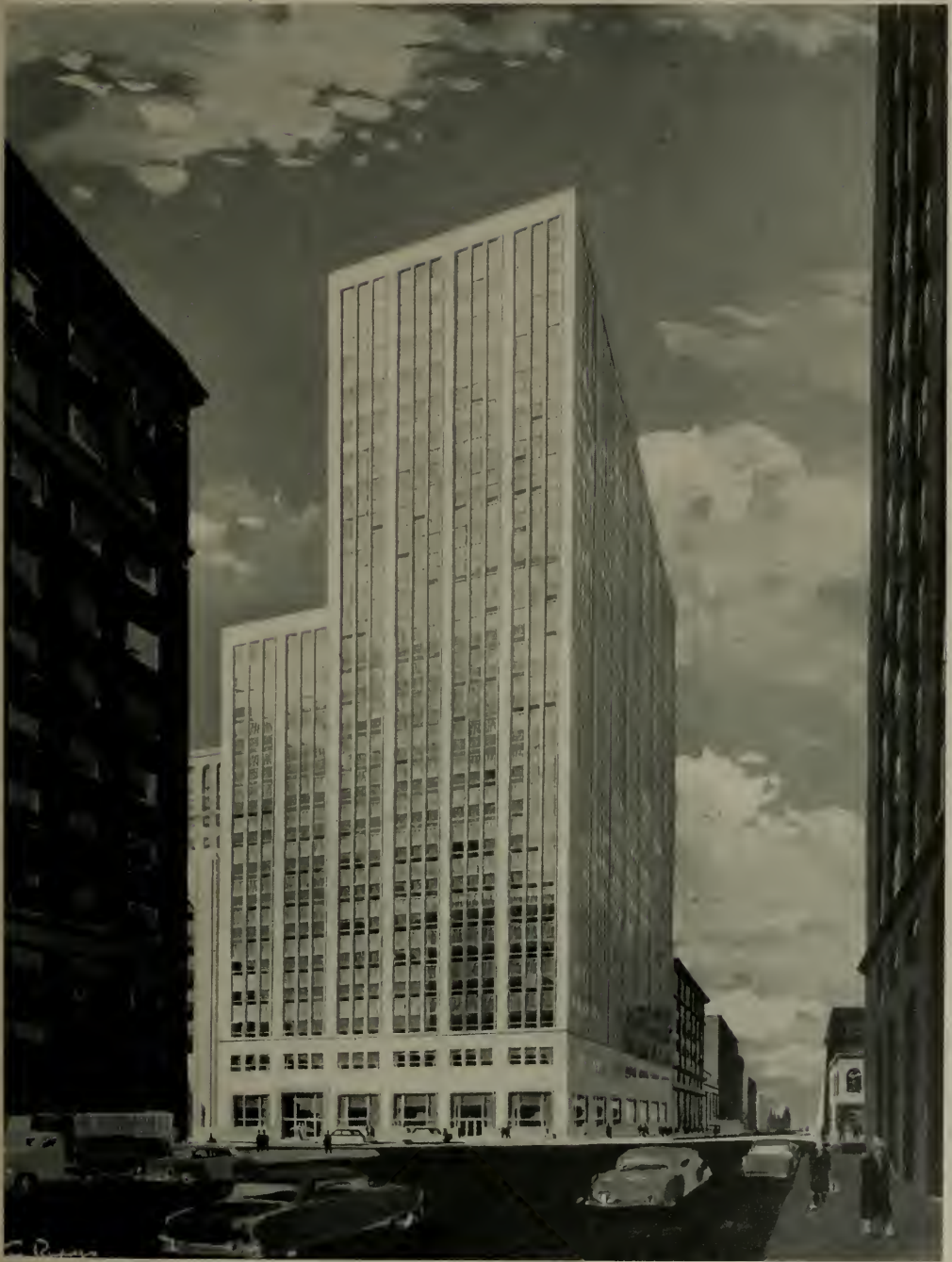
EQUITABLE LIFE ASSURANCE SOCIETY BUILDING, San Francisco
