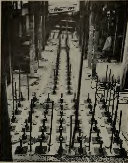
View of entire pylon at Third Floor level at completion of tensioning of Stressteel bars.
