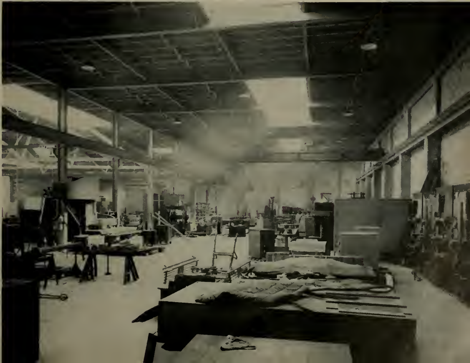
Lower view shows Main Factory facilities for heavy vault construction.
