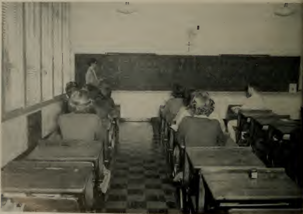
INTERIOR VIEW—Typical High School installation including ION-controlled automatic electric heating equipment.
