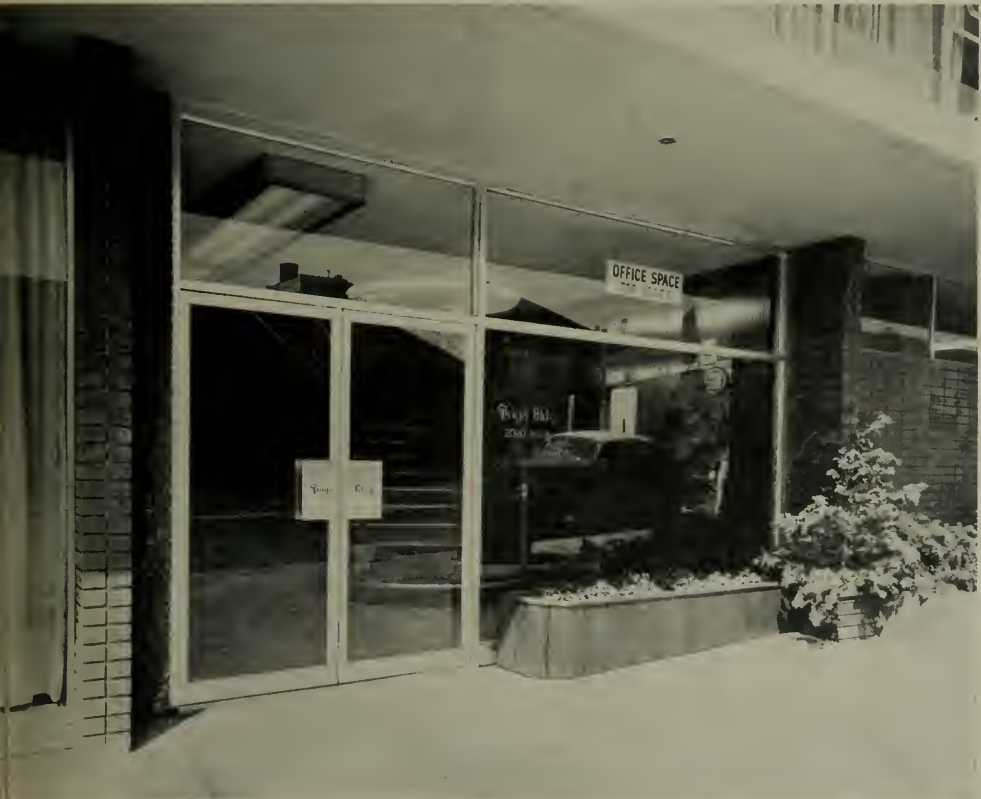
ENTRANCE to the attractive building, showing modern hollow hulor doors with identification push plates.
