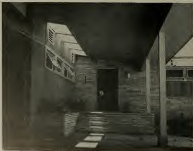
Flagstone steps lead from carport to main entrance door, protected by roof overhang. For privacy from road, windows are high.
