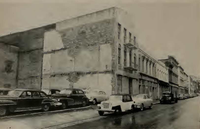
PARKING LOT and building, viewed above, as they looked in 1952 when purchased by the Jackson Square Land Company.
