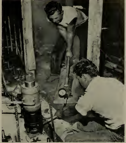
Tensioning crew in action. Note method of taking up elongation of bar with pin wrench. Split washer or shims at hand to slip into place when proper elongation is obtained.
