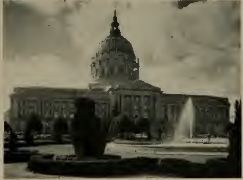
REBUILT —Stands among nation's outstanding civic buildings. (Bakewell & Brown, Architects.)
