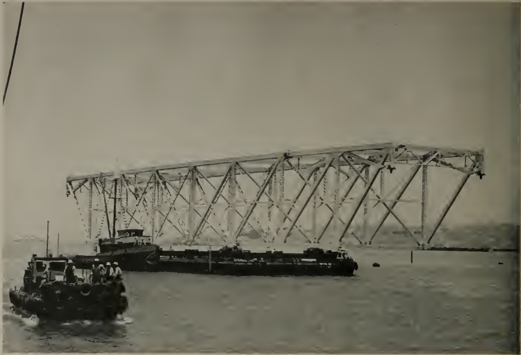
Fig. 1—Aluminum Falsework Truss Being Towed Into Position.
