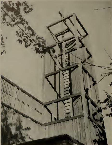
CENTRAL LUTHERAN CHURCH, Portland. Belluschi and Skidmore, Owings & Merrill, Architects. (Above)
