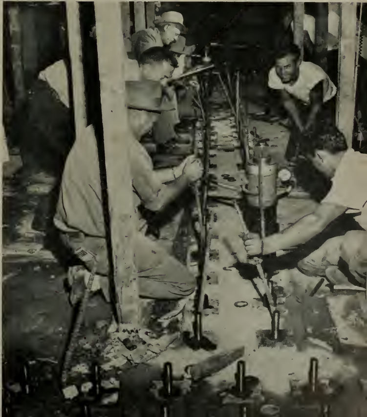
Tensioning crew in action. Note method of taking up elongation of bar with pin wrench. Split washer or shims at hand to slip into place when proper elongation is obtained.
