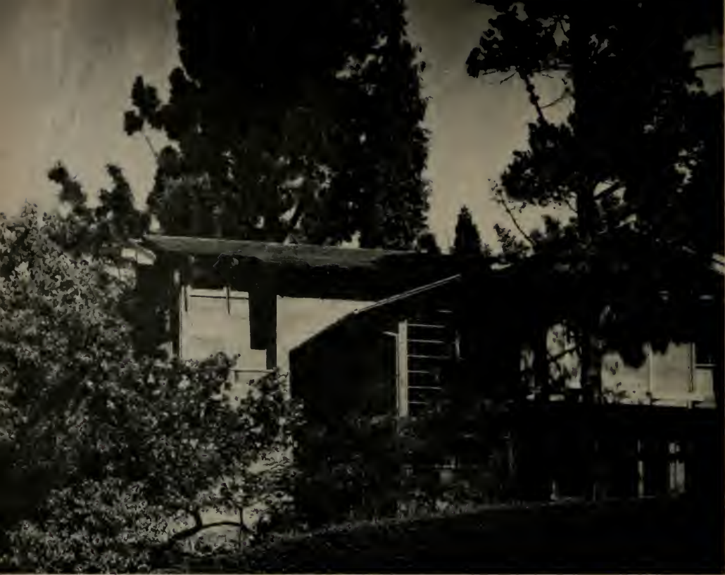
EXTERIOR VIEW OF THE KITCHEN WING . . . Apartment below.
