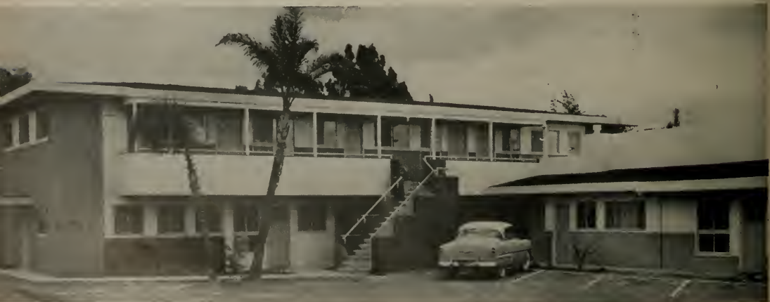
CLOSE-UP view of two story portion of the Grossmont Professional Building, indicating type of architecture and construction.
