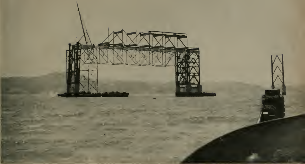
Fig. 4—Position of Permanent Steel Truss Being Erected Upon Aluminum Falsework Truss.
