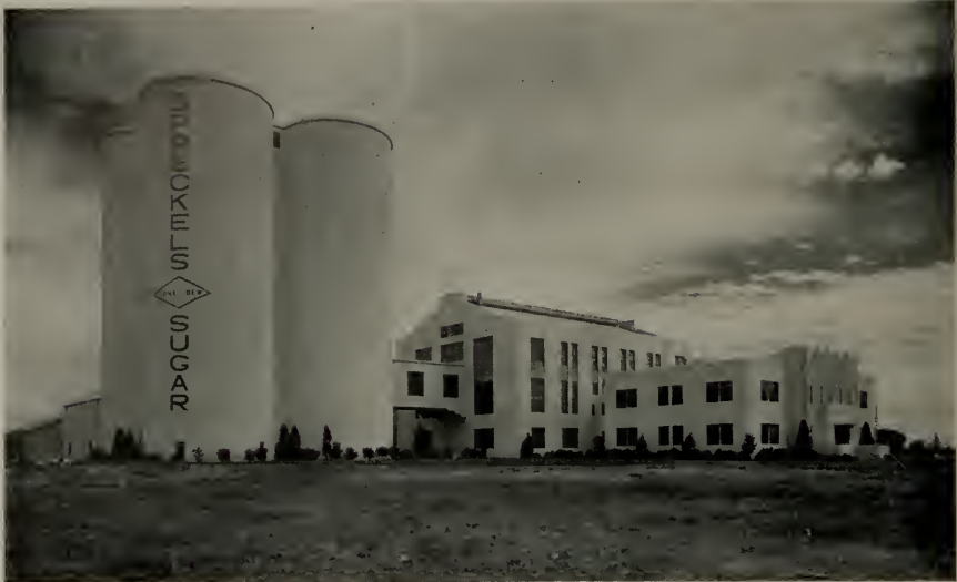
SPRECKELS SUGAR COMPANY plant at Woodland, California
