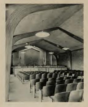
designed the Compton-Imperial Housing Project Auditorium. He says: "Wood laminated trusses were used on the project to meet the general design problem of clear span requirements as well as pleasing form. In addition, the wood trusses offered the necessary firerating and a more economical solution."
