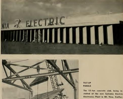
stalled at the new Sylvania Electric Electronics Plant in Mt. View, California, is picked up by large crane and snaked out bockwards between roof supports; is then "tilted-up" into proper position.
