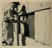
**3** To insure permanent bond between Veneer and structure, the wall surface is also brushcoated with the same Portland cement mixture.
