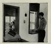
The conveyor consists of a vertically moving chain bearing finger type carriers; adjusted to unload at each receiving station and marked accordingly by a number of distinctive color. May be arranged for loading or unloading at any number of floors. Loading is done manually directly into the carriers on the "up" side of the carriers, unloading is completely automatic on the "down" side. Unistrand Conveyors are designed and
