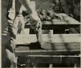
**2** Immediately before setting, the back of the Ceramic Veneer unit should receive a brush coat of neat Portland cement and water.
