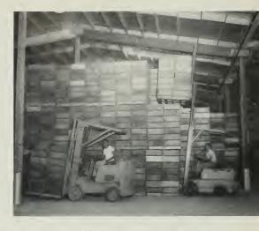
WAREHOUSE IN OPERATION—Designed to store cased canned goods; Shows fork lift trucks stacking green pears which will ripen in the enclosure . . . an ideal method of ripening since the variance of day and night temperature is small due to the thermal qualities of the aluminum roof and siding.
