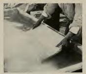
1 Ceramic Veneer units must be soaked in clean water for one hour before using. Wall surface should also be damp at time of setting.
