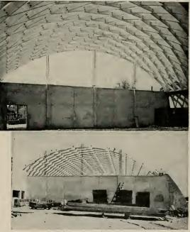
SUMMERBELL Lamella Raaf Construction is easily adapted to till-up wall construction, as illustrated above.
