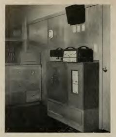
Heart of system is located in Socristy. Automatic roll player sits on counter top to left. In center is bell cabinet; matching cabinet to right contains clock and timer mechanism.
