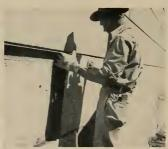
**5** The C.V. unit is then set in place. Excess of mortar will be forced out of joints from the back, leaving a 34 inch mortar bed.
