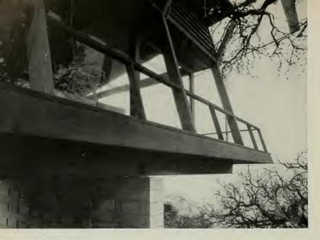
Longitudinal steel girders cantilever well beyond the supporting reinforced concrete block pier to carry floor level out over steeply sloping site.
