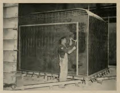
double-brick construction was a commercial practicability. All conduit and piping can be installed and repaired cheaply and quickly, because an air cavity is left between the adjacent walls of any pair of cells.
