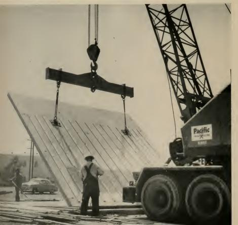
Shown here are the twa tiers of 20 ft. wide precast concrete wall panels that make up the 46 faat high walls.
