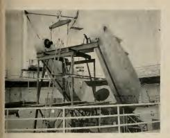
Erection of fork assembly in place supported by the base frame. Scoffolding directly in front of the two fork arms is temporary structure used for erection purposes only. Structure at this point of assembly is approximately S0 feet high.
