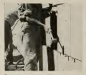
7 He then taps the unit with a rubber mallet to fill all voids, forcing the excess mortar out of joints. Spacers are removed after initial set.
