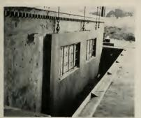
WALL PANEL ready for stripping. Table "tilts" to vertical positions to allow panel to be handled in this position until installed in walls.
