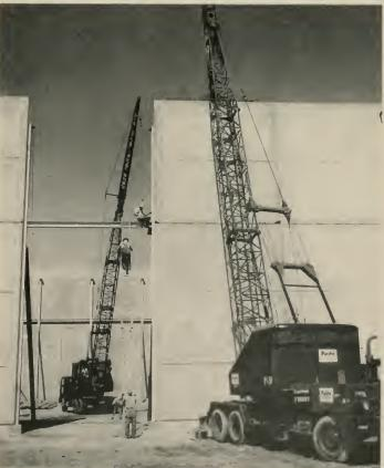
Using up to the minute construction techniques some eighty-four precast concrete wall panels were prepared and installed in a recent four days.
