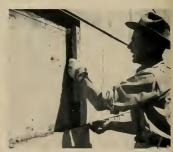
**6** It takes the mason only a few seconds to position the C.V. unit and check it with a level. This insures a true wall plane.
