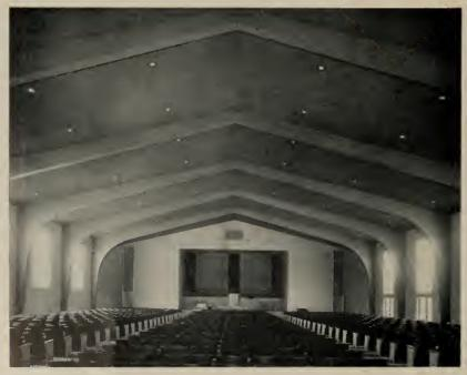
Seattle gives an idea of the decorative value of these man-made wooden arches. The graceful lines of these arches as they sweep majestically from floor to roof is inspiring. The ten curving, boomerang style wooden members provide 90 feet of clear floor area. They have been sanded and finished in natural color to retain the beauty of the Douglas fir texture and grain.
