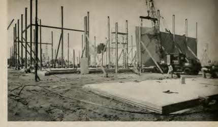
Precast concrete wall panels are poured on special "casting platforms" near their intended erection area—above illustration shows how site loaked at the start of one four-day push.
