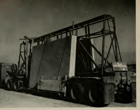
SPECIAL "A" FRAME TRUCKS ARE USED TO TRANSPORT PRECAST PANELS TO JOB SITE. SLABS ARE HANDLED ON THE VERTICAL.
