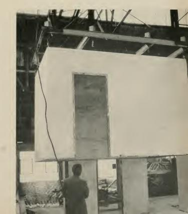
The poured cells are lifted clear of the domed concrete mold, and carried to a section of the foctory for drying preparatory to installation.
