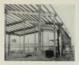
SHOWING erection of prefabricated wall section of United States Products Worehouse in San Jose, California. Walls were raised in 20 ft, sections by fork lift truck.
