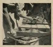
**4** Next, slightly more than 3% of an inch of mortar is applied to the C.V. unit. The same amount is also applied to the wall area.
