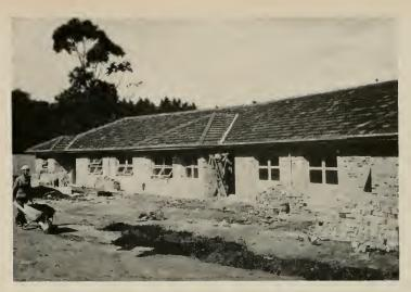
THE CELLS—8'9" by 12'6" and 8'9" by 5', are transported to site and bedded down on standord foundations. Standard brick veneer and marseilles tiles gave this row of units the appearance of a much more expensive construction.
