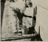
8 Face joints may be raked out and pointed with fine mortar. To complete the job, surface is washed with clean water.
