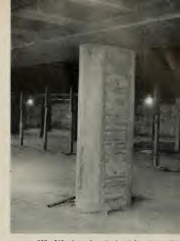
18" x 36" columns from the fourth floor to the fifth floor are smaller to provide wider aisles. NOTE a typicol calumn used elsewhere in the construction is 18" x 54".
