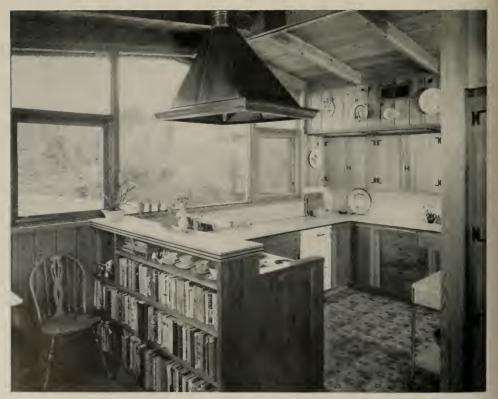
roof insulation which in turn rests on the one-by six fir decking. The decking serves a double purpose as roof boards and ceilings in every room. The slope of roof is pitched gently upward from the west side to extend out over the patio. The lines of the home are highlighted by this "eyeshade" roof extension.
