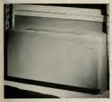
Chilled water is used for cooling; hot water for heating. Each unit is served by only three pipes-water supply and return and drain. Fresh outside air ventilation introduced through aperture in rear of unit; damper controls mixture of fresh and recirculated air.
