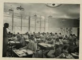
Typical Classroam . . . windows facing hill, acoustical tile ceilings, display boards at rear, movable desks and seat combinations, indirect lighting and asphalt tile floars.
