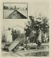
Some 1800 ft. of 9" Macadam base asphalt roadway was cut to a depth of 3%", in accordance with specifications of the city, in a matter of  $12\frac{1}{2}$  hours, or an average of  $2\frac{1}{2}$  ft. per minute.
