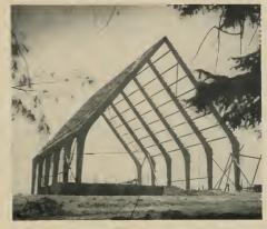
Same idea of the simplicity of erection problems can be had by a laok at this skeletan of laminated arches which pravide all the structural elements at the St. Albert the Great Church.
