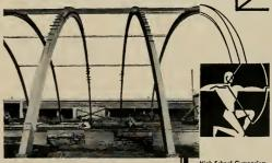
SUMMERBELL glued laminated arches, in any curvature and span desired, make it easy to plan gymnasiums and field houses totally free of obstructions. Fire safety, ease of erection, flexibility for all types of lighting and provision for large door and window openings are a few of the additional advantages. Write for illustrated brochure.
