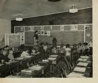
Economy roaf rafters become ceiling joists for classrooms. Note pitch af roof against far wall. Acoustical tile ceilings give good results here . . . blackboards placed against end brick wall.
