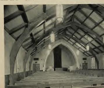
in every four feet, without glass being evident to the person in the pew. Since there is a basement below, the bottoms of the trusses were tied together with laminated beams supporting joist construction.
