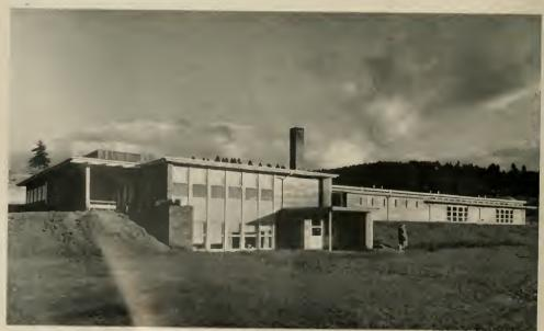
30 by 36 feet in size. All rooms are entered from a single-loaded corridor which parallels the class-rooms along each wing. Each room has an exit into the corridor and also an exit into a play and outdoor classroom area. These areas are separated from those of adjoining rooms by a screened shoulder-high wooden mask to give teaching privacy.
