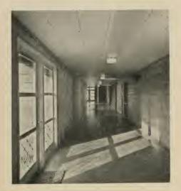
STANDARD corridor built as single laaded section paralleling each classroom wing. Note fir panelling used along walls to withstand heavy use.
