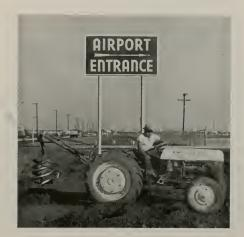
Newly developed mechanical auger is used for digging holes for planting of trees and shrubs.
