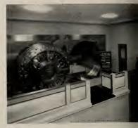
Giant modern Vault Daar in the safe deposit department of the new Anglo California National Bank in Oakland. The door is 22 inches thick, 9 feet in diameter, and weighs 70.000 pounds.
