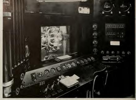
All of the operating controls and metering devices required for engine testing in the new "test cells," ore grouped around double-glazed observation windows in compact and convenient orrangement. Siz control desks, similar to one illustrated above, are paired in the control passages extending through the cell block. Sperry controls (left foreground) and potentiometer is mounted flush on desk ot right with slant gauge directly above window. Engine in position for testing is seen in test cell.
