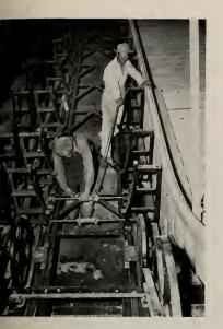
It takes a lot of work and equipment to install a modern electric stairway and pictured here is the first pair of step axles which form a continuaus moving chain that returns back underneath the upper moving surface. The heavy welded truss an the bottom carries the load with step roller tracks an each side. Flanking the tracks, foreground, are big sheaves for quiding the flexible rubber handrails.
