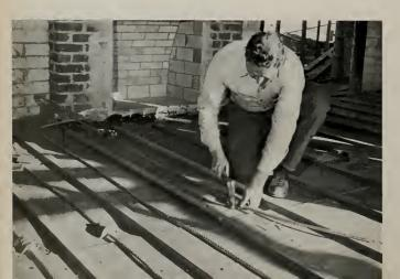
Wire Rope Cobles ore laid over gloss wool floor insulation with special clips for floor.
