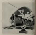
Manufactured by the Quijac Tool Company of Los Angele California, this portable machi: has an integrally-mounted ½ h. 110-volt, universal type AC-L motor with a direct gear drive the rollers. Gears are self lubric ing. Automatic trip switch star cutting operations when the cut wheel contacts the pipe and au. matically stops when the cut finished.
