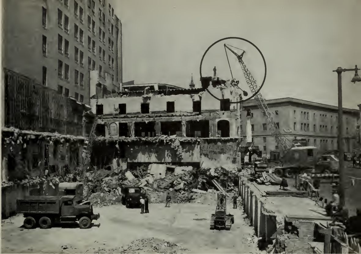
DEMOLITION BALL Wrecking Old Balconade Building (Note action in circle).
