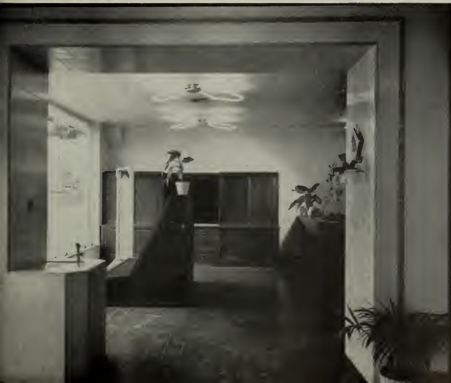
VIEW OF TILE SHOW ROOM FROM GENERAL OFFICES
