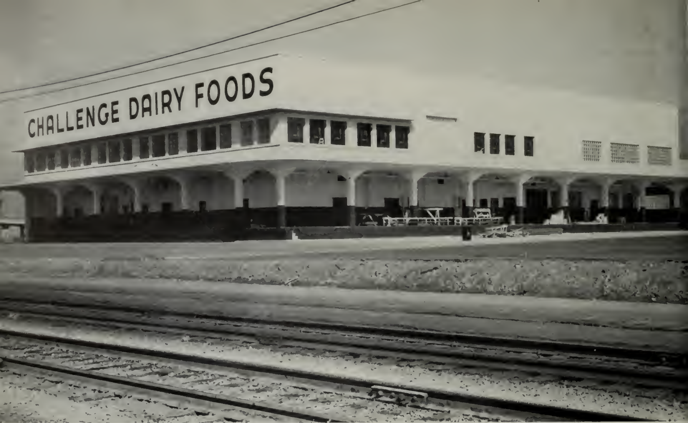
WESTERN VIEW OF THE MAIN PLANT
