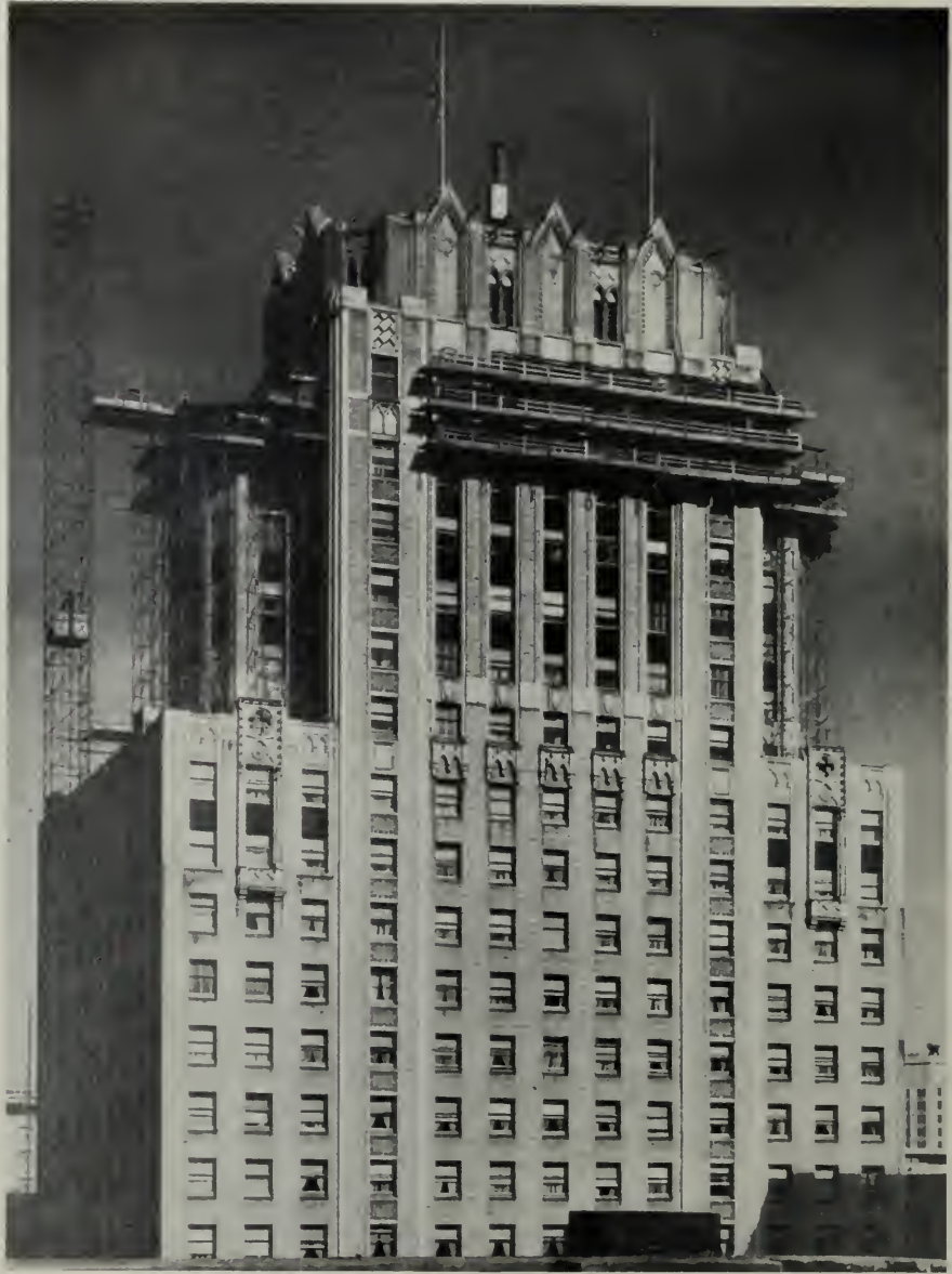
Illustrating use of scaffolding during STARLITE construction
