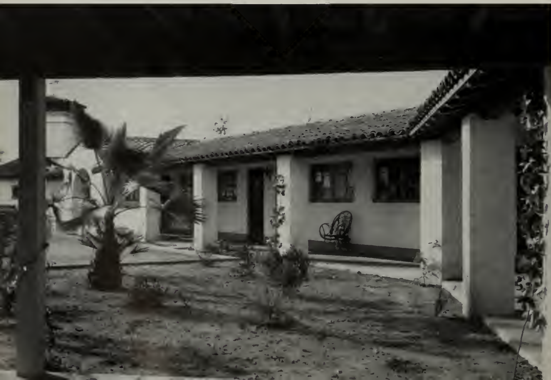
BELOW: Guest room buildings, exposed rafters, concrete block pillars and tile roof add to the pleasure of El Rancho.
