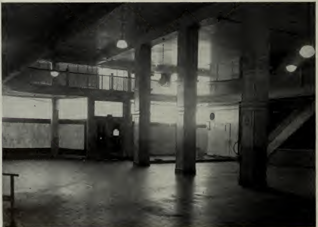
BELOW: Interior of the ground floor prior to remodeling. The problem of large center pillars and mezzanine space with unsightly stairway is clearly shown.
