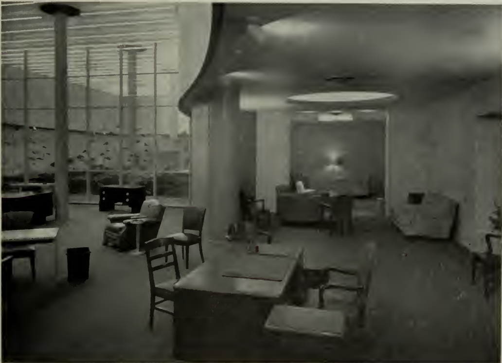
Modern Design of Interior—Indirect Lighting and Glass Partitions
