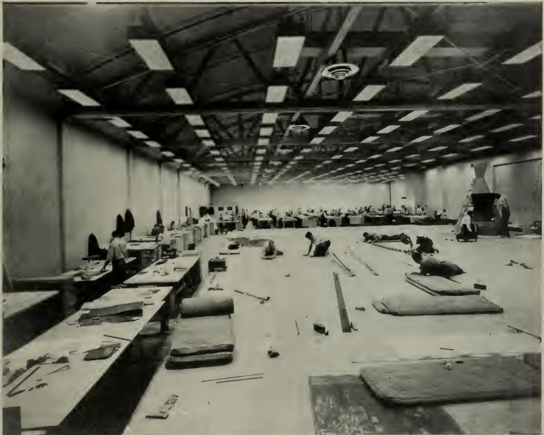
Air is distributed uniformly and without drafts over the vast floor area of this loft of the Vega Aircraft plant, at Burbank, California. By scientific air-diffusion, Anemostats (on the under-side of the trusses) insure equalization of both temperature and humidity.
