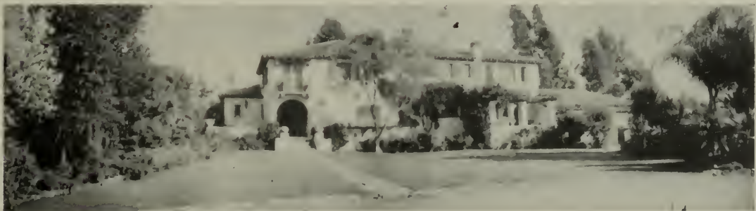
ONE OF THE FIRST RESIDENCES in RANCHO SANTA FE
