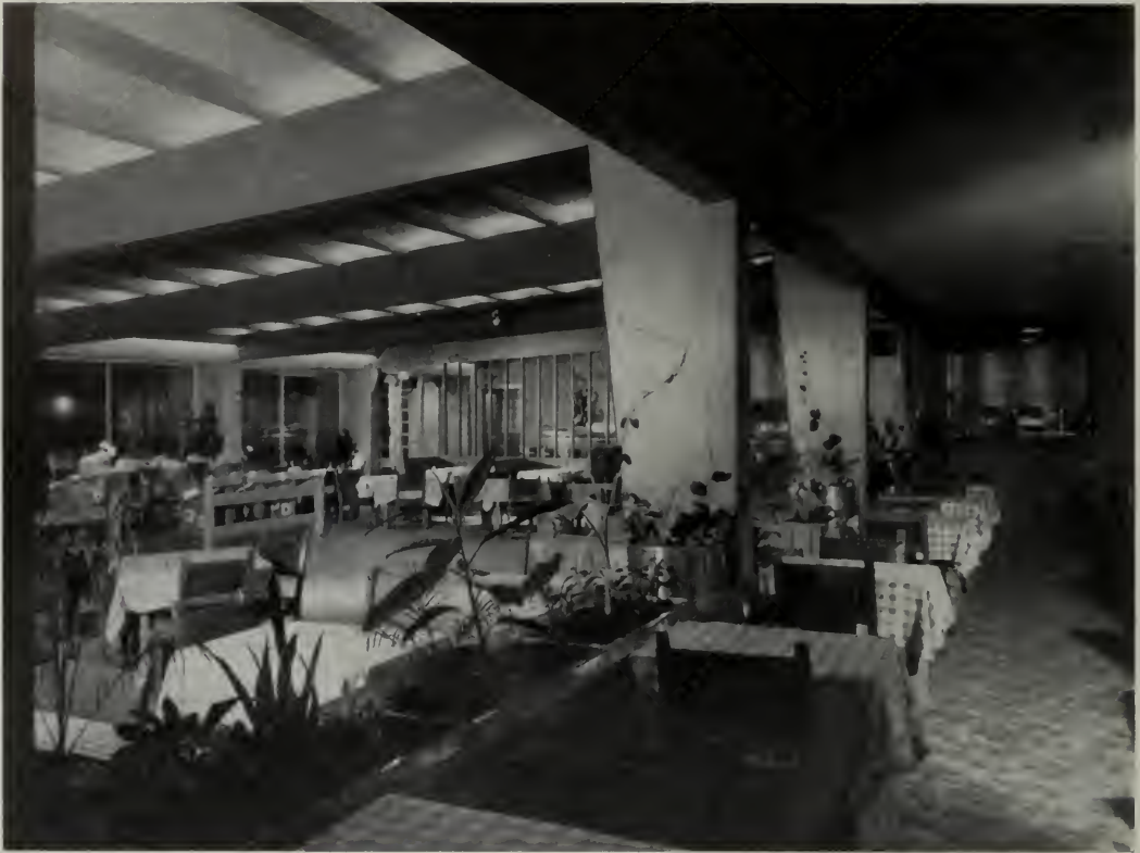
DINING ROOM: Unusual ceiling design featuring tube lighting on top of beams. Dance floor is in center, and copper planting boxes, natural stone, wood and leather fixtures contribute to the relaxing western atmosphere.
