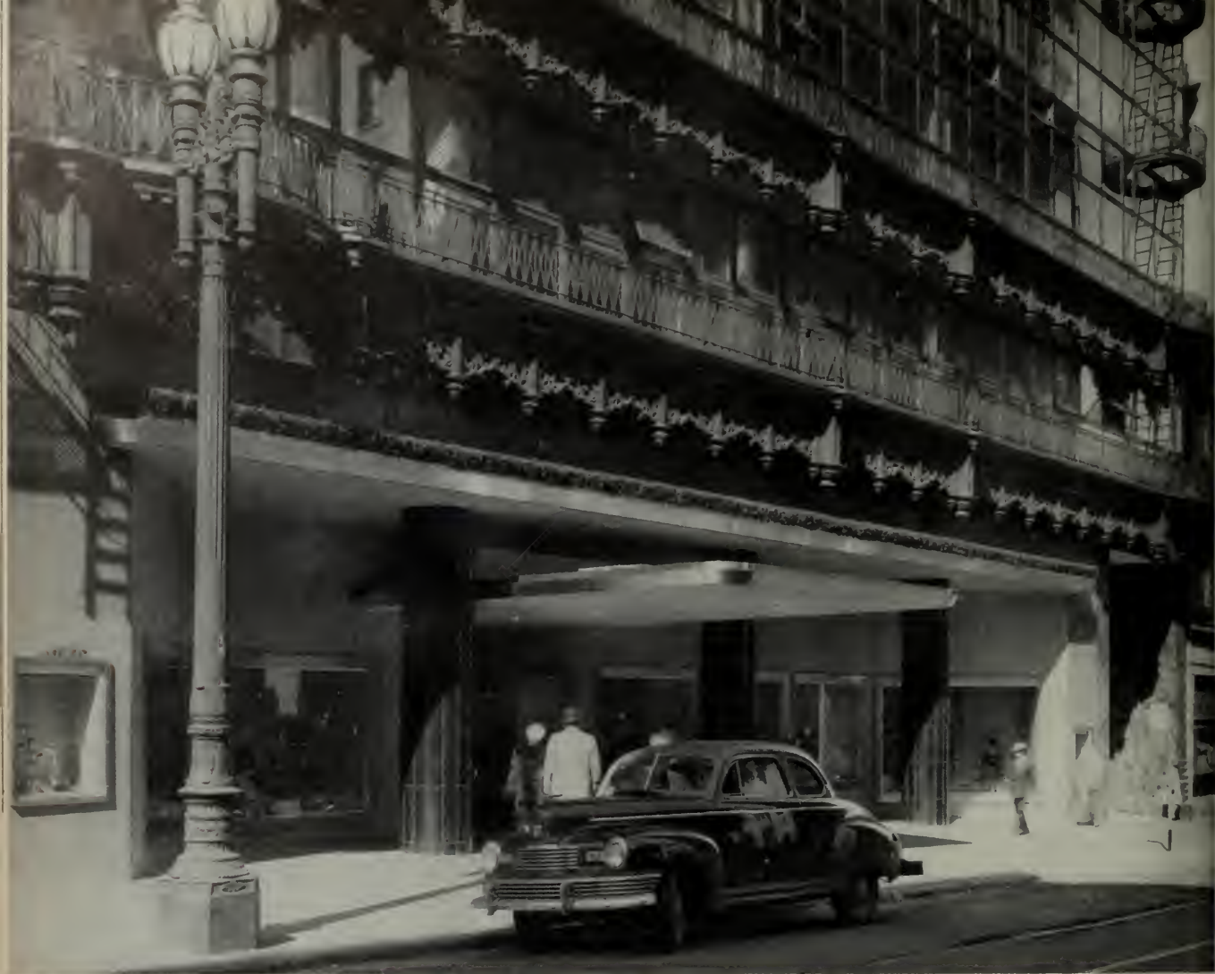
NEW STORE ENTRANCE—Recessed Display Windows
