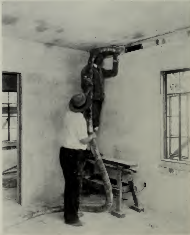
Insulation crew works between roof and top-floor ceiling
