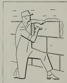
3. Ceramic Veneer is put in place, tapped to fill voids.
