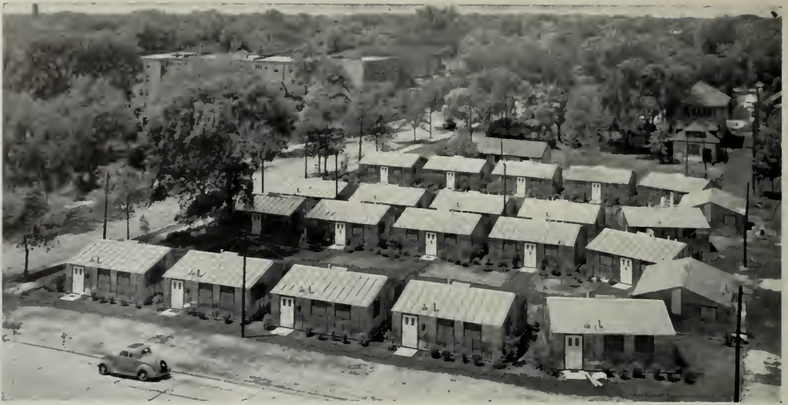
This aerial photograph shows part of a project which is alleviating the housing shortage at Northwestern University, Evanston, Illinois. The homes were furnished by The Steelcraft Mfg. Co. of Cincinnati, Ohio, who shipped all parts in convenient bundles to the campus grounds. The entire project, which now provides shelter for approximately 1000 veterans and faculty members, was completed within 90 days.
