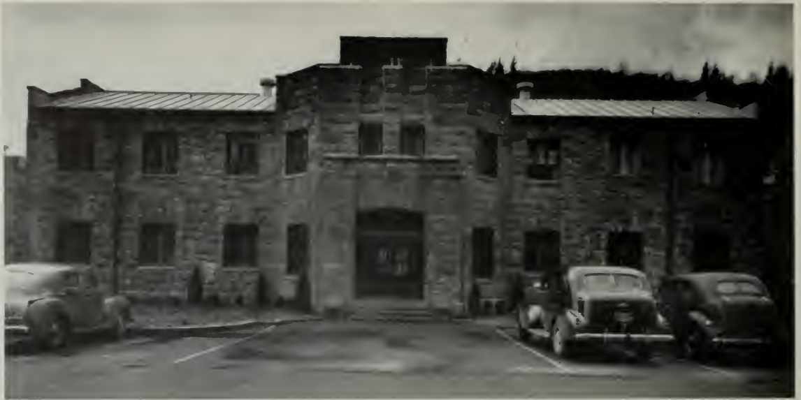
AMINISTRATION BUILDING . . . East Exposure
