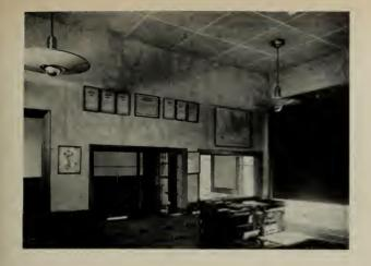
View at left: Interior of radio operations room showing Fiber-glas acoustical board on walls and ceiling.
