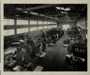
Parts for UTILITY APPLIANCES are die-formed on presses varying up to 375 tons pressure.
