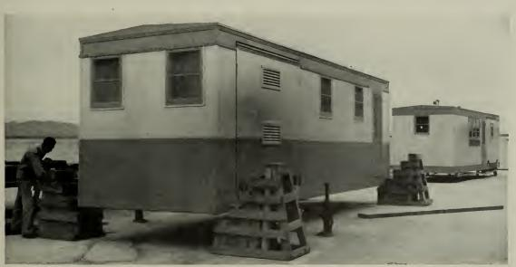
Simple method of loading and unloading a Wingfoot Home with little equipment calls for the use of jacks and house steps. The house is jacked up gradually to a height sufficient to back a trailer beneath it. Note that bedroom bays are collapsed to permit movement on the highway.
