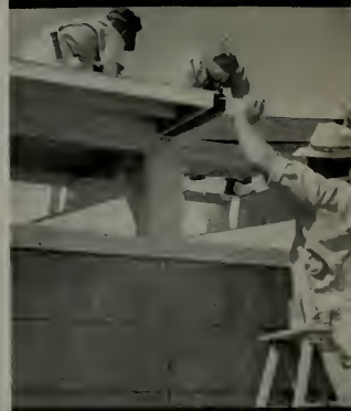
Dropping Roof Panel into Place
