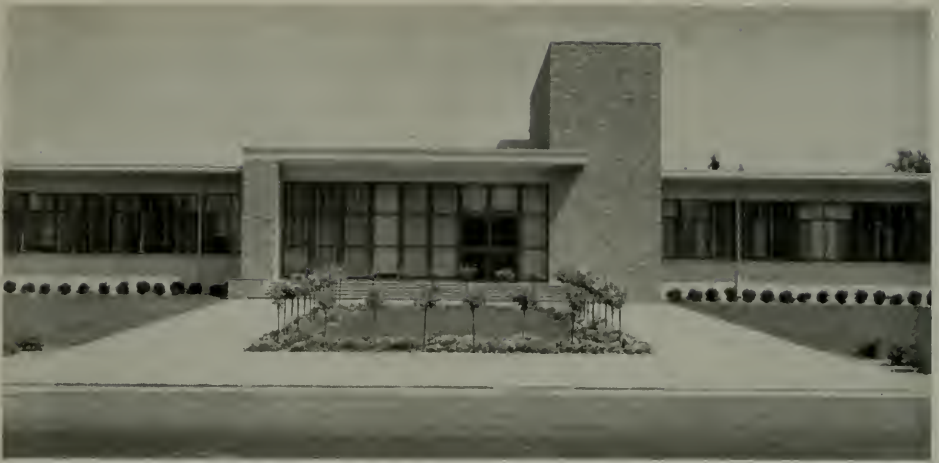
STREET VIEW OF ADMINISTRATION BUILDING, KAISER STEEL PLANT FONTANA, CALIFORNIA
