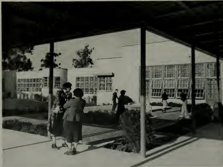
Because of its close proximity to the Douglas Aircraft factory, frequent additions to this school have been made in recent months. The building is an excellent example of the California open-type school, arranged around potios with open corridors supported on slender steel columns.
