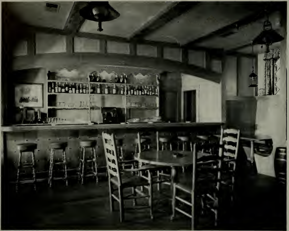
INTERIOR OF TAVERN, LOOKING TOWARD BAR, SANTA MARIA, CALIFORNIA Designed by Cheesewright, Mason & Company.
