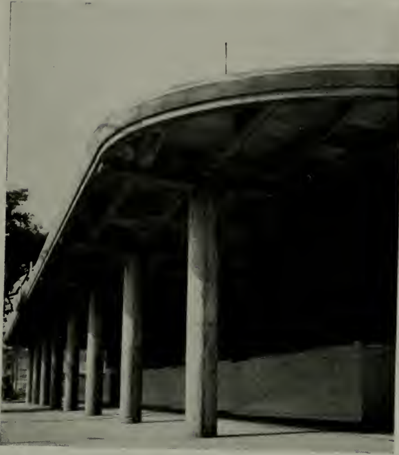
DETAIL OF ARCADE, LOCKHEED COMMISSARY BURBANK, CALIFORNIA
