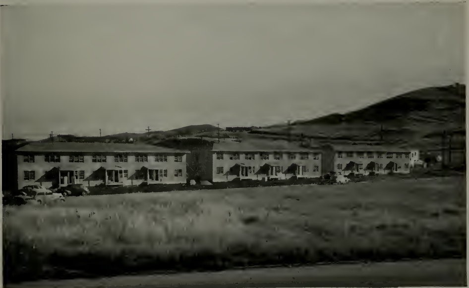
THREE OF 285 FOURTEEN-APARTMENT BUILDINGS AT RICHMOND, ALL OF WHICH WILL BE COMPLETED THIS MONTH—A 4,000-UNIT PROJECT FOR THE U. S. MARITIME COMMISSION
