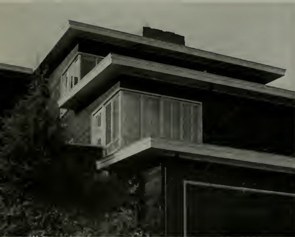
Detail of step-back living rooms and garage . . . exterior treated in natural Redwood.
