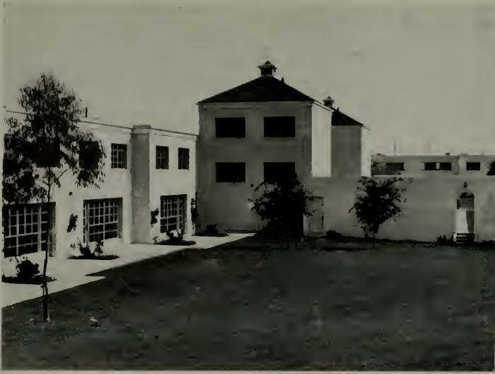
Height of apartment structures flanking garages is accentuated and roofs are hipped architectural variations. Garages are concealed from courts in this view.
