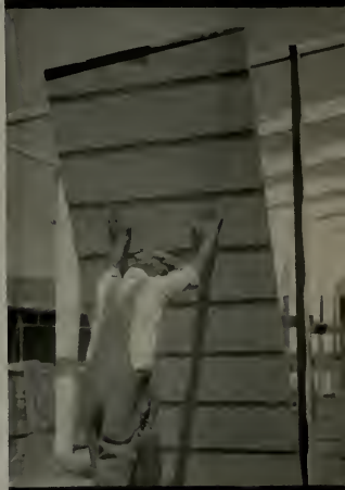
Assembling of Three-Hinged Arches
