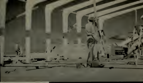
Assembling of Three-Hinged Arches
