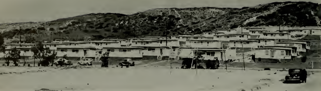
Los Altos Housing Project, Pacific Beach, San Diego. The site had been partly developed for a residential subdivision.
