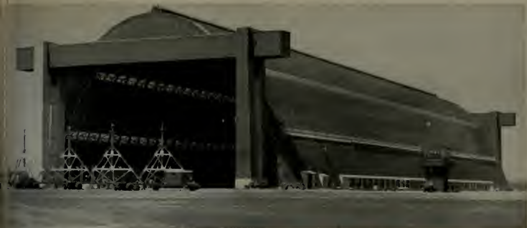
This wooden blimp hangar at the Naval Air Base, Santa Ana, California, is 171 feet high, and has a clear span across of 237 feet, largest ever erected.
