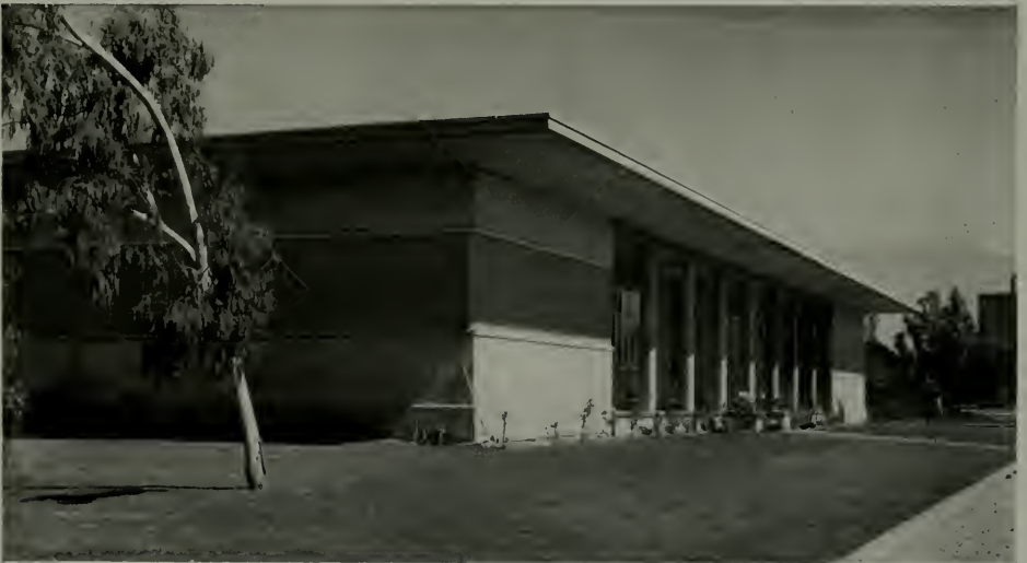
PHYSICAL TESTING LABORATORY, KAISER STEEL PLANT, FONTANA Birge M. and David B. Clark, Architects
