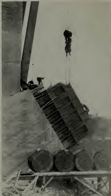
Placing of steel grillage section weighing 63\frac{1}{2} tons on anchor bolts at abutments.
