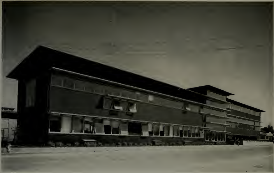
WEST SIDE OF BUILDING. NOTE LONG CORAL COLORED AWNINGS
