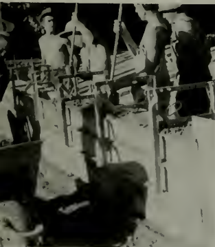
Tamping of typical form lift.
