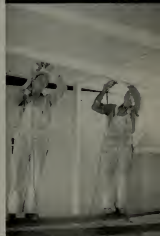
Fastening Roof Panel With Electric Screwdrivers
