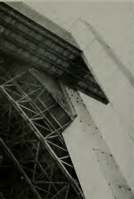
Left, folding doors at each end of hangar are supported by twin concrete pylons carrying an enormous built-up wooden "box beam." The doors fold up in recess between pylons.
