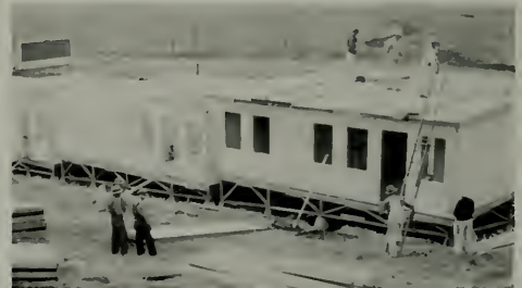
View shows prefabricated house erection in Vallejo with one roof section on the ground ready to be placed on the building.
