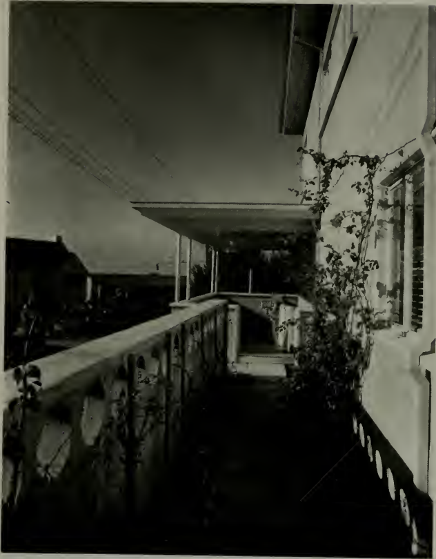
Left: Service walk, showing Concrete Grid Walls.
