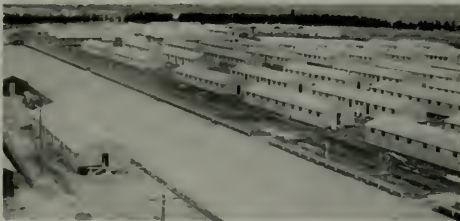
McCarthy-built barracks for housing alien evacuees at Tanforan Race Track. 170 barracks were built in 7 days against a time limit of 15 days.
