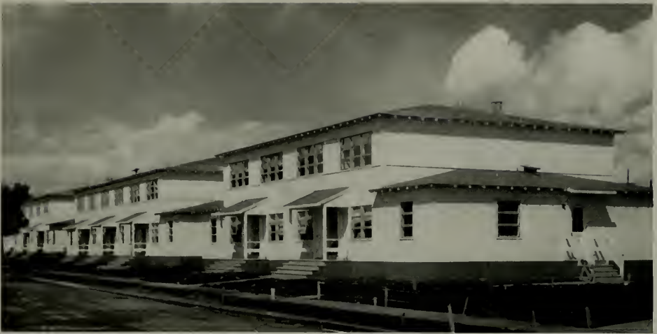
TYPE OF PERMANENT APARTMENT UNITS FIRST TO BE BUILT IN RICHMOND BY THE ROBERT McCARTHY COMPANY FOR U. S. MARITIME COMMISSION
