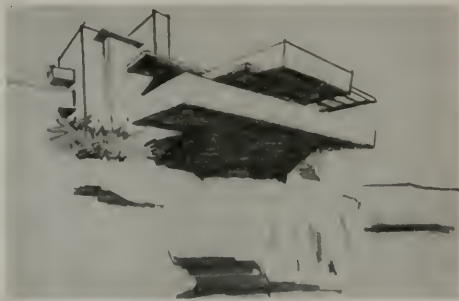
Falling Water House by Frank Lloyd Wright, an outstanding example of cantilevered construction
