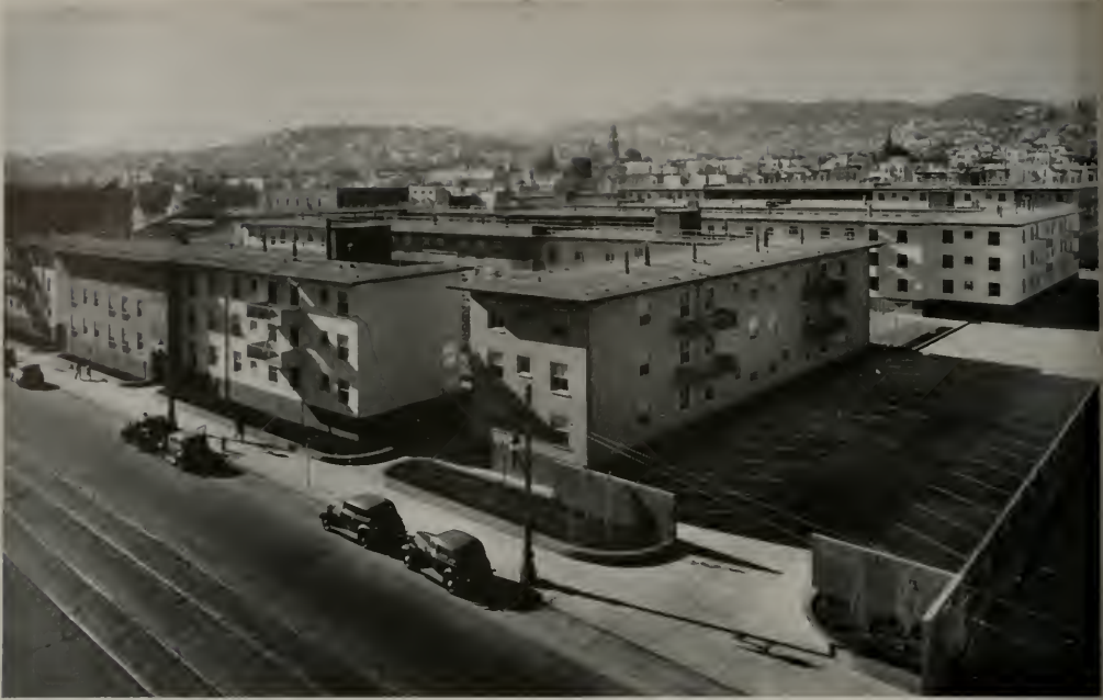
VALENCIA STREET FRONTAGE, LOOKING TOWARDS FIFTEENTH STREET, SAN FRANCISCO
