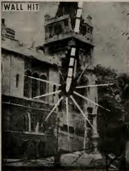
Bomb, in curving flight, went through side wall and blew up on third floor.
