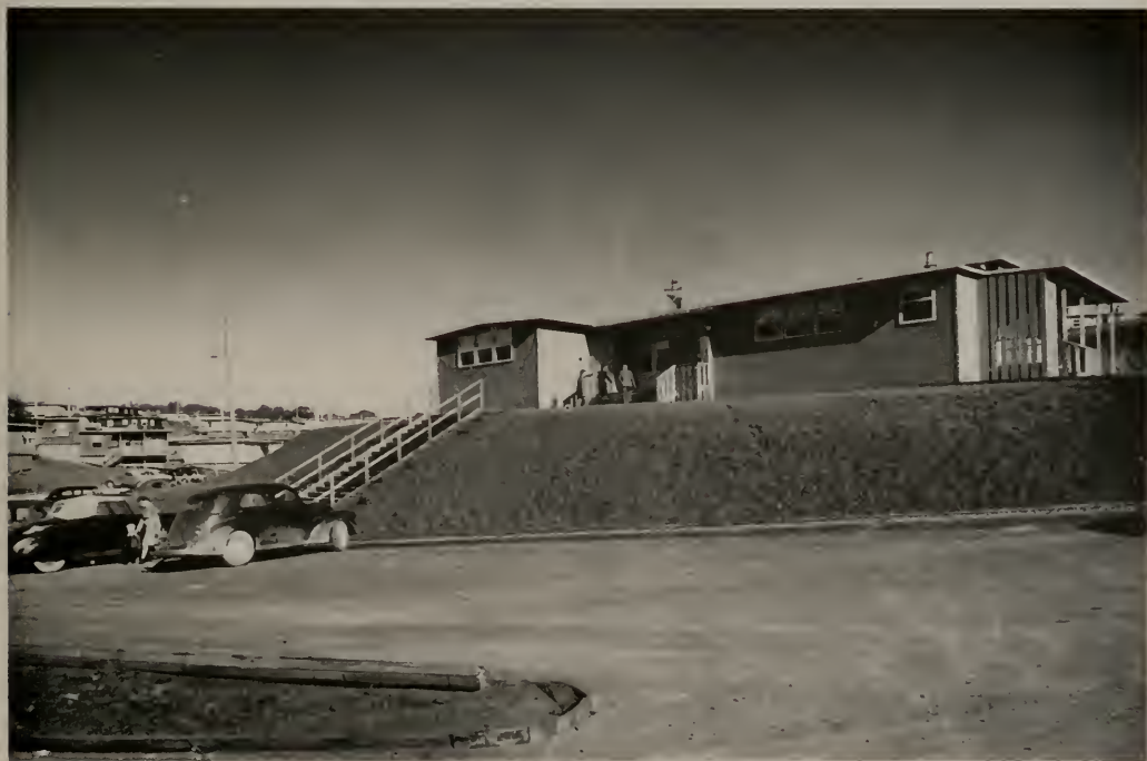
COMMUNITY CENTER—BUILT AT THE SITE BY CONVENTIONAL CONSTRUCTION Russell G. de Lappe, Architect
