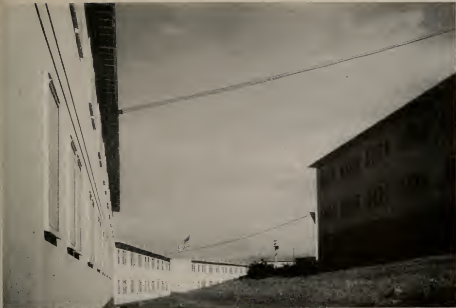
VALLEJO: Grouping of Dormitories conforms to convex hillside.
