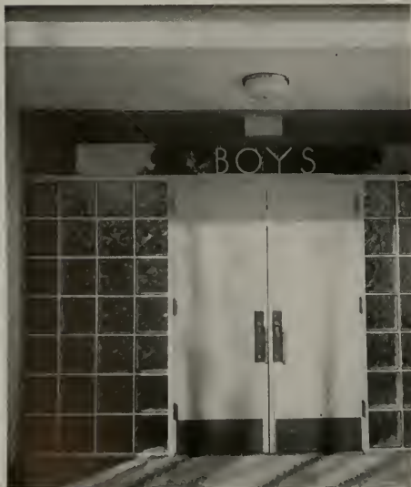
ENTRANCE TO BOYS' LOCKER AND SHOWER ROOM
