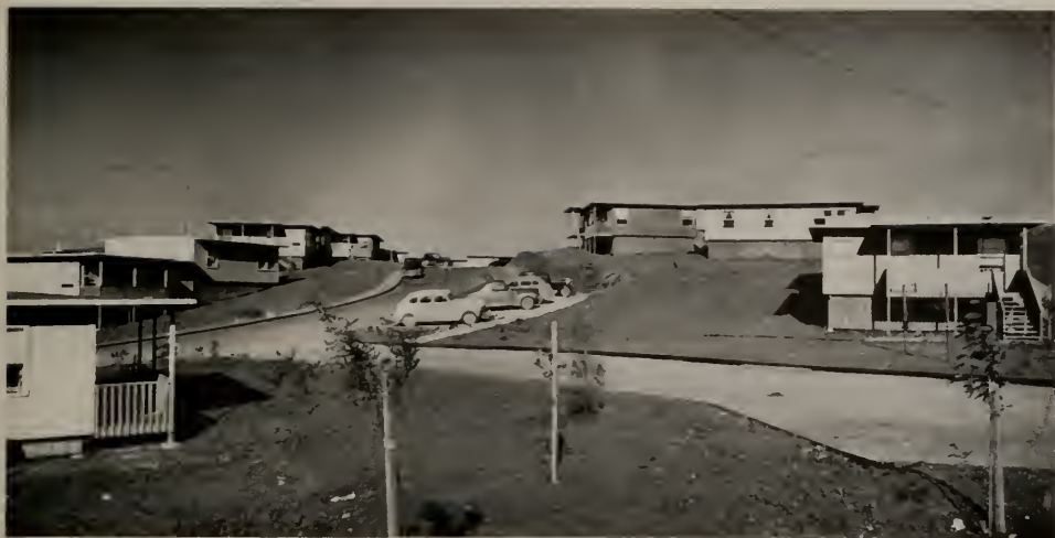
EXTERIORS ARE REDWOOD SIDING, FACTORY-FINISHED, SOME WITH PAINT, SOME WITH PIGMENT STAIN Russell G. de Lappe, Architect
