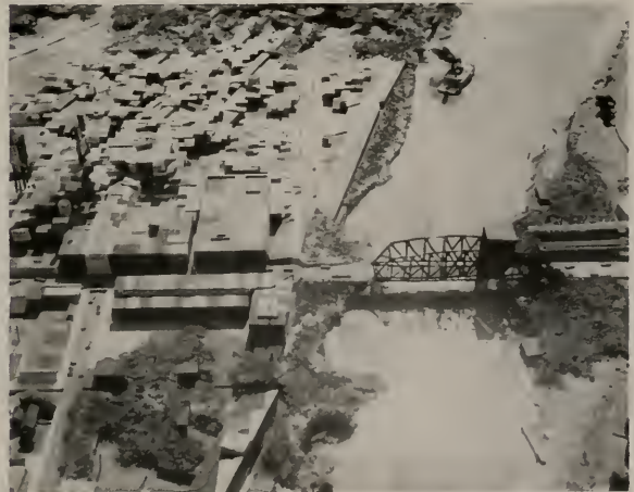
The same scene after the camoufleur has applied his art. Screening of river house, wharves, bridge; narrowing of river (through use of floating nets); disruptive painting—all combine to confuse the approaching bombardier.
