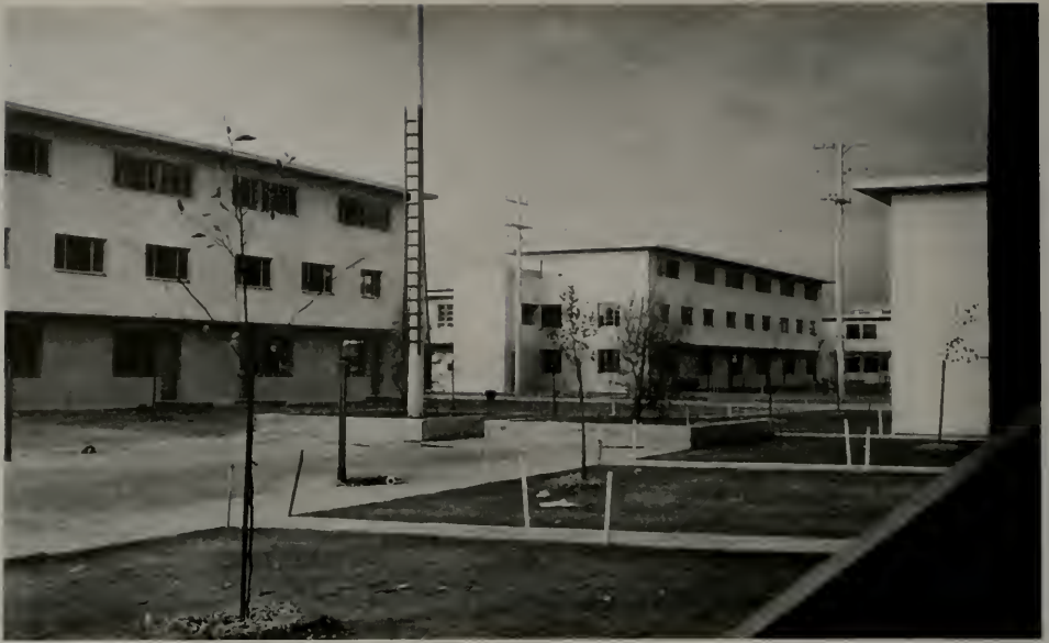
Spacious Lawns Will Improve Appearance of These "U" Buildings Of Which There Are Twelve
