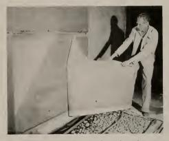
from the concrete, after the forms have been removed, leaving a surface which is smooth and attractive in appearance without refinishing.
