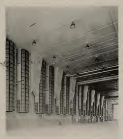
Glass fiber air filters arranged in 912 cells, each cell cantaining faur filters, line the wall through which the washed, warmed and filtered air enters the enclosure
