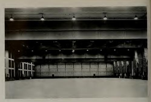
The filter panels through which the washed, warmed and filtered air enters are at the right. The exhaust units are at the left.
