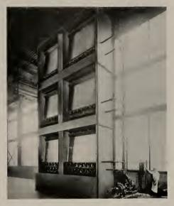
One af the exhaust units in the fabricating shap, prior to installation
