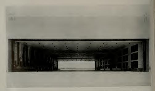
View through the enclosure, with end doors rolled up to permit entrance of bombers. The air filters through which the air passes the enclosure are at the left; the exhaust units at the right.
