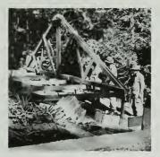
Standard 32-foot span timber roof truss for warehouse at Forest Service Experimental Range Station, Strawberry, Calif. 21/2" TECO split ring connectors at all joints.
