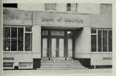
Entrance detail, faced with N. CLARK & SONS CERAMIC VENEER. Also showing use of Alameda Quarry Tile for stair treads and risers.
