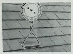
A FORCE OF 85 POUNDS IS REQUIRED BEFORE A PROPERLY NAILED CEDAR SHINGLE OF AVERAGE WIDTH CAN BE PULLED FROM A ROOF, SHOWING REAL WIND RESISTANCE
