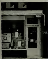
Store front, New York. Chas. Telchin & F. Ginna, Architects.
