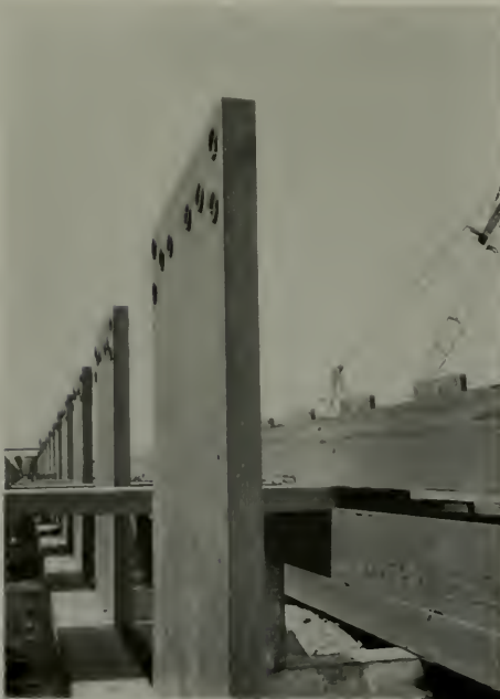
SPECTACULAR USE OF PLYWOOD AT THE GOLDEN GATE INTERNATIONAL EXPOSITION WHERE, IN THE COLONNADE OF STATES, 48 GIANT COLUMNS, 104 FEET IN HEIGHT, ARE BEING BUILT WITH WEBS 3" THICK, 29 PLY HOT-PRESSED, RESIN-BONDED PLYWOOD. THESE GUSSET PLATES ARE JOINED WITH SPLIT RING CONNECTORS. T. L. PFLUEGER, ARCHITECT.
