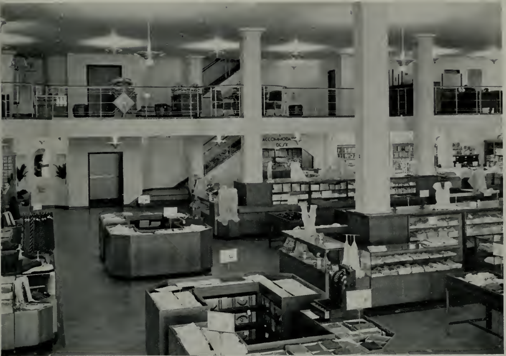
PART OF FIRST FLOOR AND MEZZANINE, ROSENBERG'S, SANTA ROSA Hertzka and Knowles, Architects
