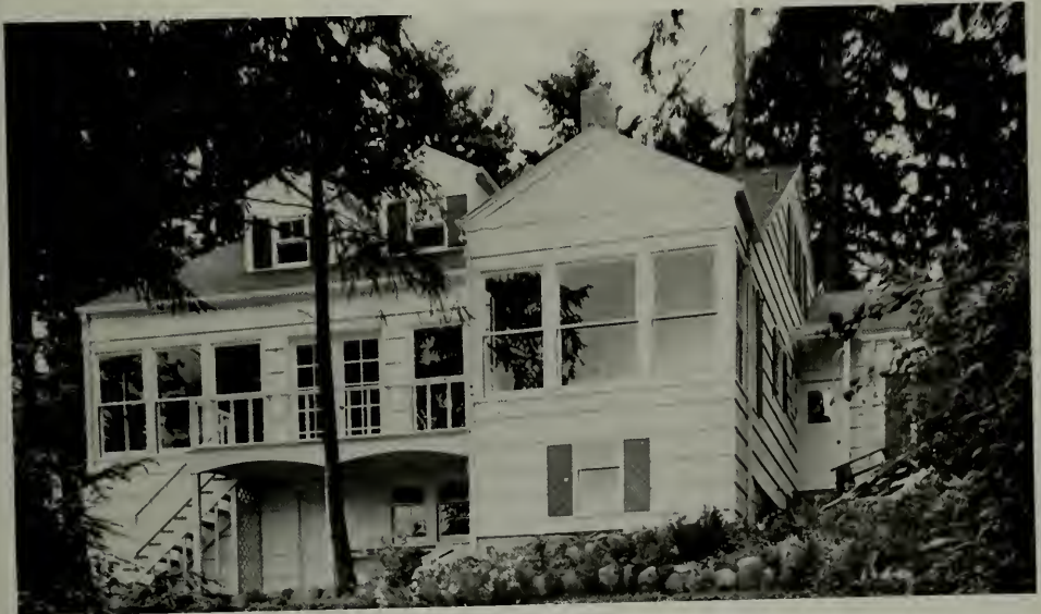
THE CLARK HOUSE AFTER ALTERATIONS AND ADDITIONS. ROOF IS RED CEDAR SHINGLES APPLIED TO 5/16" DOUGLAS FIR PLYWOOD SHEATHING SILAS E. NELSON, ARCHITECT
