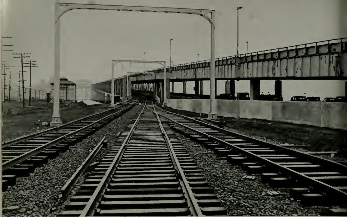
Where Bay Bridge trains will enter and leave the easterly end of the span.
