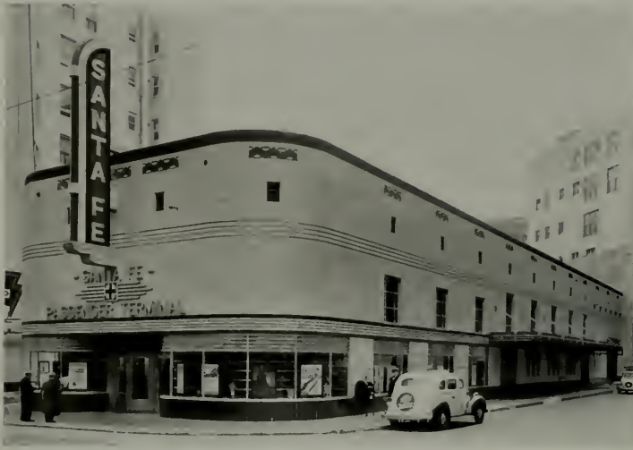
SANTA FE PASSENGER TERMINAL San Francisco
