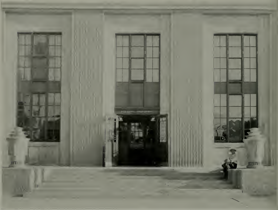
DETAIL OF ENTRANCE, REDDING POST OFFICE BUILDING, REDDING, CALIFORNIA ALBERT F. ROLLER, ARCHITECT
