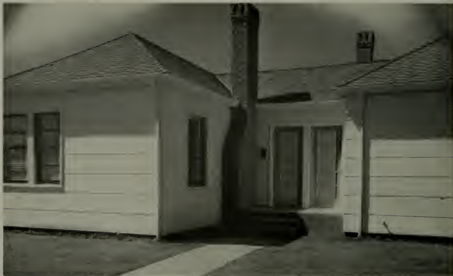
HOUSE FOR A. R. BRADLEY, ALBANY, OREGON Exterior of hot pressed resin-bonded Douglas fir plywood.
