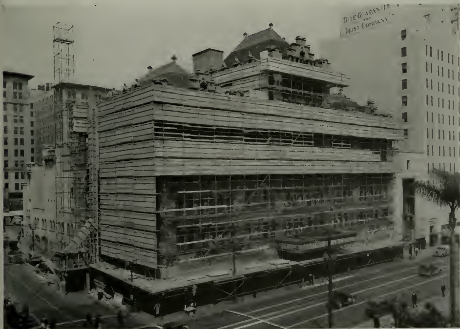
NEW PHILHARMONIC BUILDING, FORMERLY THE AUDITORIUM, LOS ANGELES Douglas fir plywood protective covering used while old face of building is being lifted for new.
