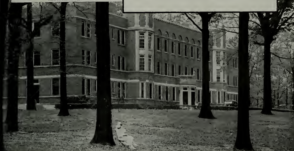
St. Mary's Hospital, Knoxville, Tenn. Crowe and Schulte, Architects. 125 Johnson room thermostats control 154 Johnson radiator valves
