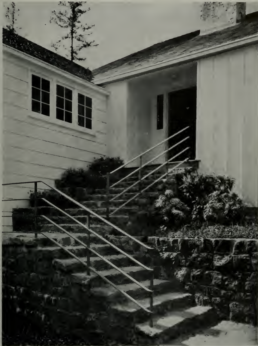
ENTRANCE FRONT, RESIDENCE FOR MR. AND MRS. ROBERT ARNESON, LAKE OSWEGO, OREGON
