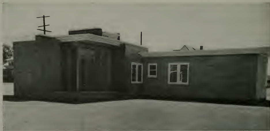
ULTRA MODERN HOUSE FOR R. A. SWANSON, ALBANY, OREGON, FROM PLANS BY FRANK LLOYD WRIGHT; R. C. MILLER, BUILDER Exterior of brick and hot pressed resin-bonded Douglas fir plywood with redwood face ply.
