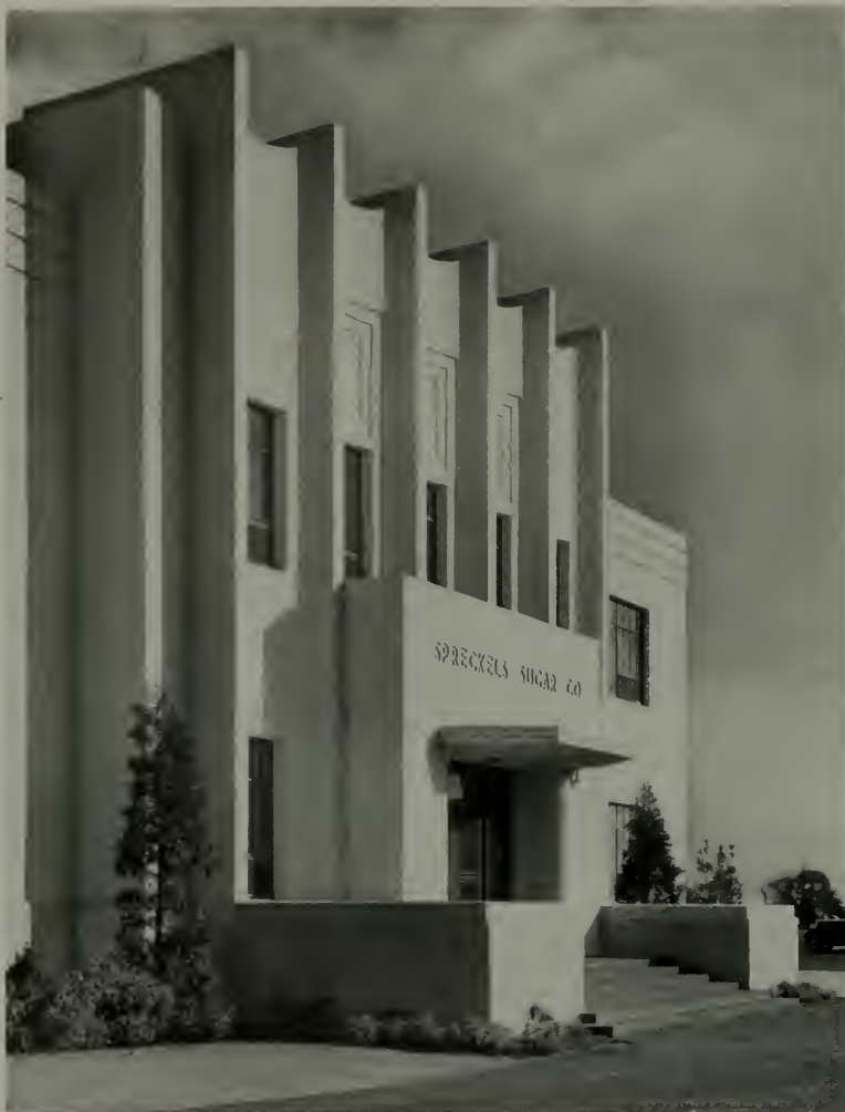
DETAIL OF ENTRANCE, SPRECKELS SUGAR PLANT, NEAR WOODLAND, CALIFORNIA Geo. W. Kelham, Harry A. Thomsen, Jr., Architects
