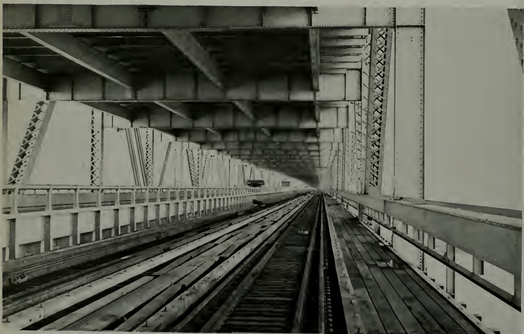
Looking down the East Bay Crossing shows ties and tracks in place.
