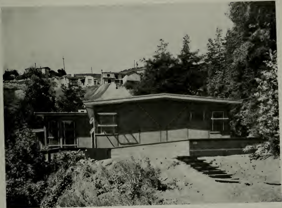
HOUSE FOR PROFESSOR ROBERT TRYON, BERKELEY, CALIFORNIA MICHAEL GOODMAN, ARCHITECT Exterior of \frac{1}{4} " plywood panels over sheathing used experimentally.
