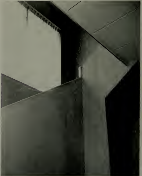
A STAIRWAY OF PLYWOOD IS FINISHED NATURAL WITH WHITE SHELLAC AND WAXED TO GIVE A SOFTER GRAIN TONE.
