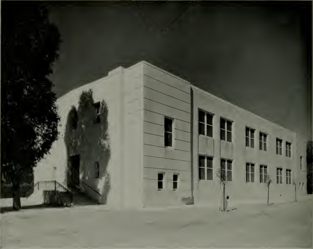
CLASSROOM BUILDING, VAN NUYS HIGH SCHOOL, VAN NUYS, CALIFORNIA ALLISON & ALLISON, ARCHITECTS
