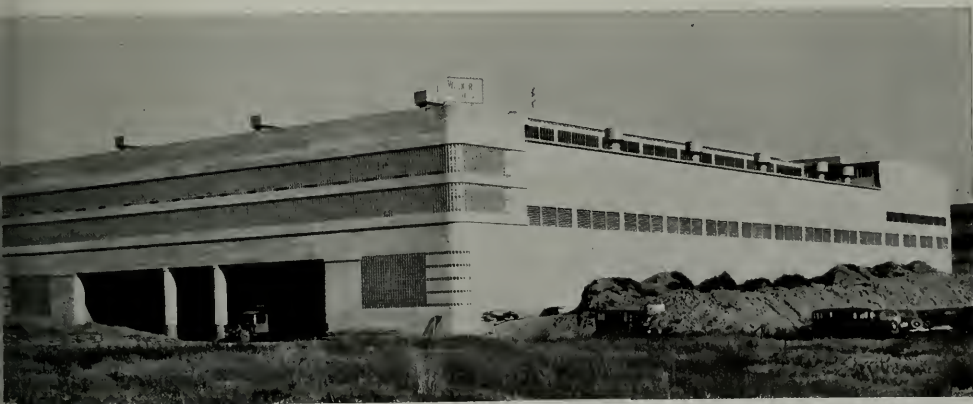
COMPLETED UNIT OF OWENS-ILLINOIS PACIFIC COAST COMPANY PLANT, LOS ANGELES Albert F. Roller, Architect
