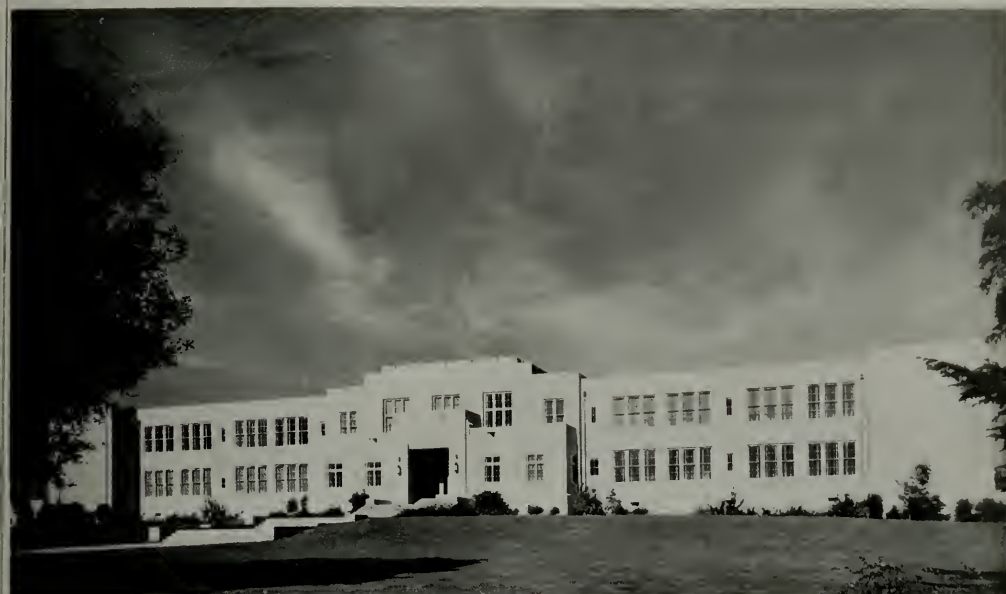
CENTRAL ELEMENTARY SCHOOL, HUNTINGTON BEACH, CALIFORNIA ALLISON & ALLISON, ARCHITECTS
