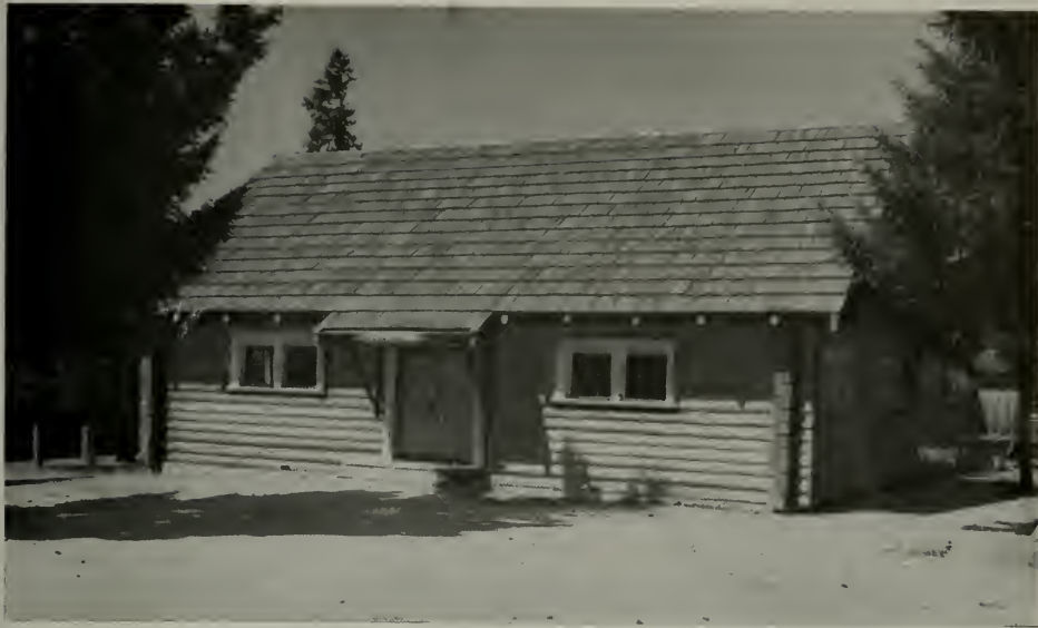
PACK HALL, THE ORIGINAL CLASS ROOM BUILDING FOR UNIVERSITY OF WASHINGTON RESEARCH, DOUGLAS FIR FOREST, 30 MILES EAST OF TACOMA, WASHINGTON
