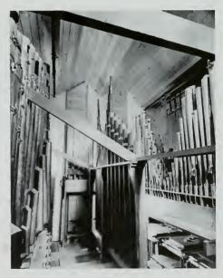
The interior of one of the two organ reverberation rooms showing the introduction of "splayed" ceiling to eliminate any parallel surfaces.
