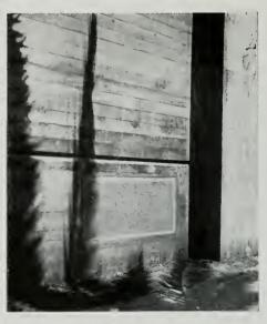
LEFT—DETAIL OF INNER FORMS OF BOX GIRDER, showing open-bottomed unit, combining forms of girder webs, cross diaphragms and bottom fillets.
