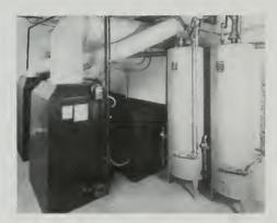
SHOWING FORCED AIR. GAS FURNACE AND AUTOMATIC WATER HEATING IN-STALLATION IN PASEMENT
