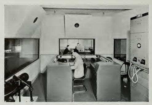
In the foreground is the console of the master control room of Warner Brothers KFWB, with the announcers' studio showing through the glass panel. This room is finished in a grey to match the instrument racks.
