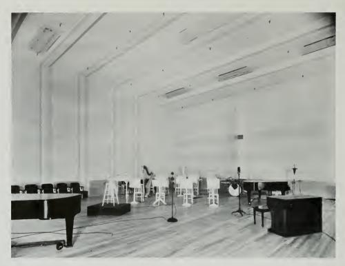
Studio Five in Warner Brothers KFWB at Hollywood was planned for the presentation of orchestra and choruses without audience, and its acoustical design allows placing the source of sound to any point desired in the room. Six different materials were used in the wall construction. Elimination of the wainscoting proved a distinct aid in the control of flutter echoes.
