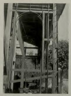
STEEL FRAME HOUSE-Exterior view at south end of garage showing method of using  $3_A$ " furring channels around corners and method of using  $3_A$ " furring channels for arched window openings.
