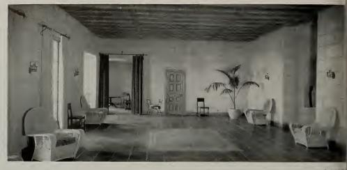
CAST-IN-PLACE CONCRETE FLOORS FOR APARTMENT BUILDINGS AND RESIDENCE. The integrally colored concrete floor finish in this building has been marked off in squares with a cuttin tool. Highly polished with wax, this type of floor harmonizes with the quiet dignity of the interior decoration.
