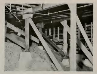
Intermediate piers should be carried well above the ground line to prevent any possible ground contact by the wood columns. Dirt tends to slide down such embankments and pile up against the wood members, providing easy entrance by termites into the building.
