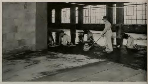
REMOVING EXCESS WATER BY THE USE OF AN ABSORBENT COVERING
