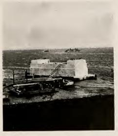
The first pier completed for the San Francisco-Oakland Bay Bridge, foot of Harrison Street, San Francisco. The pier stands 40 feet out of water and is 52 feet wide hy 122 feet long.
