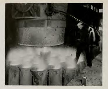
TEEMING MOLTEN STEEL AT PITTSBURG PLANT OF COLUMBIA STEEL COMPANY
