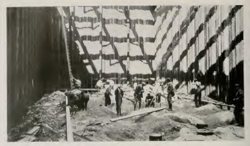
SAN FRANCISCO-OAKLAND BAY BRIDGE. INTERIOR OF A SHEET PILING COFFERDAM AT PIER E-20
