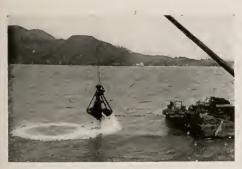
CLAM SHELL BUCKET USED TO REMOVE ROCK BLASTED 100 FEET BENEATH THE WATER
