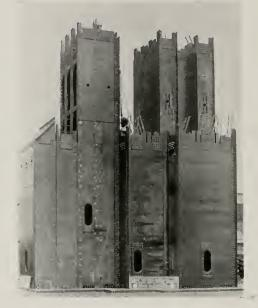
TRIAL ERECTION, BOTTOM PORTION OF EAST LEG OF MARIN TOWER Height fifty feet, weight 750 tons
