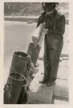
LOADING large casing bombs with 60 per cent dynamite. The bombs are 8" in diameter and 22' long. They hold from 100 to 350 pounds of dynamite.
