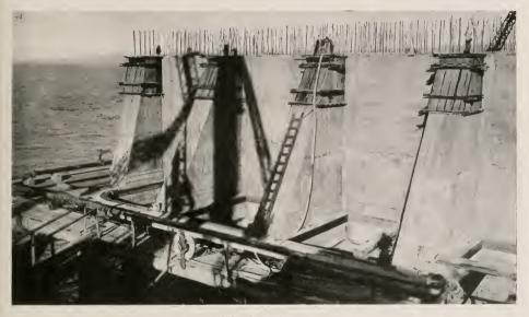
TOP OF PIER E-5, SAN FRANCISCO-OAKLAND BAY BRIDGE This picture was taken December 1, 1933, when the first pour began to taper off, with thre foot thick buttresses at each cells cross wall. Pier will go to a final depth of 170 feet. Its bottom now rests 121 feet below water level.
