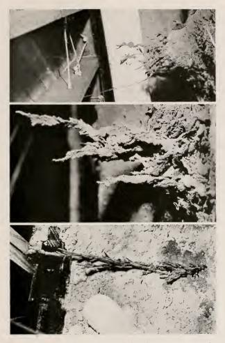
Fig. 5-Runways, tubes and towers made by subterranean termites under houses. Top-Branched tubes originating from a wood spreader embedded in concrete foundation. Wood forms had been left on the outside concrete wall of the building, which was only two and a half years old. Center-Towers of the western subterranean termite. Bottom-Towers and tubes of the western subterranean termite, from a stump left under a house.
