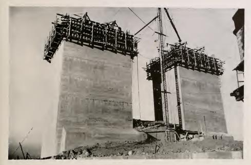
GOLDEN GATE BRIDGE SHOWING PYLON S1. SAN FRANCISCO SIDE ELEVATION APPROXIMATELY 90 FEET: FINAL ELEVATION, 250 FEET
