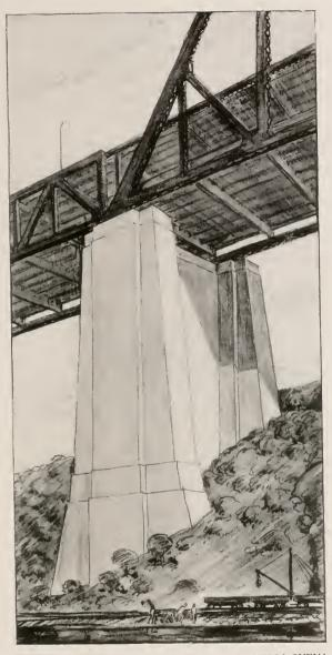
PIER EI ON ARMY POINT, EAST SIDE OF YERBA BUENA ISLAND. EXCAVATION FOR THIS PIER IS COMPLETE
