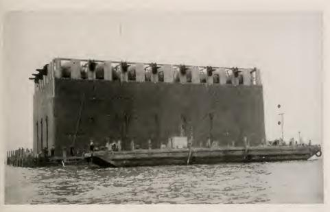
WEST BAY CAISSON A steel and timber structure the size of a small apartment house, anchored 1100 feet west of Verba Buena Island where it will be sunk to rock approximately 170 feet below the water line to establish the most castery tower of the supersion sector of the San Francisco-Oakland Bay Bridge. This caison is 74 feet wide, 127 feet long, 65 feet high, drawing 20 feet of water, and contains 28 steel cylinders, each 15 feet in diameter, now filed with compressed air to supply buoyancy.
