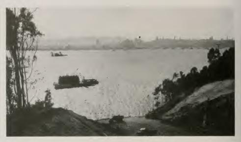
Photograph taken south of the west approach cut to the Yerba Buena Island Tunnel, showing cut in foreground made ready for the deck of the bridge.
