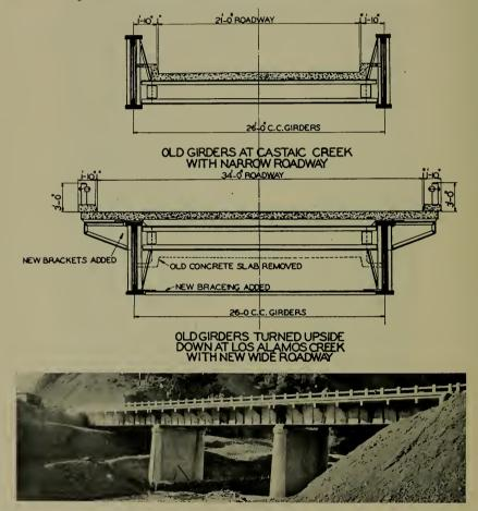
View of bridge after taking the surgical treatment that dismembered it and turned the 80-foot steel girders bottom-side up. It is now a perfectly modern structure with a 34-foot roadway, spanning Los Alamos Creek, on the new Ridge Route alternate.
