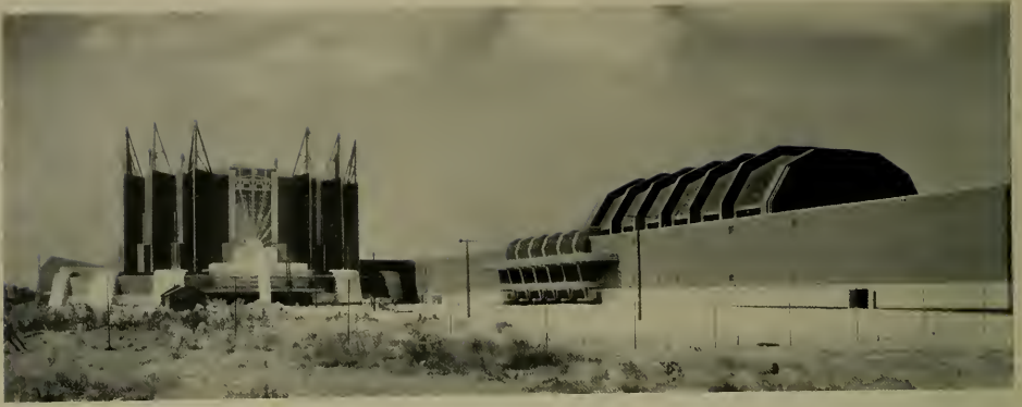
TRAVEL AND TRANSPORT BUILDING, CENTURY OF PROGRESS, CHICAGO The building represents the first application to architecture of the suspension bridge principle. It is 1000 feet long.
