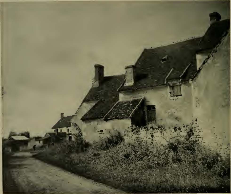
NEAR ORLEANS, FRANCE—A STUDY IN VERTICAL ROOF PLANES AND WALL TEXTURE
