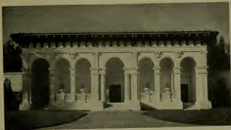
LOGGIA, CATACOMBS OF CYPRESS LAWN, SAN FRANCISCO B. J. S. Cahill, Architect
