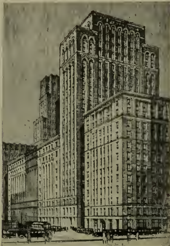
Another Lindgren & Swinerton, Inc. Contract Completed 22 STORY MILLS TOWER, SAN FRANCISCO LEWIS P. HOBART, Architect
