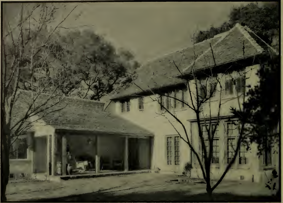
Roofed with N. Clark & Sons Sussex shingle tile
