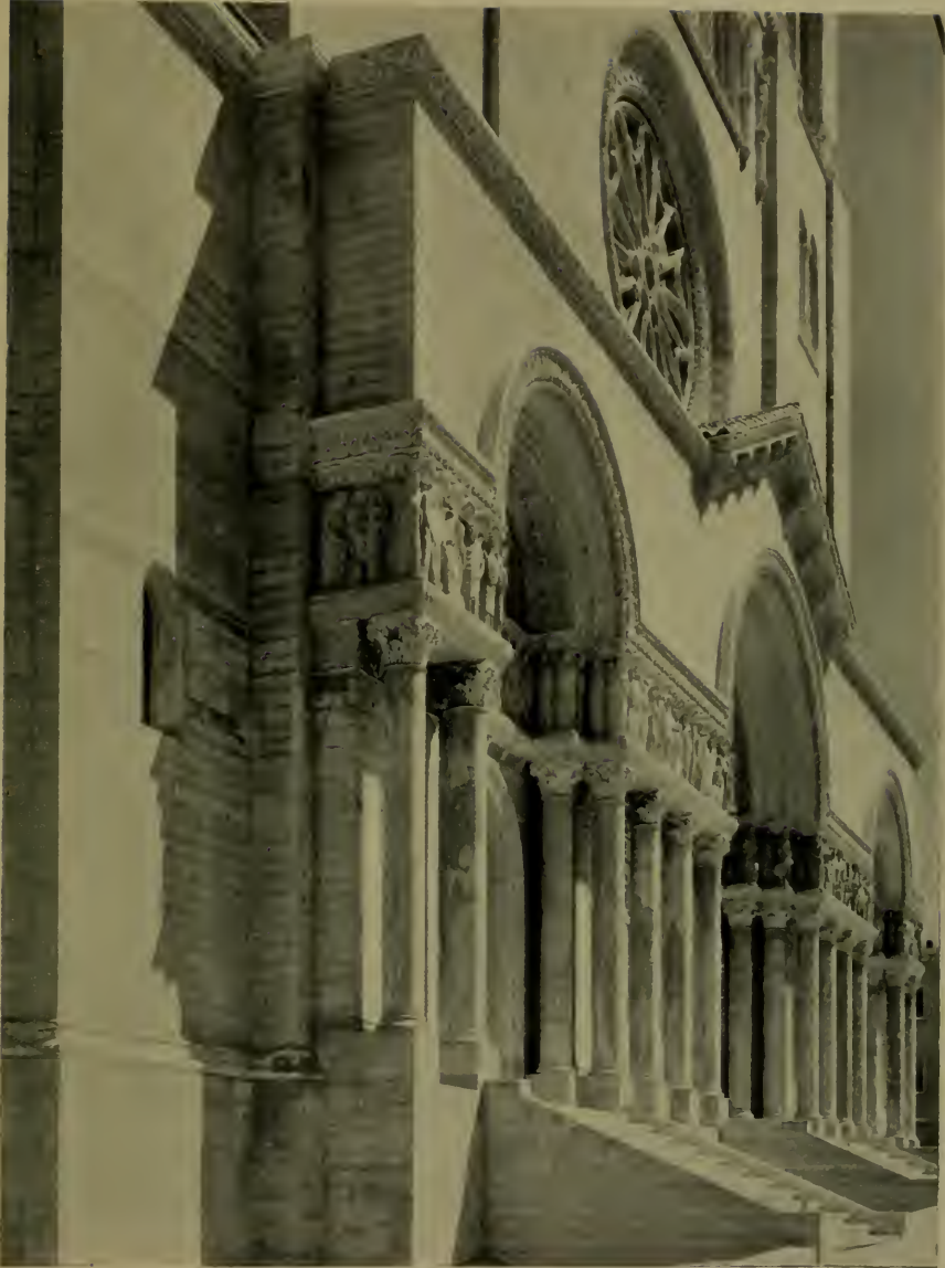
MAIN FACADE, ST. ANNE'S CHURCH, SAN FRANCISCO WILL D. SHEA, ARCHITECT
