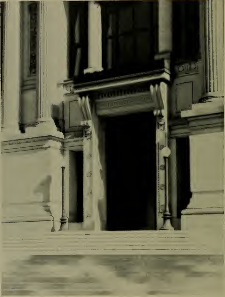
AN INTERESTING ENTRANCE DETAIL
