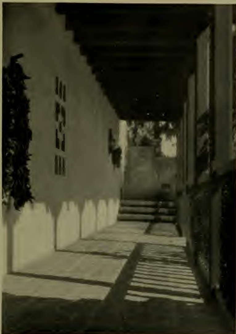
NORTH LOGGIA, RESIDENCE OF GEORGE FRIEND, ARLINGTON ESTATES, BERKELEY EDWIN LEWIS SNYDER, ARCHITECT
