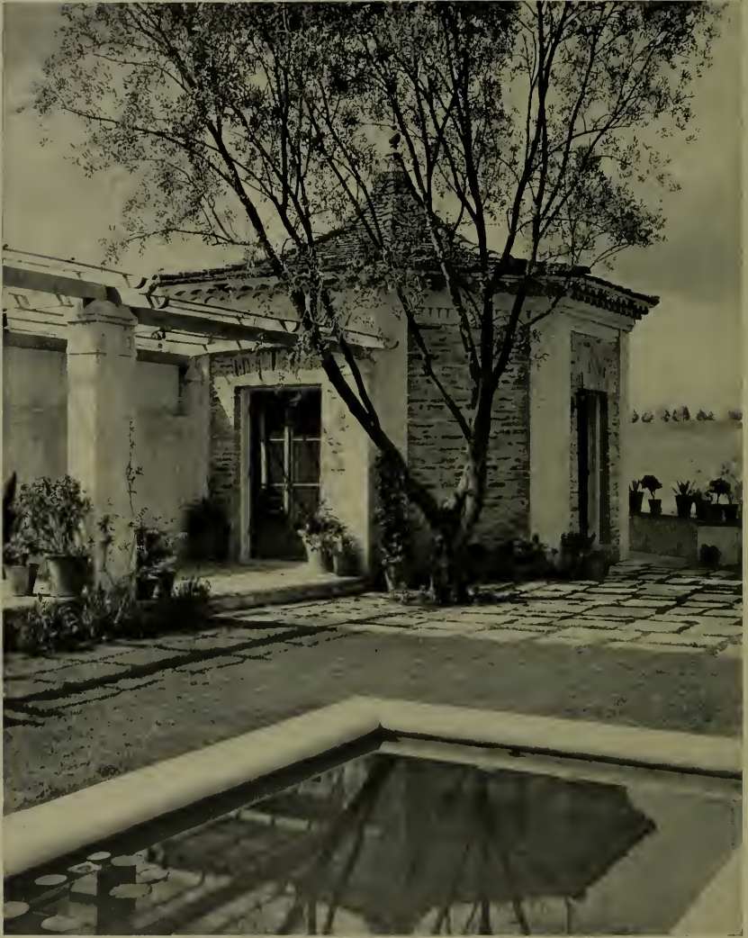
SUMMER HOME OF PAUL H. HELMS, BEVERLY HILLS GORDON B. KAUFMANN, ARCHITECT
