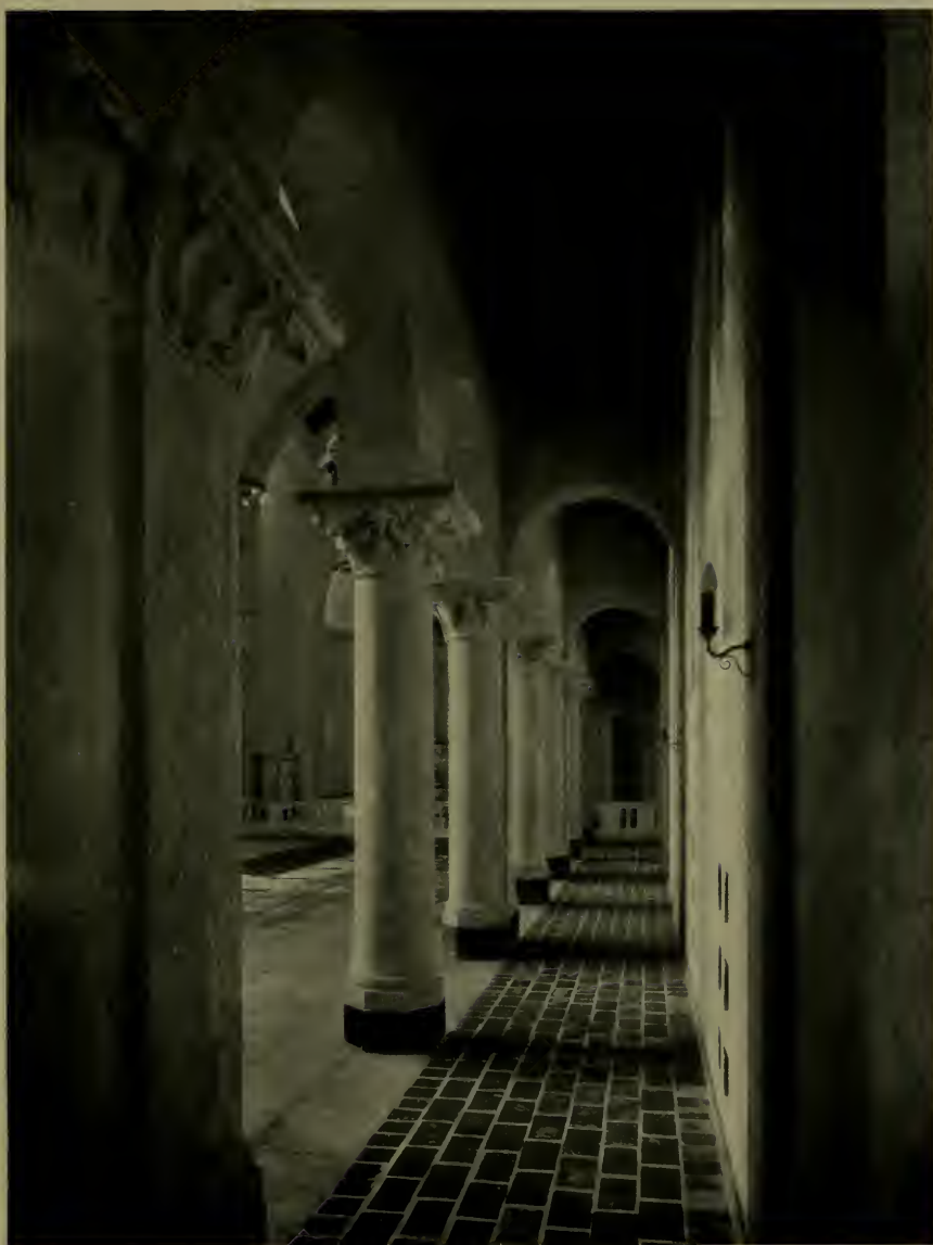
Column, caps, etc., poured monolithic in place
