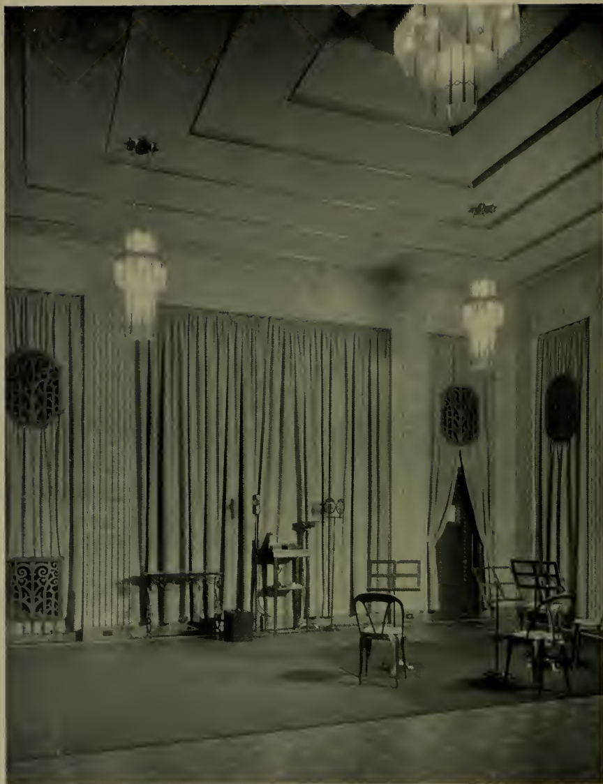
GENERAL VIEW OF STUDIO C, NATIONAL BROADCASTING COMPANY, SAN FRANCISCO
