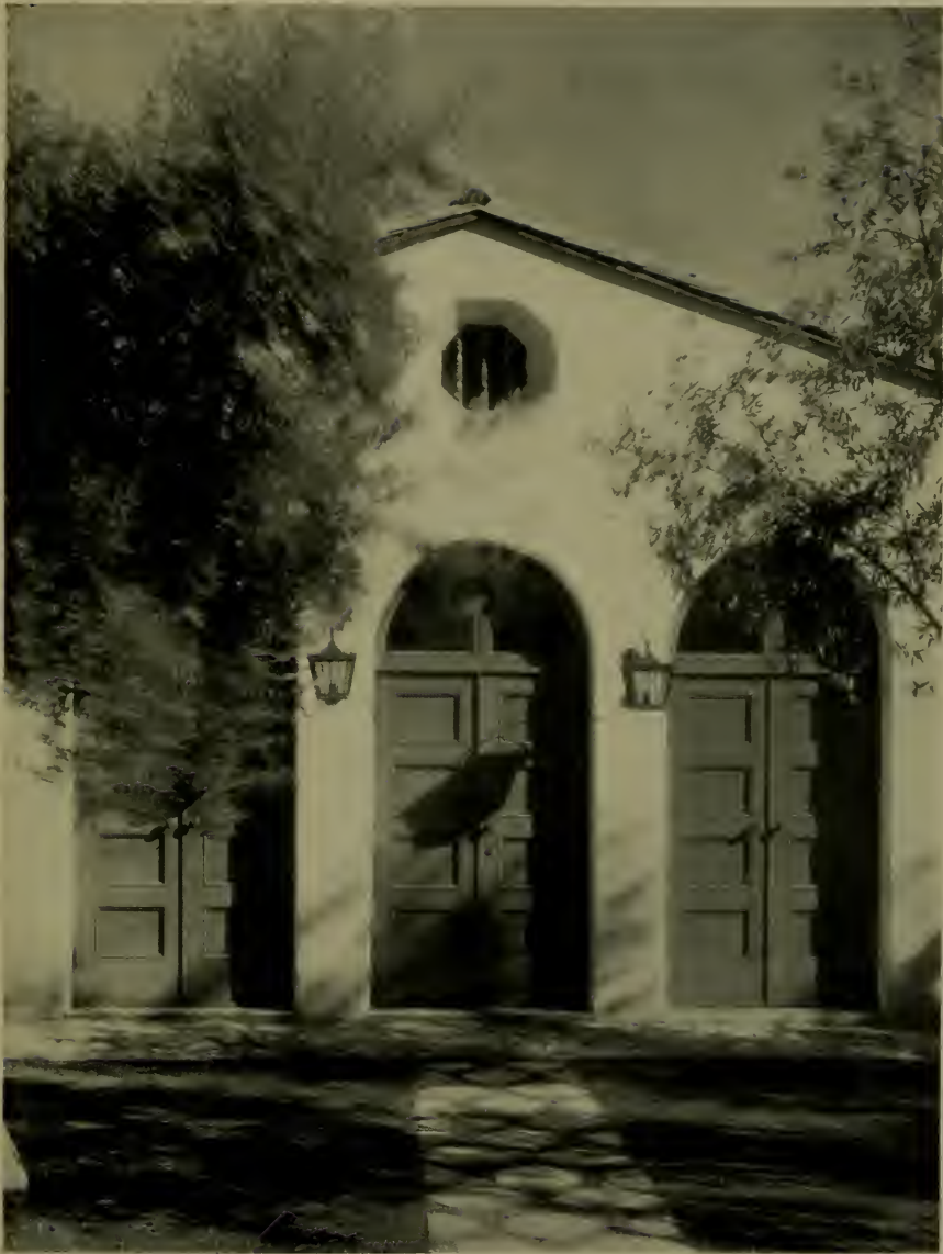
ENTRANCE, LA CANADA THURSDAY CLUB, LA CANADA, CALIFORNIA NEWTON AND MURRAY, ARCHITECTS
