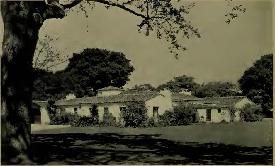
HOUSE FOR ERWIN E. RICHTER, ATHERTON, CALIFORNIA Martin J. Rist, Architect
