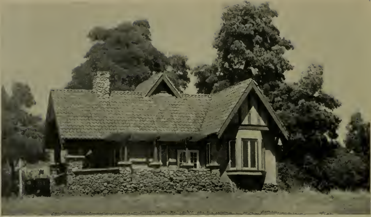
OFFICE BUILDING, EVERGREEN CEMETERY, OAKLAND, CALIFORNIA B. J. S. Cahill, Architect
