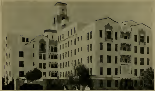
Sir Francis Drake Apartment, Los Angeles, Calif.; Consulting Architect: A. I. Rowley; Asst. Structural Eng.: Adam O. Kneeling; Contractor: Parker Construction Company
