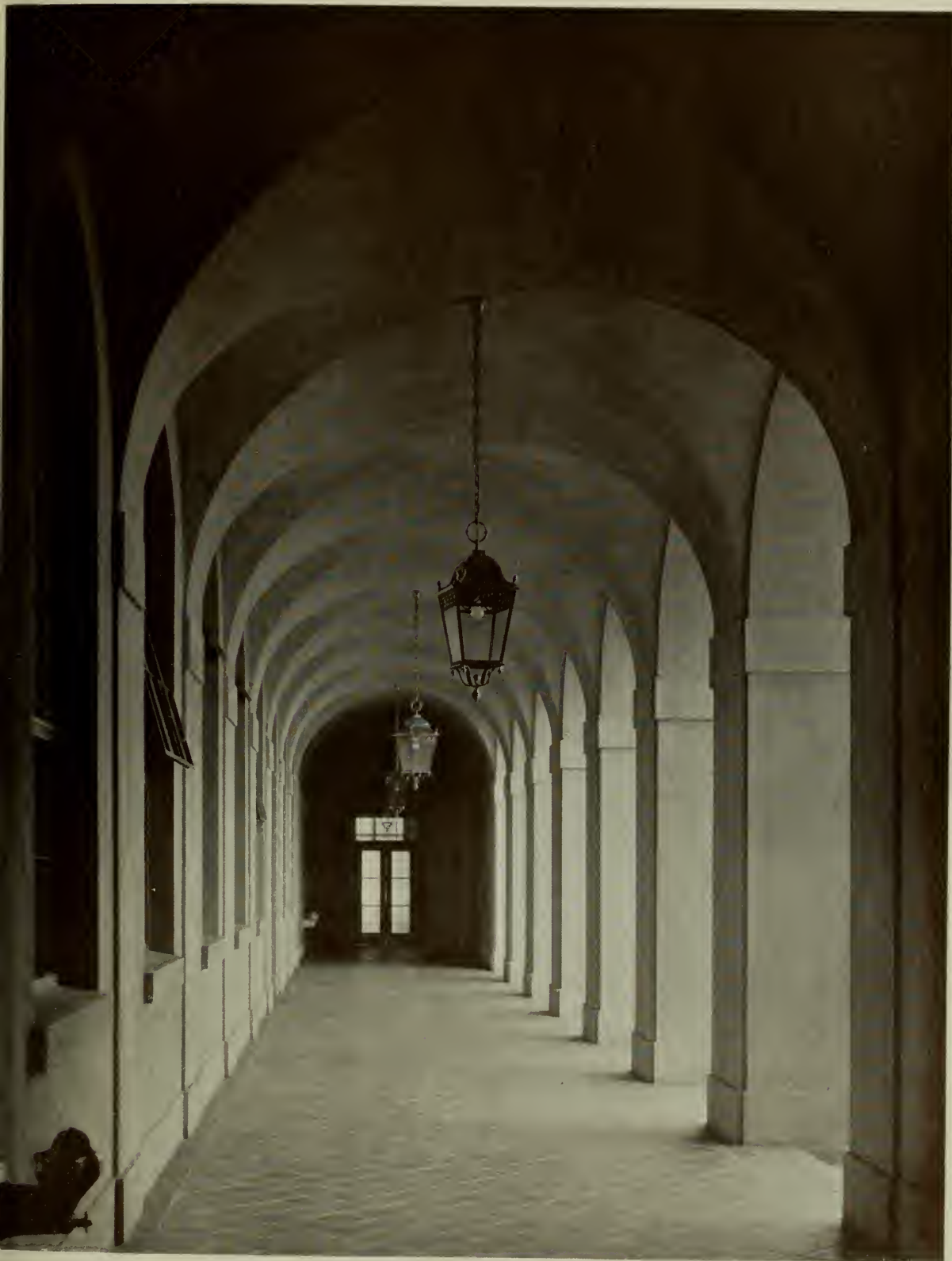
ARCADE OF PATIO, PASADENA CITY HALL, PASADENA BAKEWELL AND BROWN, ARCHITECTS
