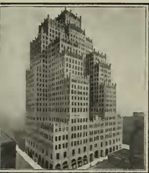
St. Louis — Bell Telephone Building
