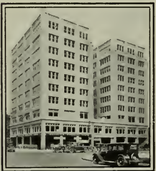
Detroit — Stephenson Building
