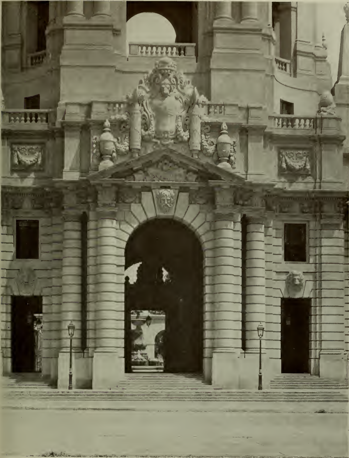
DETAIL, MAIN ENTRANCE, PASADENA CITY HALL, PASADENA BAKEWELL AND BROWN, ARCHITECTS
