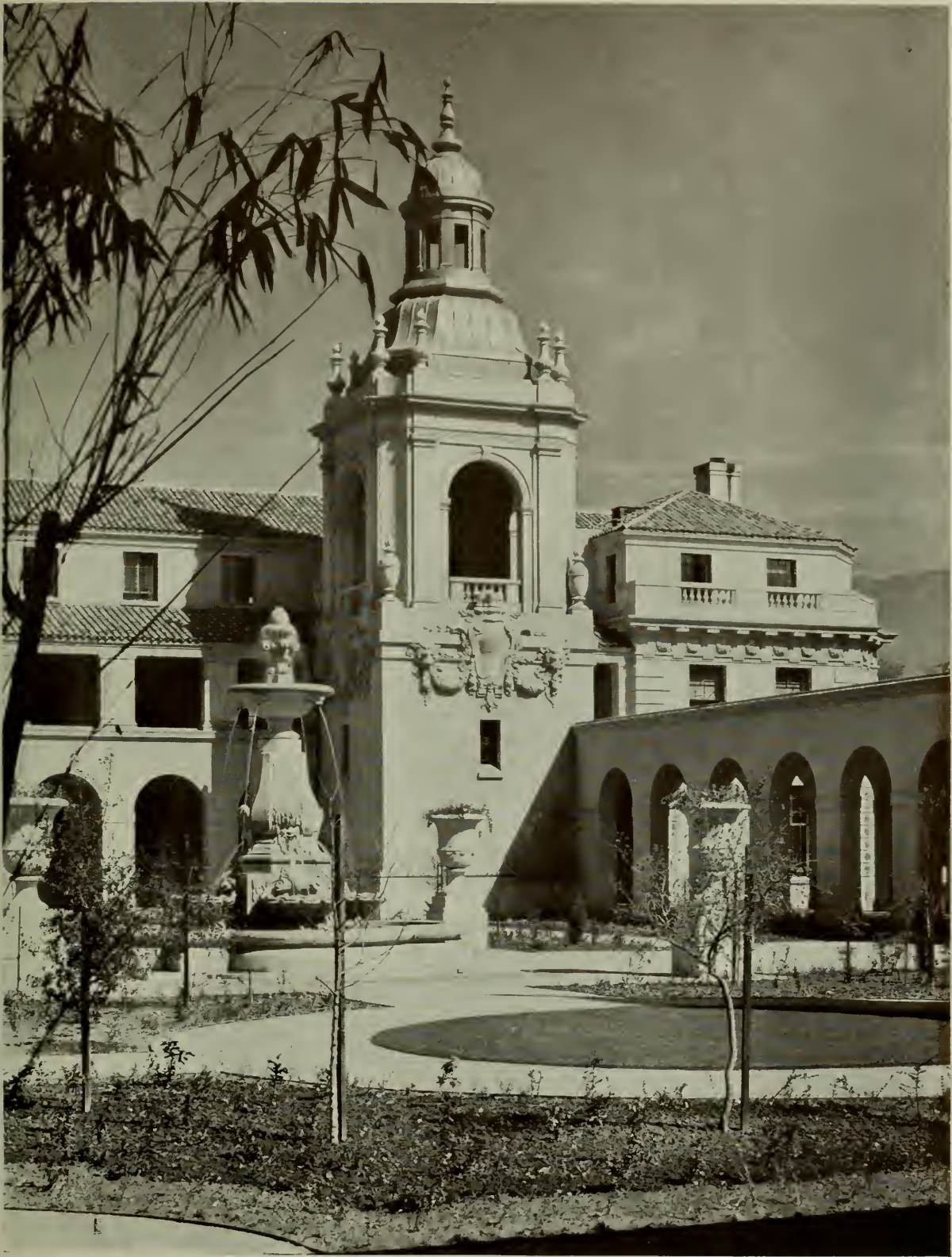
STAIR TOWER FROM PATIO, PASADENA CITY HALL, PASADENA BAKEWELL AND BROWN, ARCHITECTS
