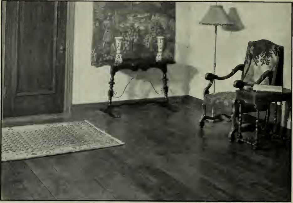
PLANK FLOORING LAID IN MASTIC
