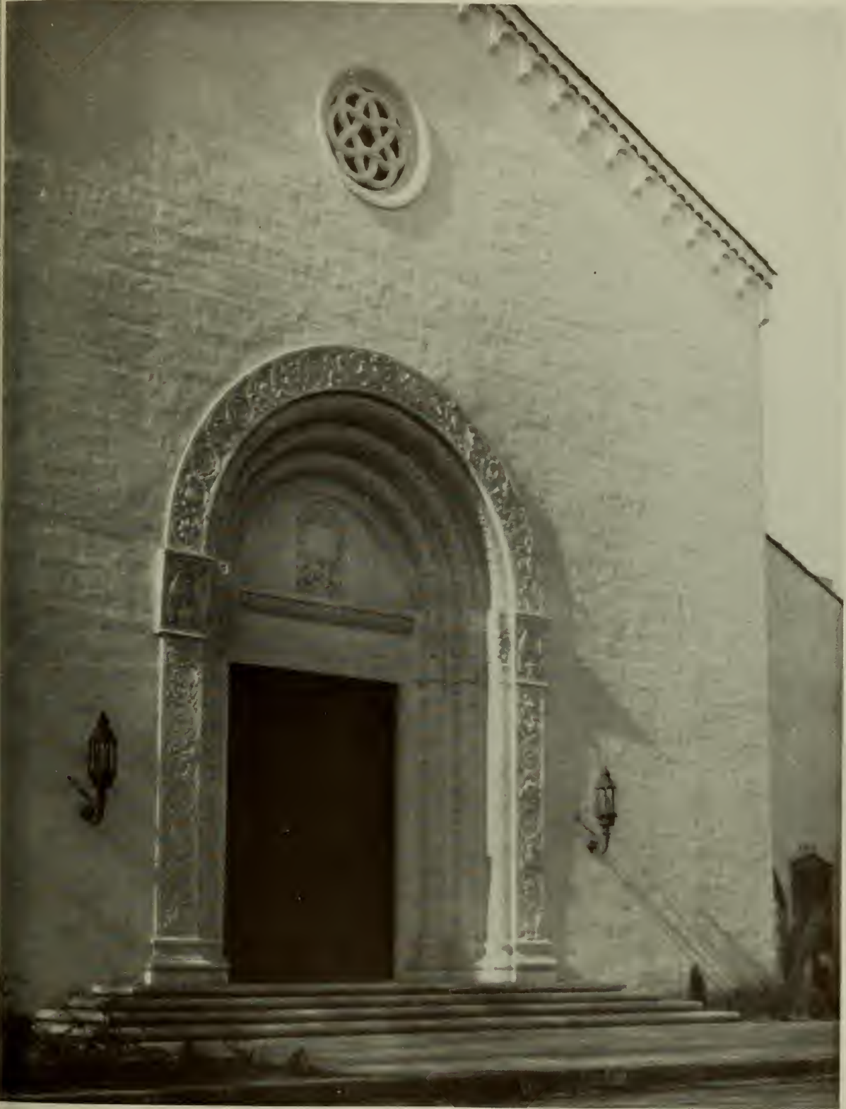
ENTRANCE DETAIL, WESTMINSTER PRESBYTERIAN CHURCH, SACRAMENTO DEAN AND DEAN, ARCHITECTS
