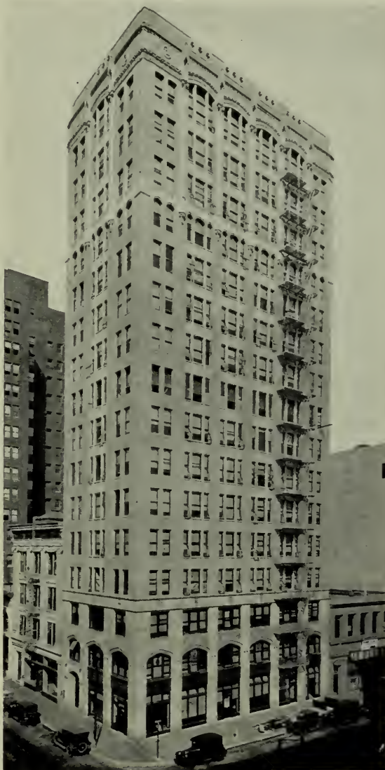
ENGINEERS' CLUB BUILDING, SAN FRANCISCO Powers and Ahnden, Architects
