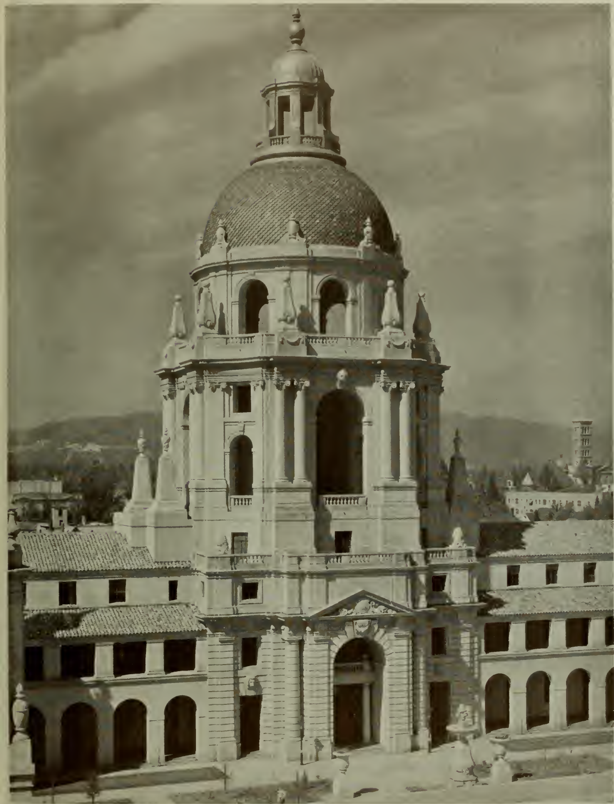
DOMES FROM PATIO, PASADENA CITY HALL, PASADENA BAKEWELL AND BROWN, ARCHITECTS
