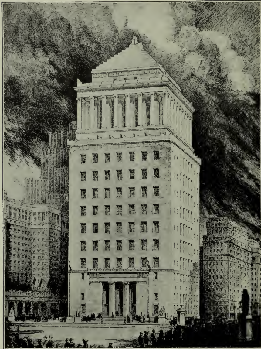
Civil Court House, St. Louis, Mo. Plaza Commission, Inc., Architects. 129,000 cubic feet Gray, 103,000 cubic feet VARIEGATED from the quarries of Indiana Limestone Company
