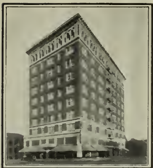
Oakland — Medical Arts Building
