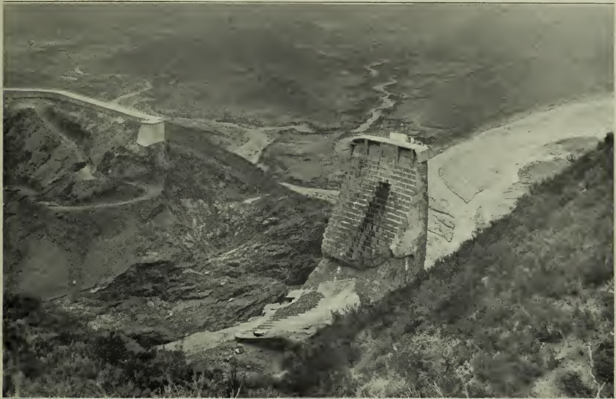
Los Angeles Examiner Photo AIRPLANE VIEW OF ST. FRANCIS DAM, LOOKING UP STREAM. FIRST BREAK APPARENTLY OCCURRED AT LEFT AS INDICATED BY TREMENDOUS HOLE SCOURED OUT OF HILLSIDE INTO WHICH WEST SIDE OF DAM WAS ANCHORED. EXTREME WEST WALL OF DAM, 600 FT. IN LENGTH, ALONG TOP OF RIDGE REMAINED INTACT. OLD CONSTRUCTION ROAD DOWN WHICH SEEPAGE FROM NEW LEAK FLOWED, IS SHOWN AT LEFT JUST BELOW BIG BLOCK OF CONCRETE
