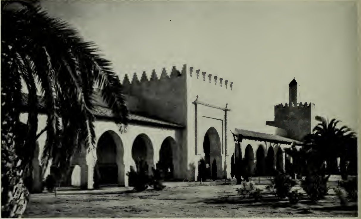
CORNER OF PATIO, PACIFIC SOUTHWEST EXPOSITION, LONG BEACH, CAL. Hugh R. Davies, Architect
