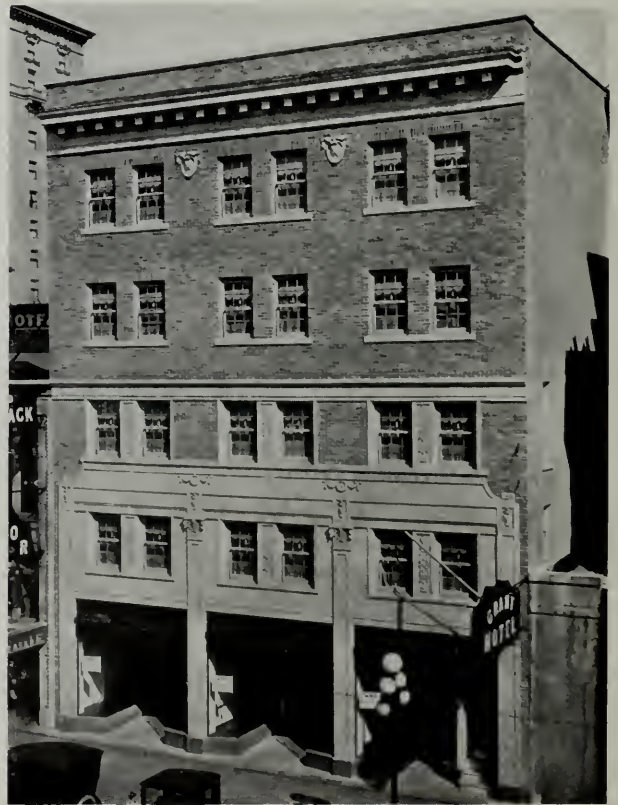
GRANT HOTEL, SEATTLE, AFTER ALTERATIONS Hancock & Lockman, Architects
