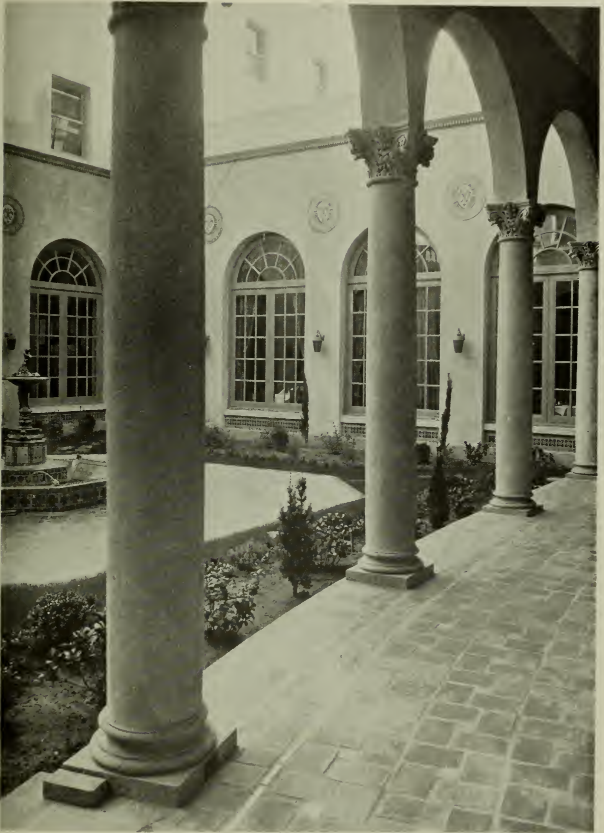
LOGGIA AND PATIO, HOTEL SAINTE CLAIRE, SAN JOSE, CALIFORNIA WEEKS AND DAY, ARCHITECTS
