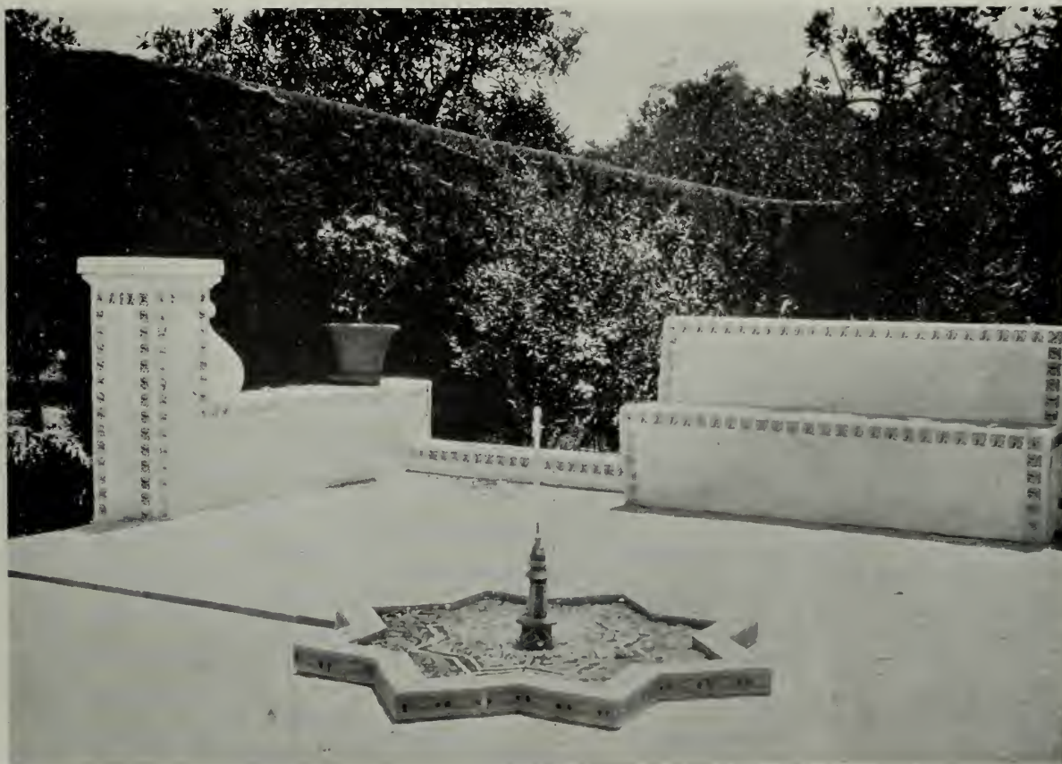
IN THIS SMALL SPANISH BASIN AND JET WE SEE HOW SIMPLY A BIT OF SPARKLING WATER MAY BE ARRANGED TO GIVE LIFE TO AN OTHERWISE PLAIN AREA. THE RUNNEL ON THE LEFT CARRIES THE OVERFLOW TO A LOWER LEVEL, WHERE THE WATER IS USED AGAIN.
