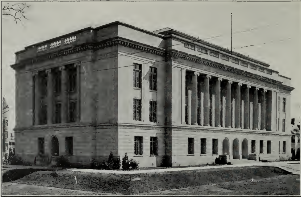
Court House, Monroe, La. J. W. Smith, Architect. Built of Gray Indiana Limestone
