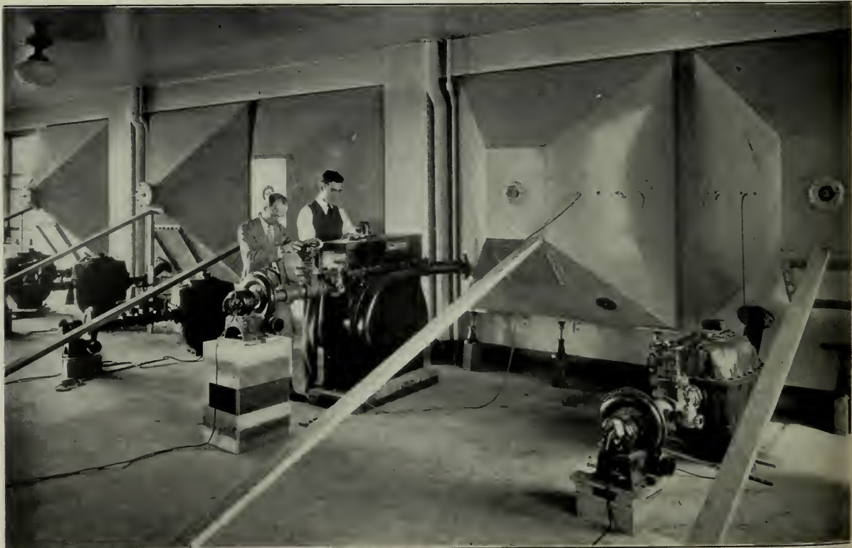
FIG. 4. SET-UP FOR TESTING WINDOW LEAKAGE IN SOUTHWESTERN BELL TELEPHONE BUILDING, ST. LOUIS, MO.
