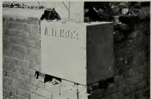
CORNER STONE SHOWS DATE CHURCH WAS ERECTED. WOOD FRAME BACK OF BRICK VENEER IN FINE STATE OF PRESERVATION
