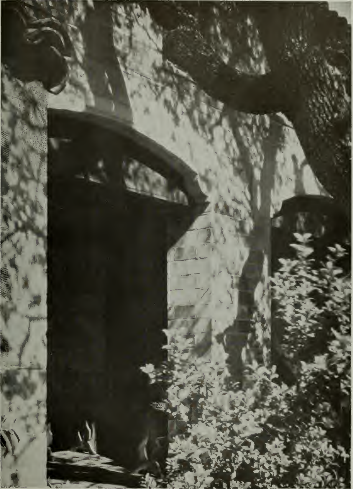
Built of Brooks Faced Tile
