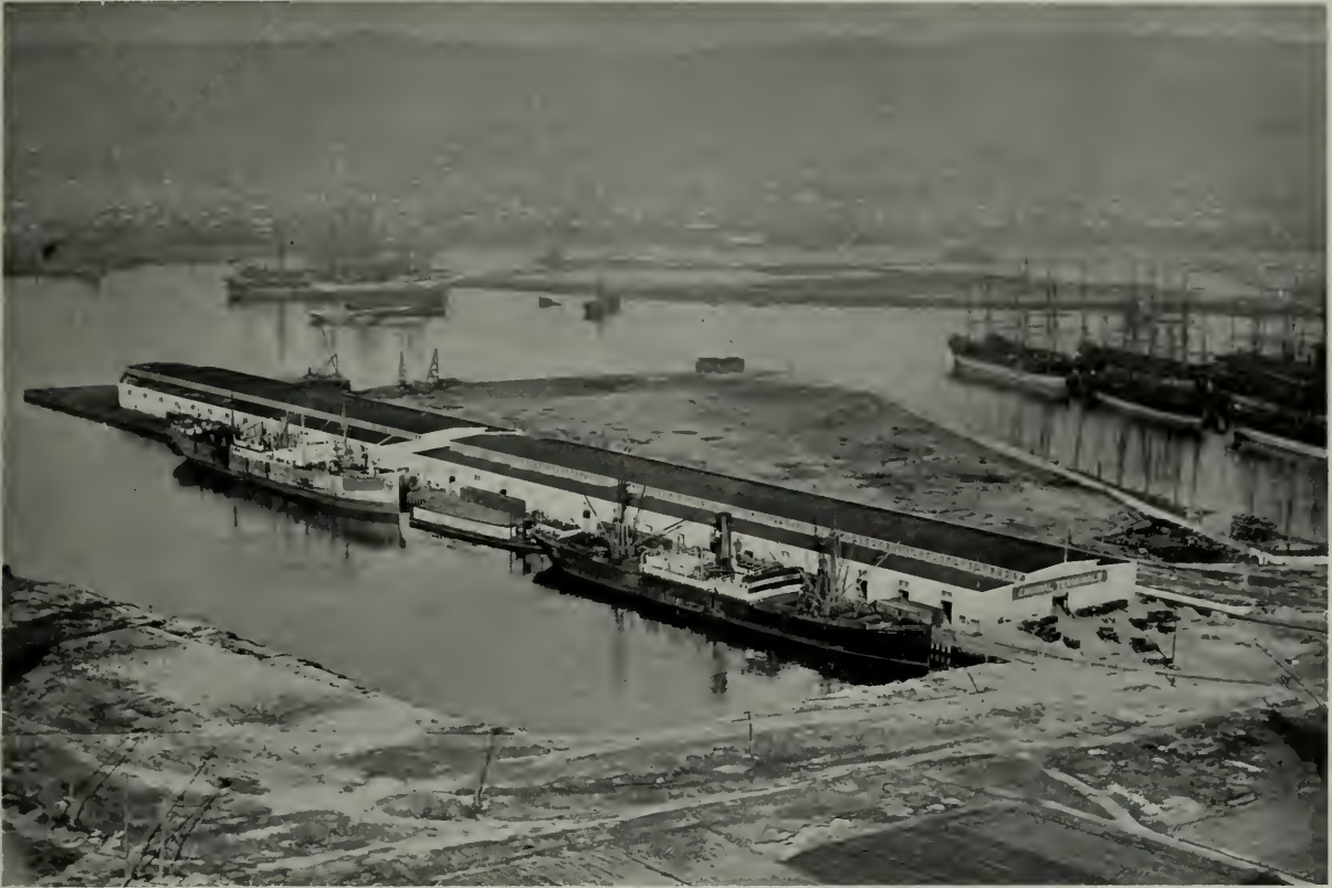
WAREHOUSES FOR ALASKA PACKERS ASSOCIATION, ALAMEDA, CALIFORNIA
