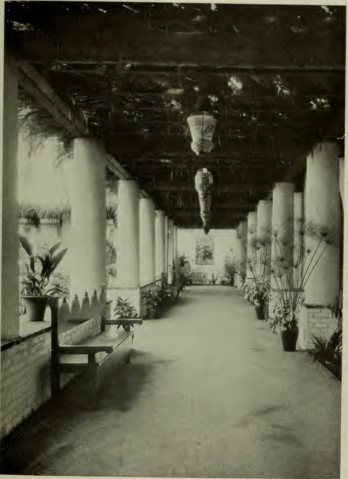
PERGOLA WALK, BILTMORE HOTEL, SANTA BARBARA, CALIFORNIA REGINALD D. JOHNSON, ARCHITECT
