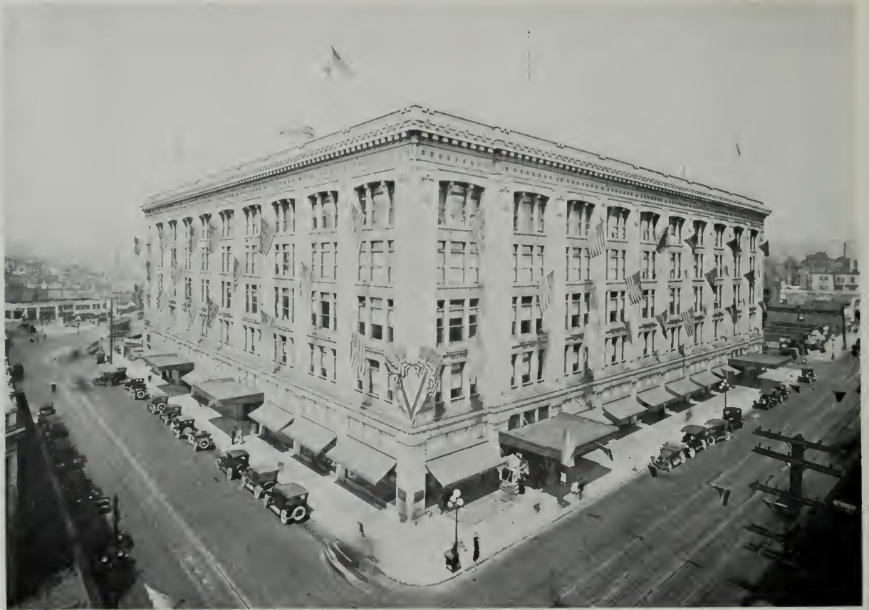
FREDERICK AND NELSON BUILDING, SEATTLE, WASHINGTON John Graham, Architect
