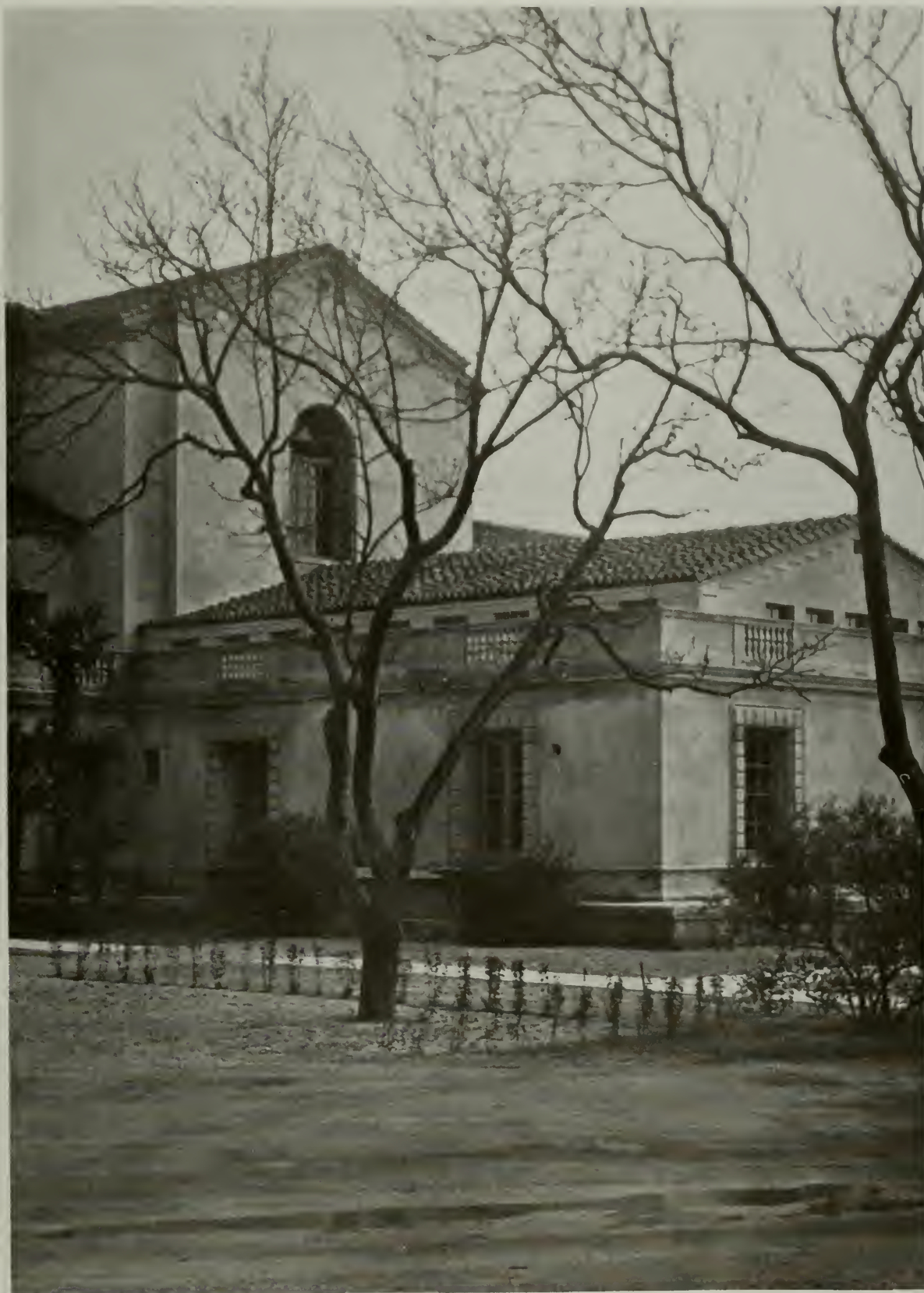
THE PASADENA PUBLIC LIBRARY BUILDING, PASADENA, CALIFORNIA MYRON HUNT AND H. C. CHAMBERS, ARCHITECTS
