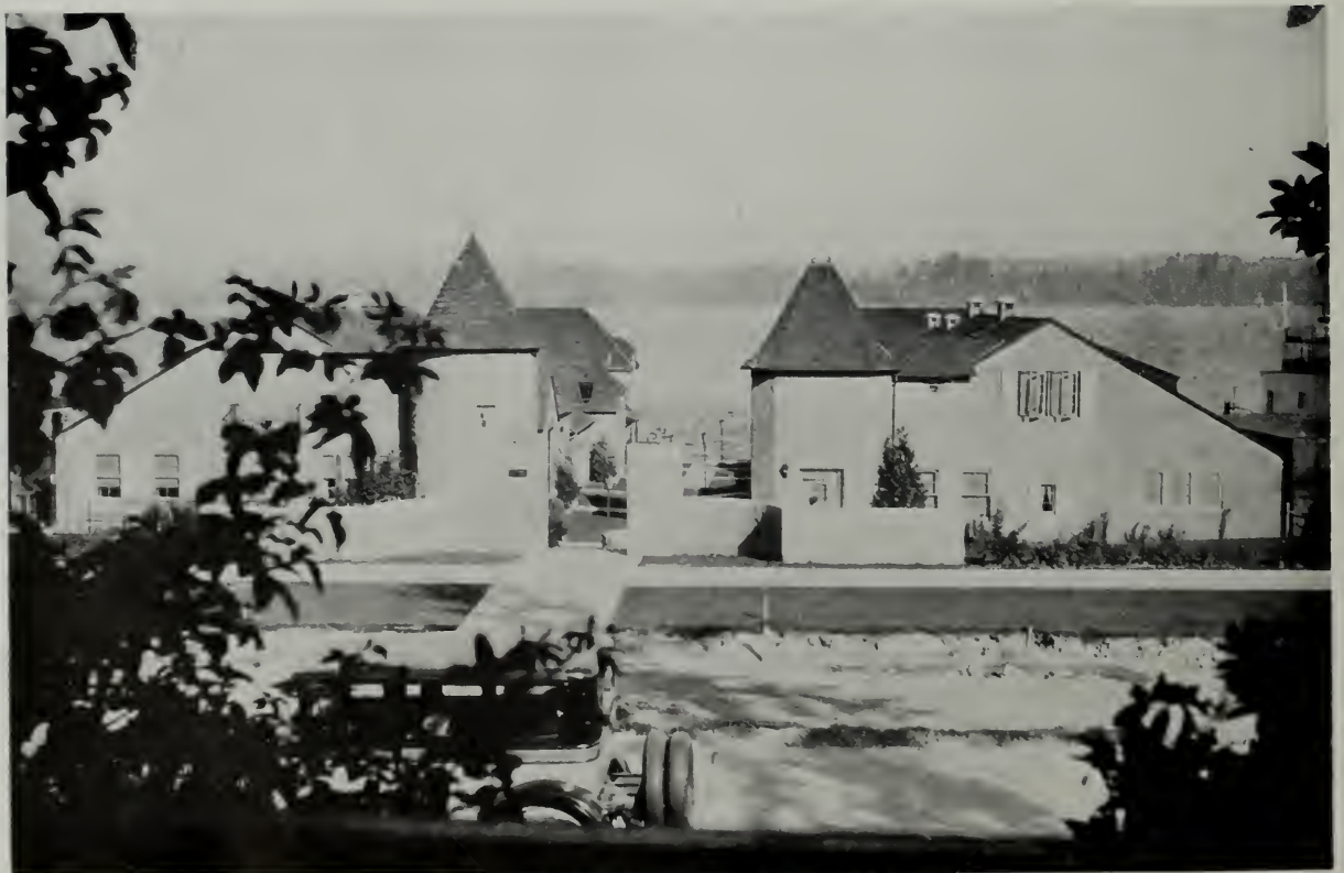
SHOREMONT APARTMENTS, SEATTLE, WASHINGTON William J. Bain, Architect
