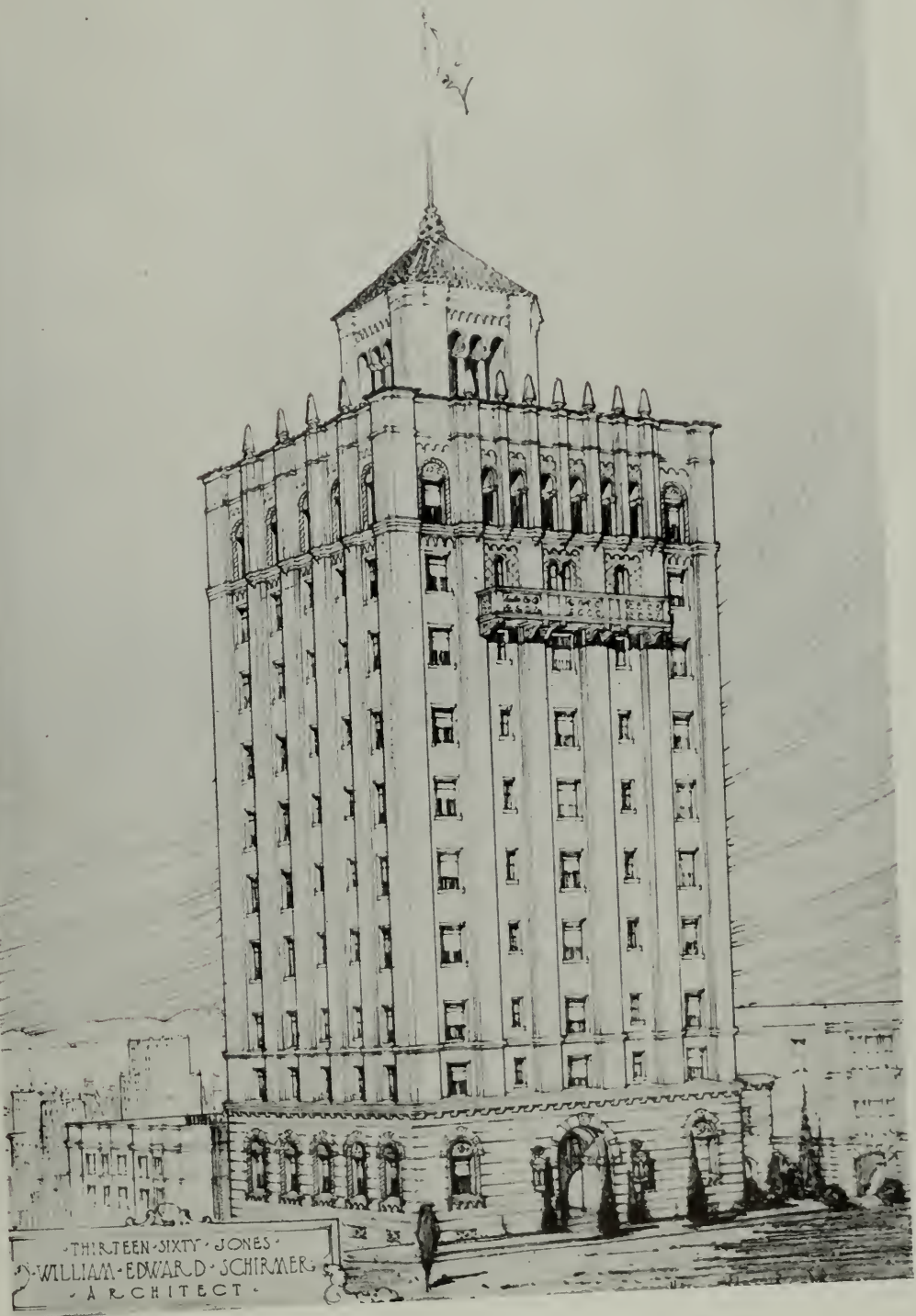
THIRTEEN SIXTY JONES APARTMENTS, SAN FRANCISCO WILLIAM EDWARD SCHIRMER, ARCHITECT
