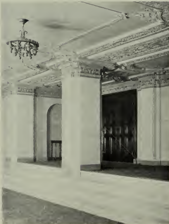
DETAIL OF FIRST STORY (UPPER) AND ENTRANCE TO BANQUET HALL, HOTEL BIGELOW, OGDEN, UTAH Leslie S. Hodgson and M. A. Mc Clenahan, Architects
