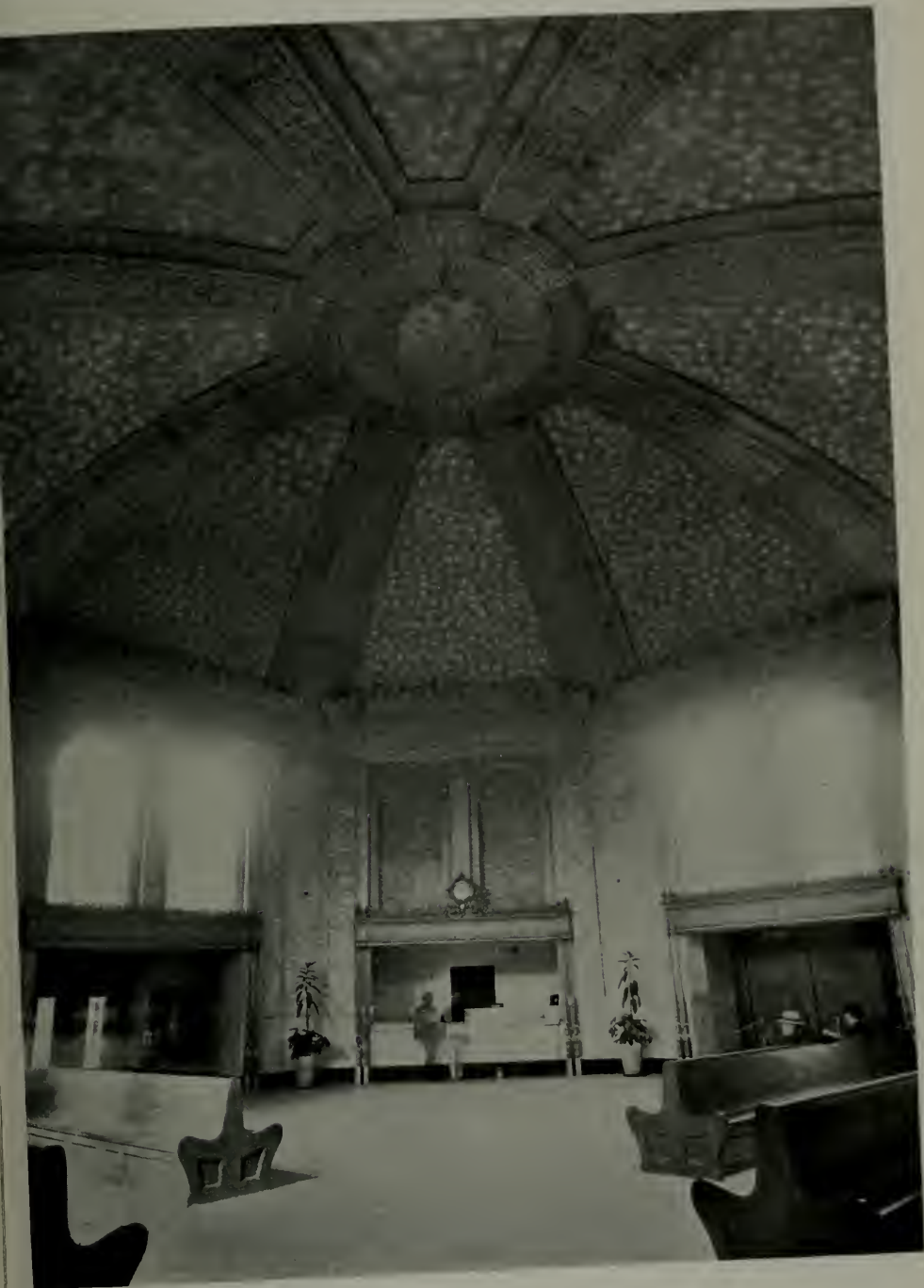
OCTAGON CEILING. UNION STAGE DEPOT, OAKLAND SWARTZ AND RYLAND, ARCHITECTS
