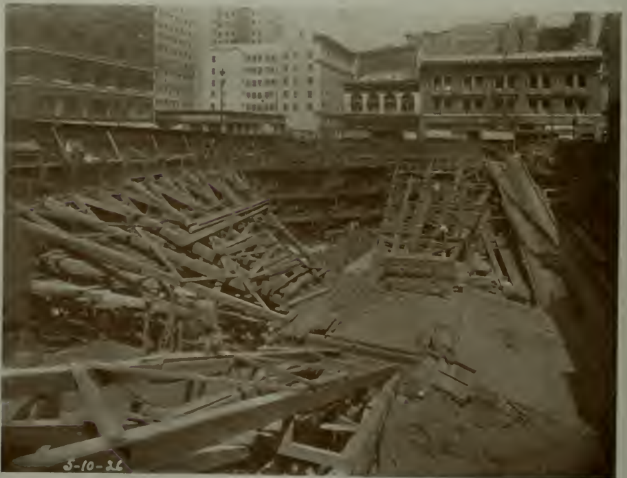
FIG II - STREET WALLS SHORED WITH HEAVY TIMBERS
