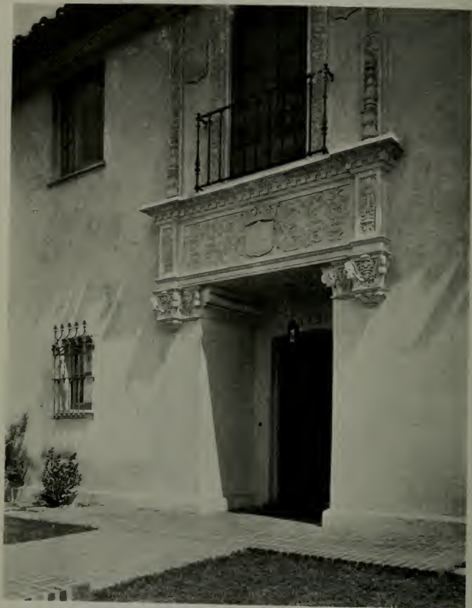
ENTRANCE DETAIL, DEL REY CLUB, BERKELEY, CALIFORNIA CHAS. F. MASTEN AND LESTER W. HURD, ARCHITECTS
