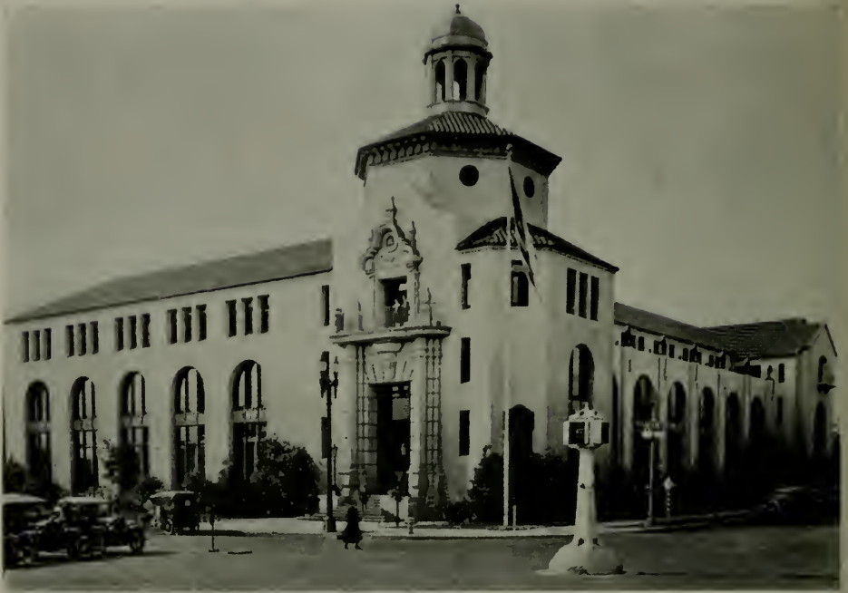
Automobile Club, Los Angeles. Construction is concrete with portland cement stucco. Filler walls are monolithic with concrete structural frame. Architects: Hunt and Burns, Los Angeles. Contractor: C. J. Kubach Co., Los Angeles.
