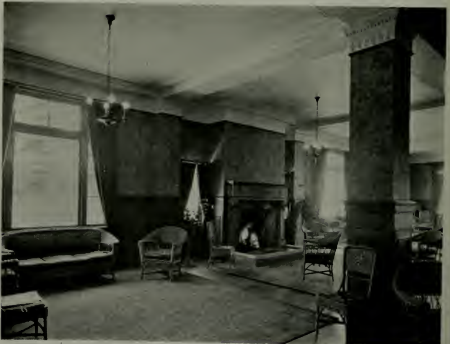
LOUNGE, FOREST HILL HOTEL, PACIFIC GROVE George Rushforth, Architect
