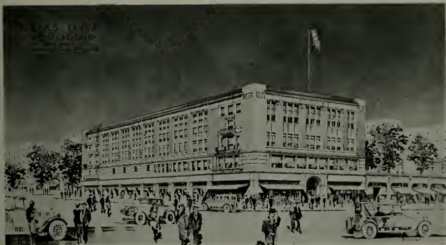
ELKS LODGE BUILDING, SANTA MONICA, CALIFORNIA
