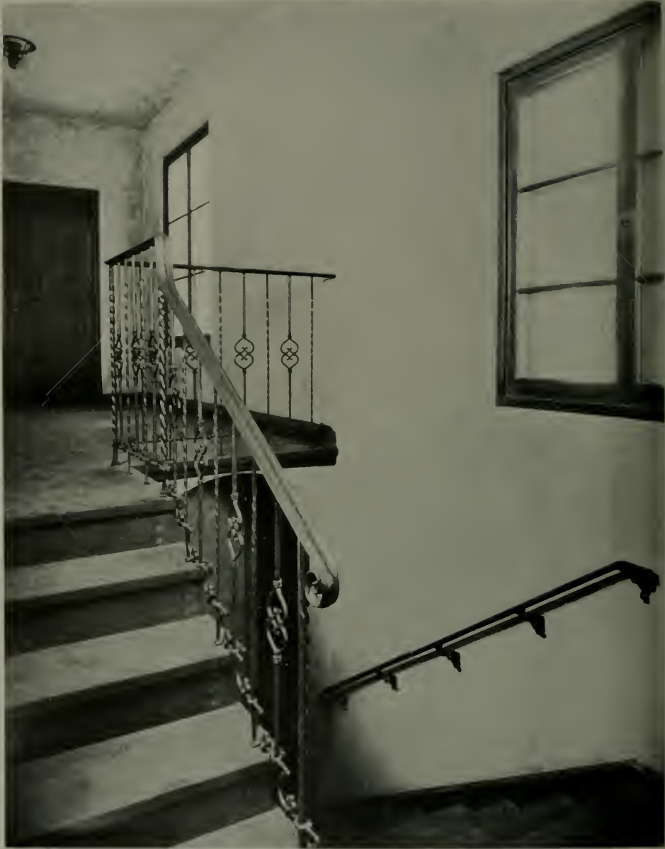
WROUGHT IRON STAIR RAIL
