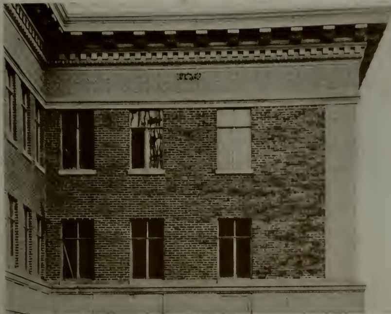
DETAIL OF CORNICE, MADE OF ARMCO SHEET METAL, BELVEDERE APARTMENTS
