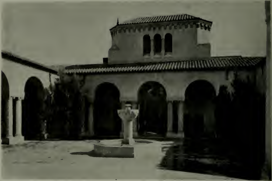
COURT, CONGREGATION EMANU-EL TEMPLE, SAN FRANCISCO S. Schnaittacher and Bakewell & Brown, Architects
