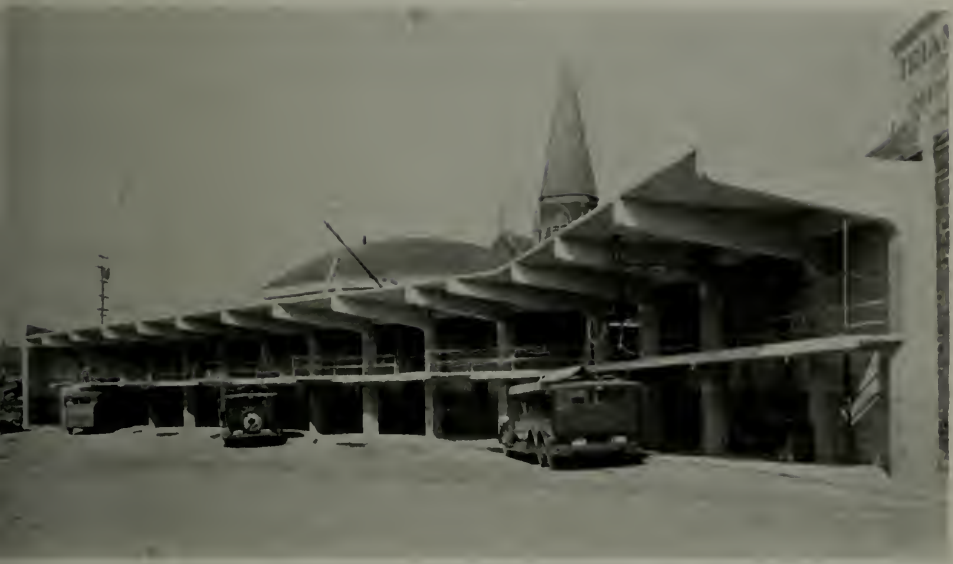
LOADING PLATFORM, AUTO STAGE DEPOT, OAKLAND Swartz and Ryland, Architects
