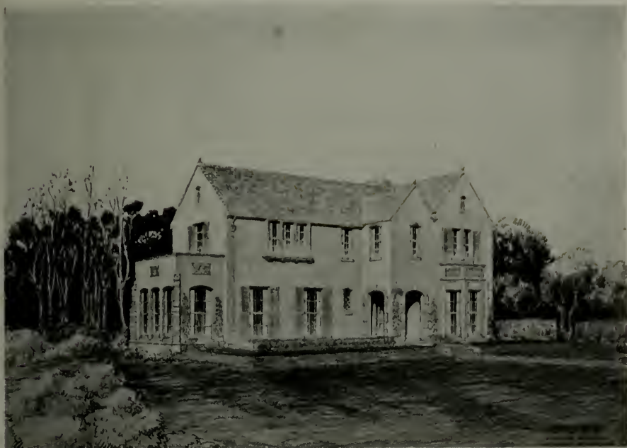
HOUSE OF FLOYD R. BEKINS, FRESNO Claude B. Barton and F. Eugene Barton, Associate Architects
