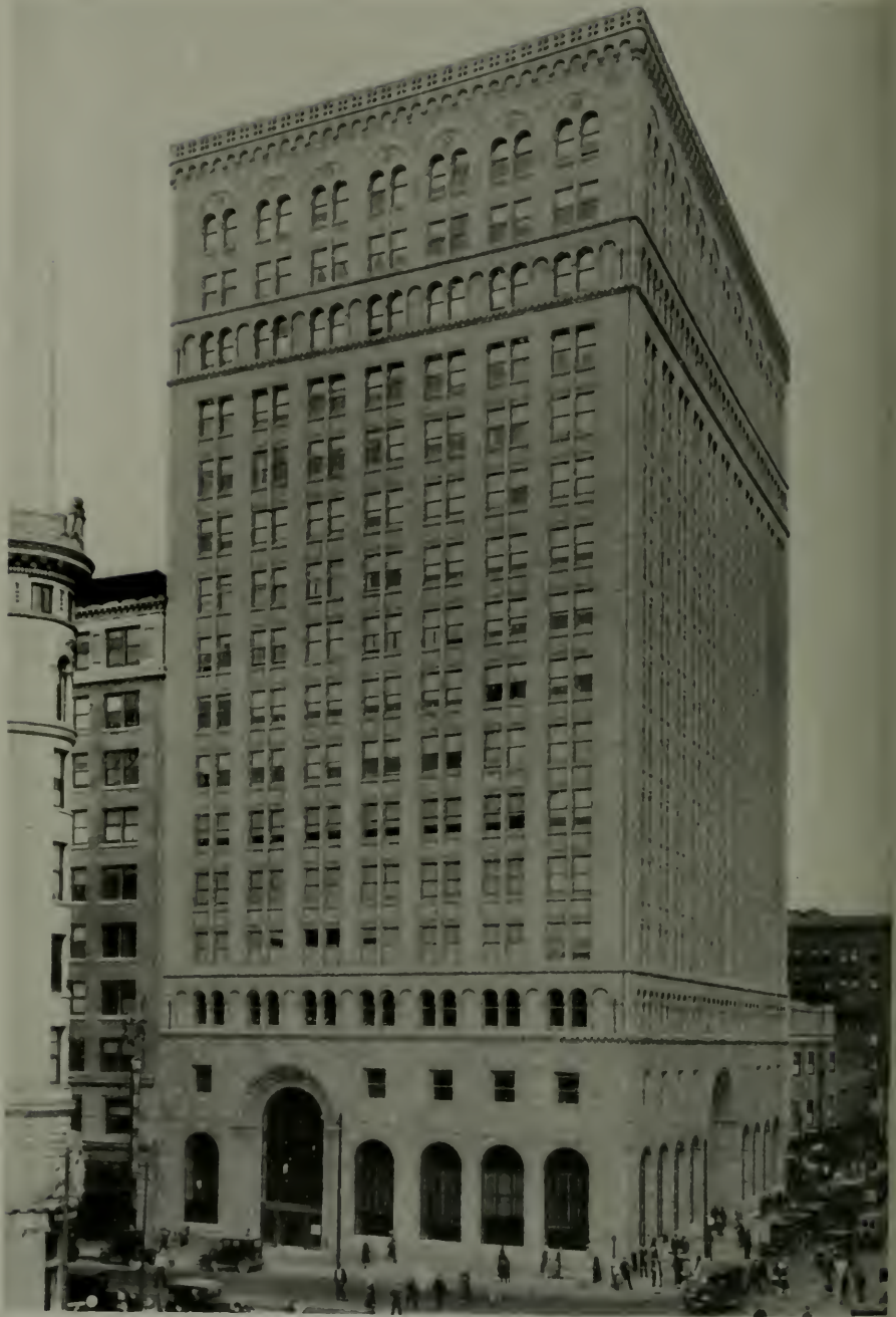
CENTRAL NATIONAL BANK BUILDING, OAKLAND GEORGE WILLIAM KELHAM, ARCHITECT
