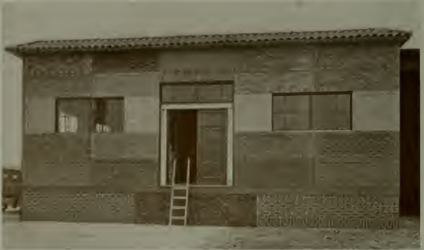
BRICK PANELED WALL. WAREHOUSE OF RICHMOND AND PORT COSTA BRICK COMPANIES, OAKLAND
