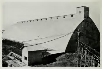
SEED HOUSE FOR THE SAN DIEGO OIL PRODUCTS COMPANY Over 32,475 pounds of 26 gauge Armco Ingot Iron used for roof and sides
