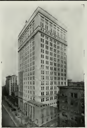
Federal Reserve Bank of Kansas City, Mo. Graham, Anderson, Probst & White, Architects
