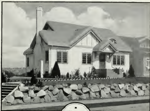
Gordner J. Gwinn Home, Seattle. Medusa Stainless White Cement used in the stucco.
