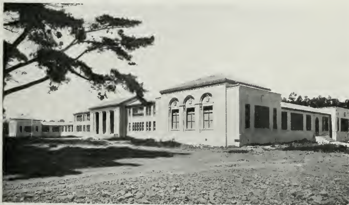
Showing type of High School in which acid-proof drain line is a necessity for permanency. Burlingame High School, San Mateo district. W. H. Weeks, Architect
