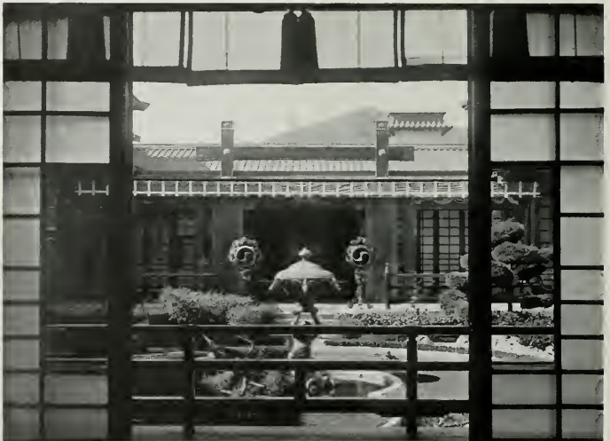
PATIO, HOUSE OF MESSRS. ADOLPH AND EUGENE BERNHEIMER HOLLYWOOD, CALIFORNIA
