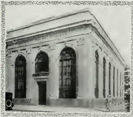
Seacost Trust Co., Asbury Park, N. J. T. M. James, Architect. Bath Limestone on granite base.
