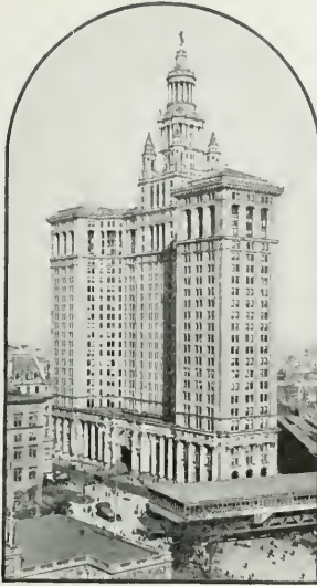
MUNICIPAL BUILDING NEW YORK CITY
