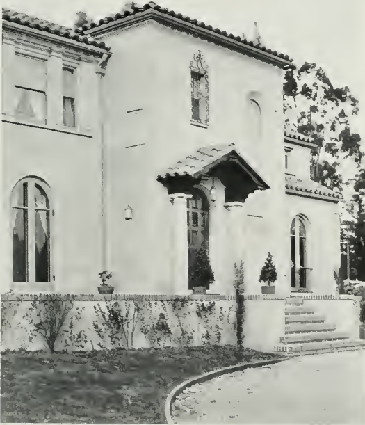
HOUSE FOR MR. CARL H. BEAL, SAN MATEO Charles K. Branner, Architect
