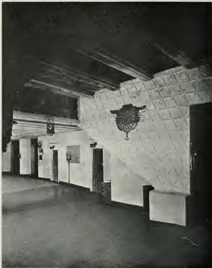
Concrete cast in place, both ornamental and structural
