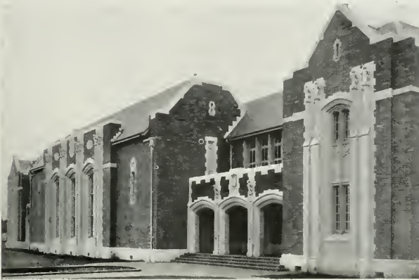
JOHN L. SHEARER GRAMMAR SCHOOL, NAPA, CALIFORNIA Built of Concrete Walls and Veneered with Cannon Face Brick for Beauty
