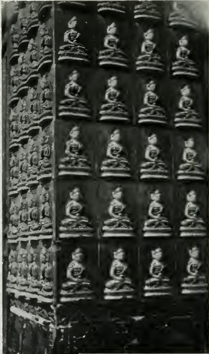
EXTERIOR WALL OF SHRINE, WINTER PALACE, PEKIN Green Glazed Terra Cotta Tile
