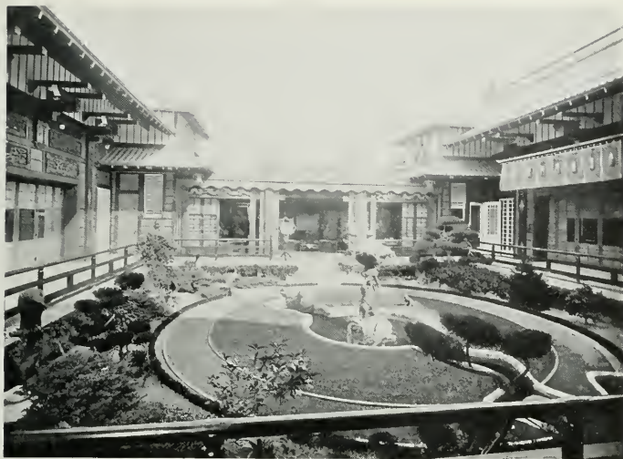
PATIO, HOUSE OF MESSRS. ADOLPH AND EUGENE BERNHEIMER HOLLYWOOD, CALIFORNIA
