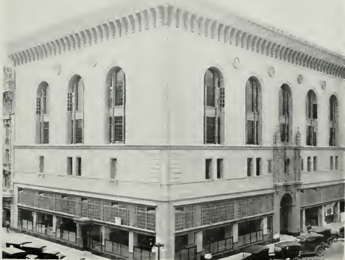
MASONIC TEMPLE, STOCKTON, CALIFORNIA Carl Werner, Architect
