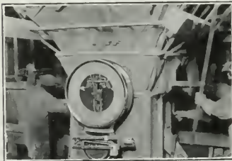
WEIGHING THE CEMENT AND STONE ON A TOLEDO SCALE
