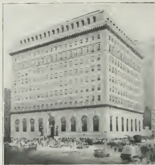
Federal Reserve Bank Building, Cleveland, Ohio Walker and Weeks, Cleveland, Architects L. K. Comstock, Cleveland, Electrical Contractors
