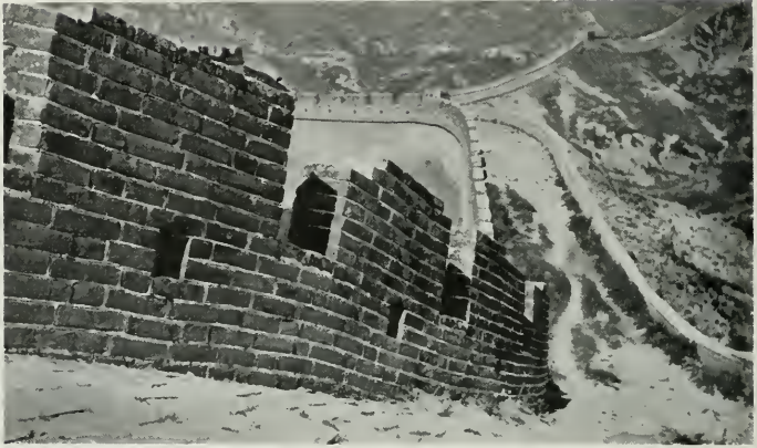
GREAT WALL OF CHINA. GRAY BRICK, ABOUT 3 IN. x 7 IN. x 15 IN. Steps in foreground in gray tile
