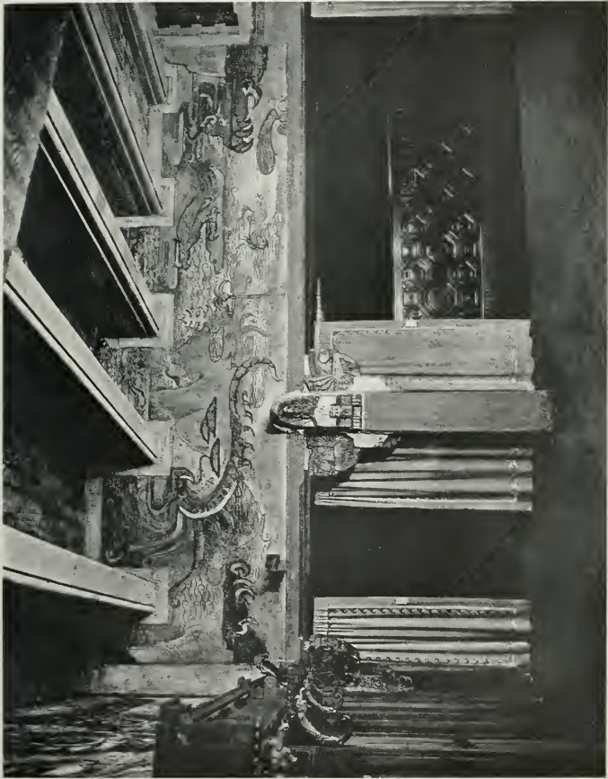
Murals done on rough concrete. Ornaments on columns are of concrete cast in place.
