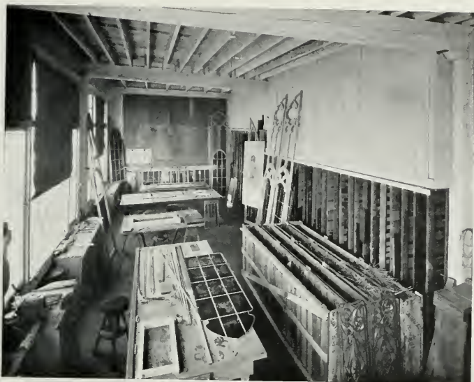
LEADED GLASS MANUFACTORY, FULLER & GOEPP BUILDING, OAKLAND
