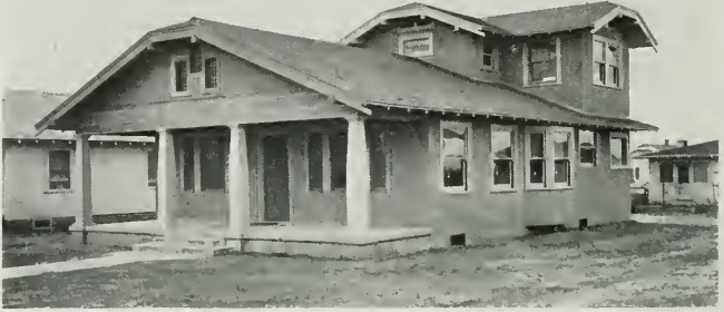
ELECTRICALLY EQUIPPED BUNGALOW, FRESNO Note Absence of Chimney
