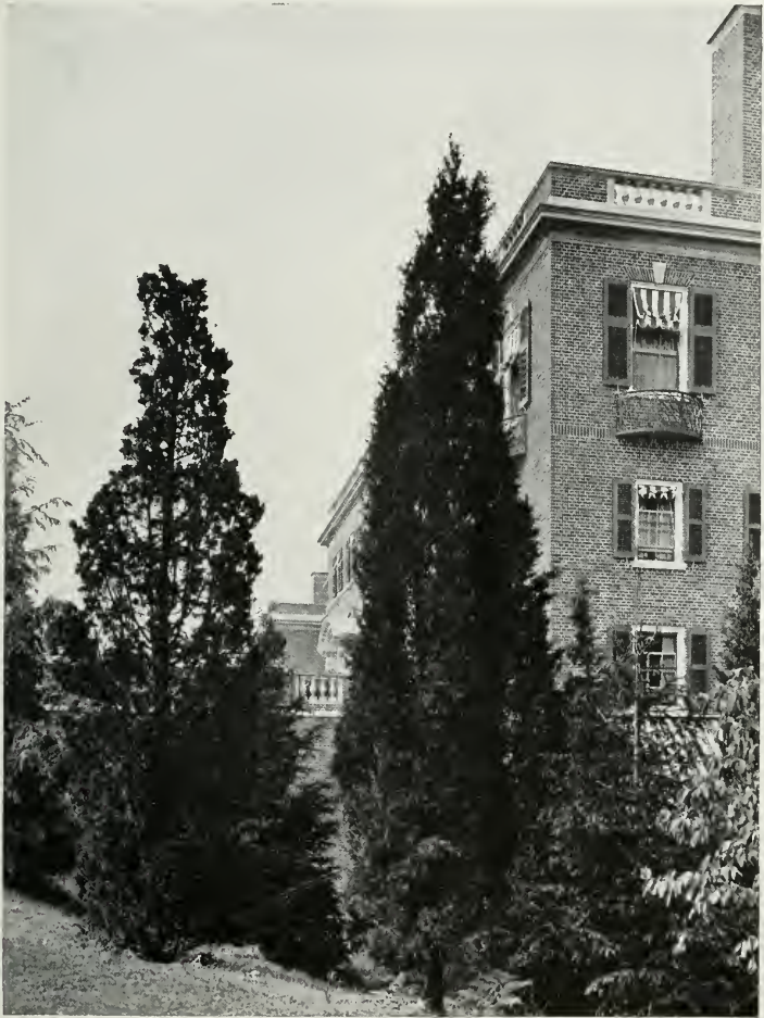
Residence of C. K. G. Billings, Esq., Locust Valley, N.Y. Gray Lowell, Architect
