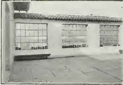
Steel Sash on the Roof Garden
