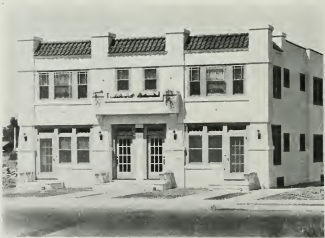
ELECTRICALLY EQUIPPED APARTMENT HOUSE, FRESNO Nels N. Nelsen, Designer and Builder
