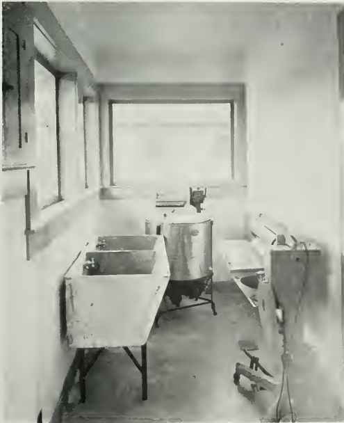
PORCH OF FRESNO APARTMENT HOUSE Electrical Equipment includes Washing Machine and Ironer
