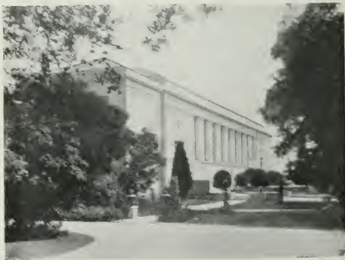
HUNTINGTON LIBRARY AT SAN MARINO Myron Hunt and H. C. Chambers, Architects Awarded Certificate of Honor for Semi-Public and Cultural Buildings, Class "B"
