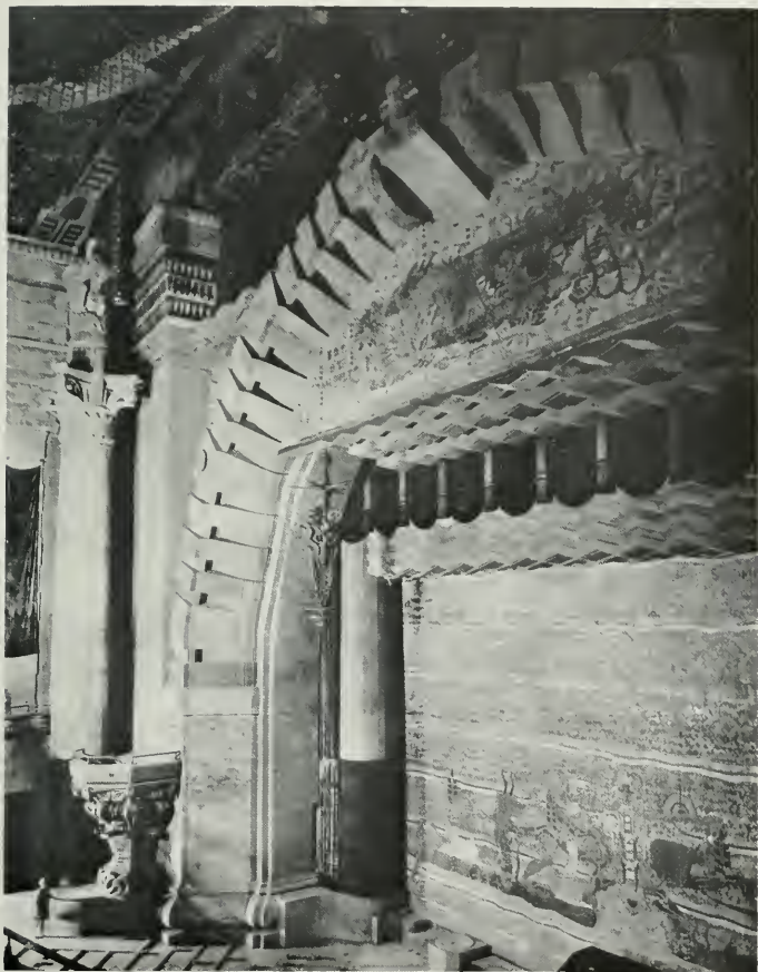
Note open trusses, beam decorated by mural in the support of organ grille
