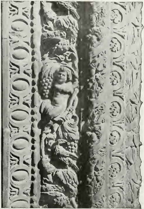
DETAIL of terra cotta window architraves, exterior of Ospedale Maggiore, Milan, Italy, erected 1456 A. D. and still standing. (Reproduced from "Color in Architecture," published by the National Terra Cotta Society.)
