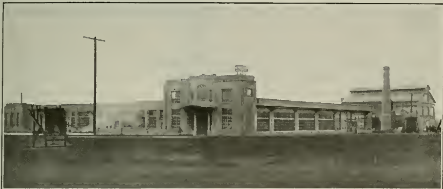
PLANT OF COAST TIRE AND RUBBER COMPANY, OAKLAND Designed by L. L. SMITH, C. E. FOUNDATION COMPANY, Builders
