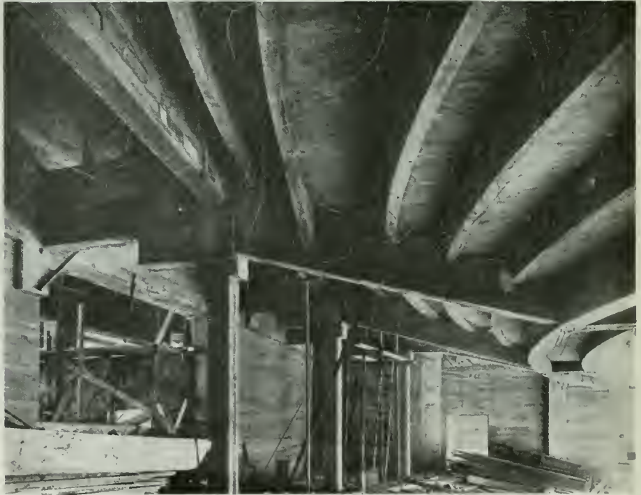
CONSTRUCTION PHOTOGRAPHS, MOROSCO THEATRE, LOS ANGELES, MORGAN, WALLS & MORGAN, ARCHITECTS
