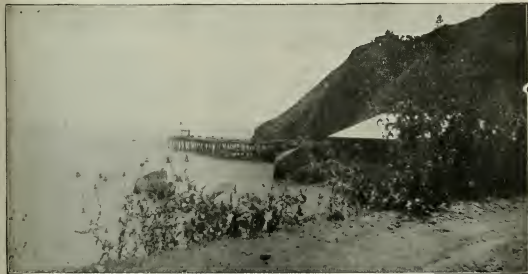
Fig. 4—Wharf recently erected at Port Orford. The piles are protected from marine borers by corrugated iron pipes.
