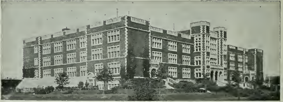
CENTRAL HIGH SCHOOL, MINNEAPOLIS, MINN.
