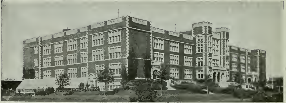
CENTRAL HIGH SCHOOL, MINNEAPOLIS, MINN.
