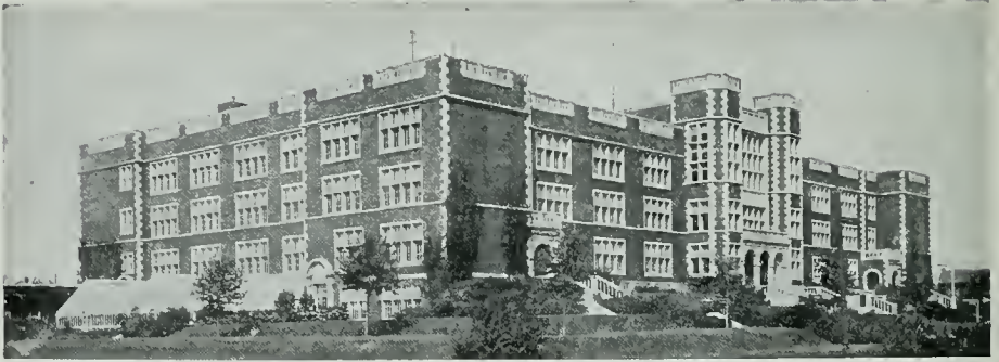
CENTRAL HIGH SCHOOL, MINNEAPOLIS, MINN.
