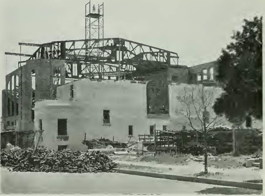
PROGRESS VIEW OF CHURCH AT LONG BEACH, CALIFORNIA, BEFORE COLLAPSE OF STEEL TRUSSES
