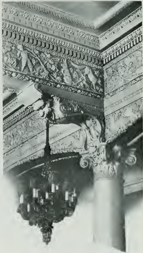
A CORNER OF THE DINING ROOM, HOTEL DAVENPORT, SPOKANE, WASH. Cutter & Malmgren, Architects
