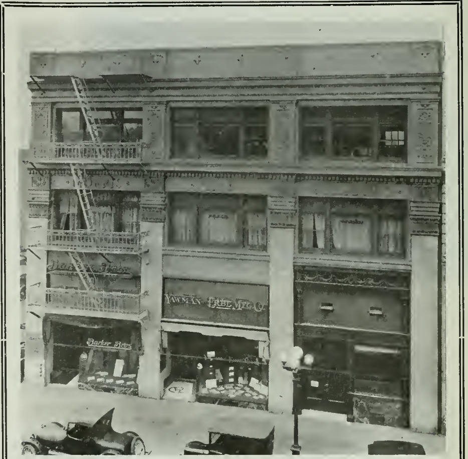
MORRIS PLAN BANK BUILDING, LOS ANGELES Morgan, Walls & Morgan, Architects
