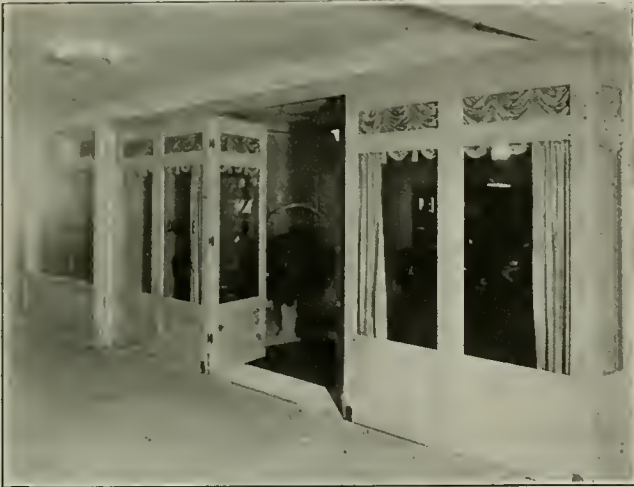
Note pair of doors and return end of partition.
