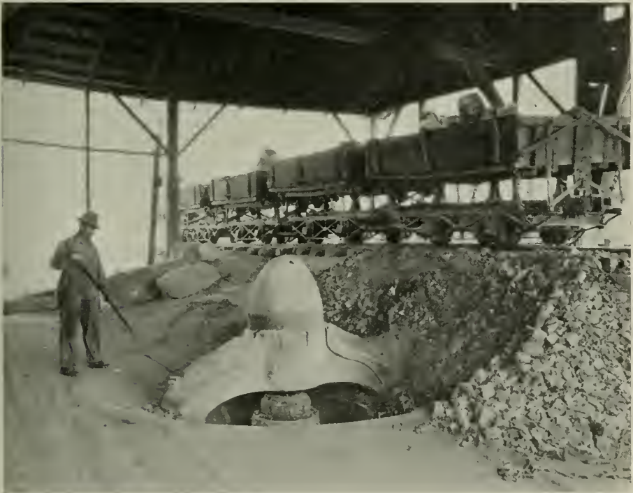
PIEDRA ROCK COMPANY'S PLANT Gyratory crusher into which a carload of rock is dumped and quickly reduced to crushed stone.
