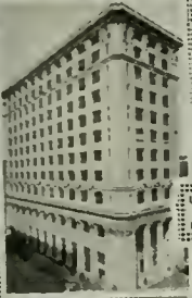
LOS ANGELES TRUST AND SAVINGS BLDG. LOS ANGELES CAL.
