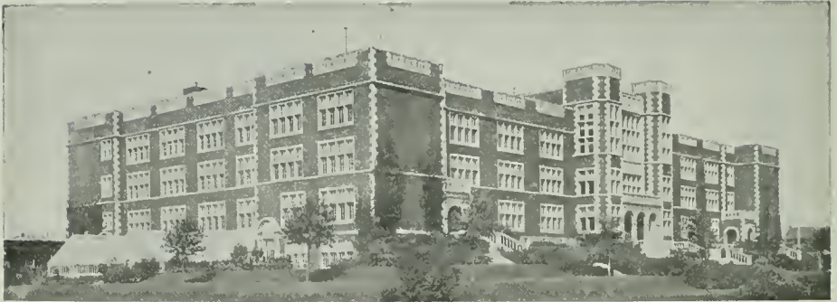
CENTRAL HIGH SCHOOL, MINNEAPOLIS, MINN.
