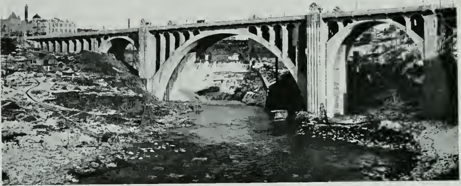
MONROE STREET BRIDGE, SPOKANE, WASH. J. C. Ralston, Engineer; Kirtland Cutter, Architect
