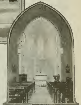
The interior is done in quartered oak; Caen stone walls with Artstone trimming. Aisle and vestibule floors of Faence tile; Chancel floor of Grey Tennessee Marble. The altar is of White Vermont Marble.
