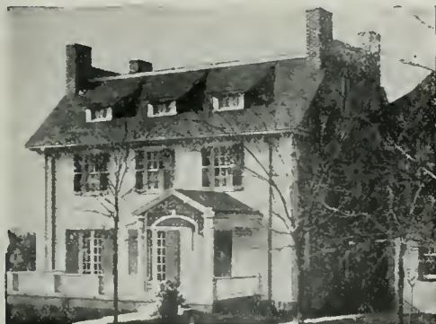
Walls finished with Cabot's Old Virginia White Roof finished with No. 3 1/2 Dark Gray Creosote Stain Walter Boschen, Architect, St. Joseph, Mo.
