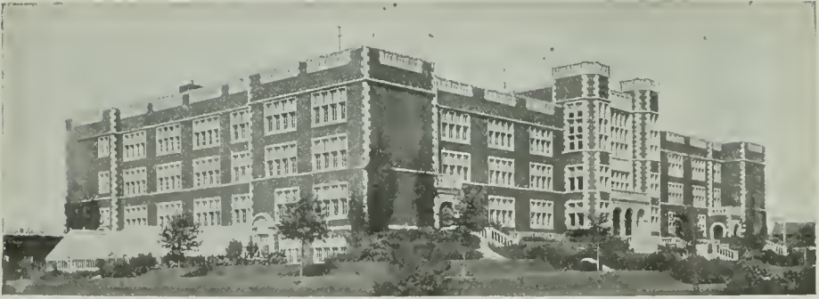
CENTRAL HIGH SCHOOL, MINNEAPOLIS, MINN.
