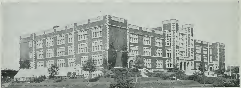
CENTRAL HIGH SCHOOL, MINNEAPOLIS, MINN.
