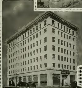
CITIZENS SAVINGS BLDG. PASADENA, CAL.
