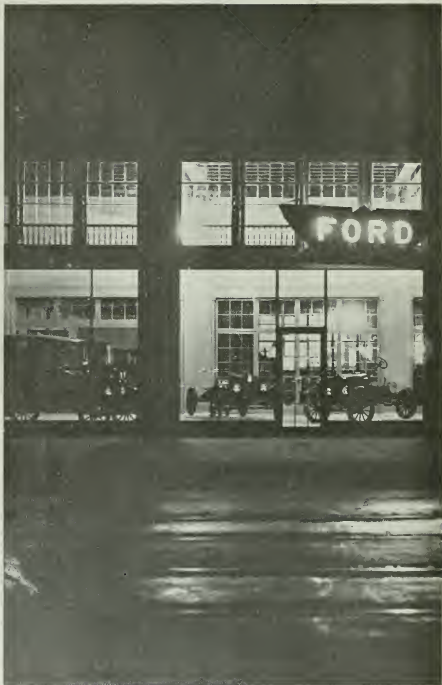
GARAGE FOR F. D. NAYLOR, STOCKTON, CALIFORNIA CHARLES W. McCALL, ARCHITECT
