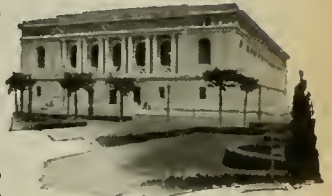
Carnegie Library San Francisco; all sheet metal and iron grills on windows are of Armco Ingot Iron. Geo. W. Kelham, Architect.
