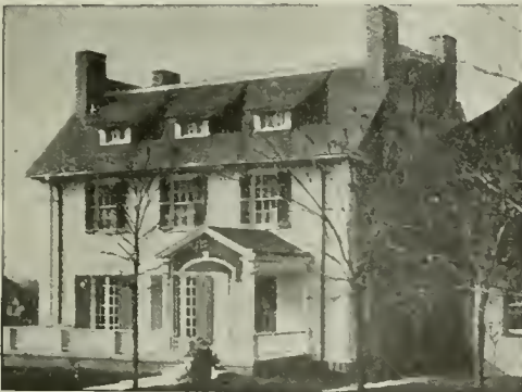
Walls finished with Cabot's Old Virginia White Roof finished with No. 36 Dark Gray Creosote Stain Walter Boschen, Architect, St. Joseph, Mo.
