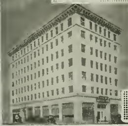
CITIZENS SAVINGS BLDG. PASADENA, CAL.
