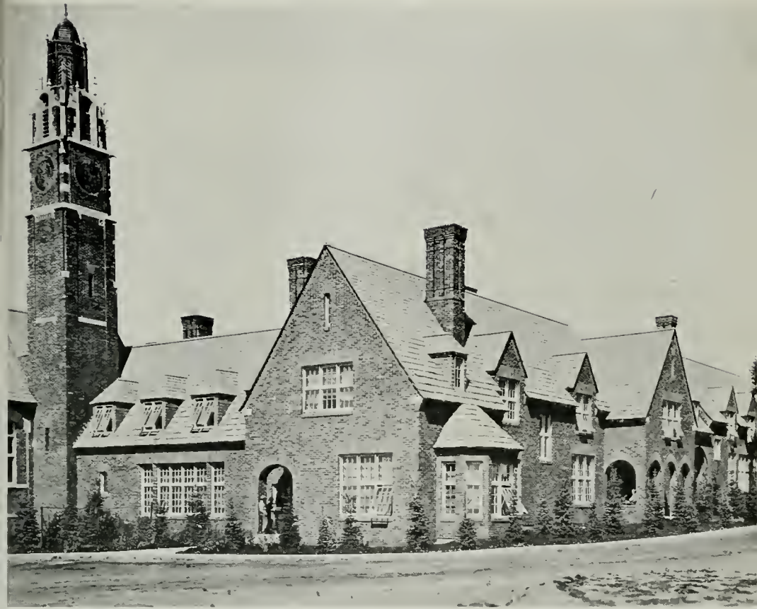
OFFICE AND TOWER, THE ADMINISTRATIVE BLDG., HUTTON SETTLEMENT, SPOKANE, WAS WHITEHOUSE & PRICE, ARCHITECTS
