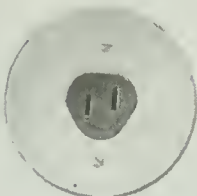
The finished ceiling Elexit
