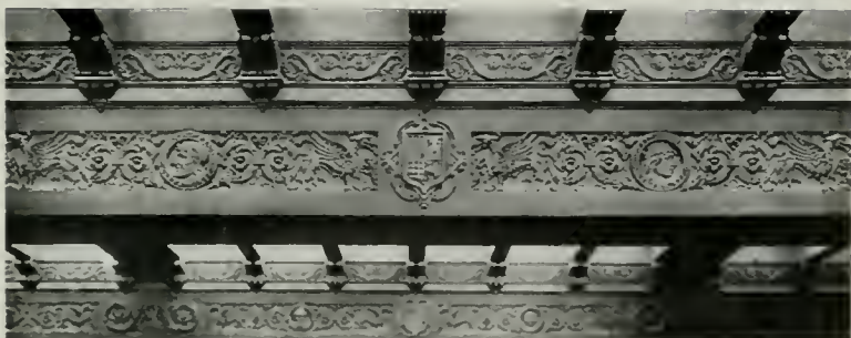
DETAIL OF CEILING IN LOBBY
