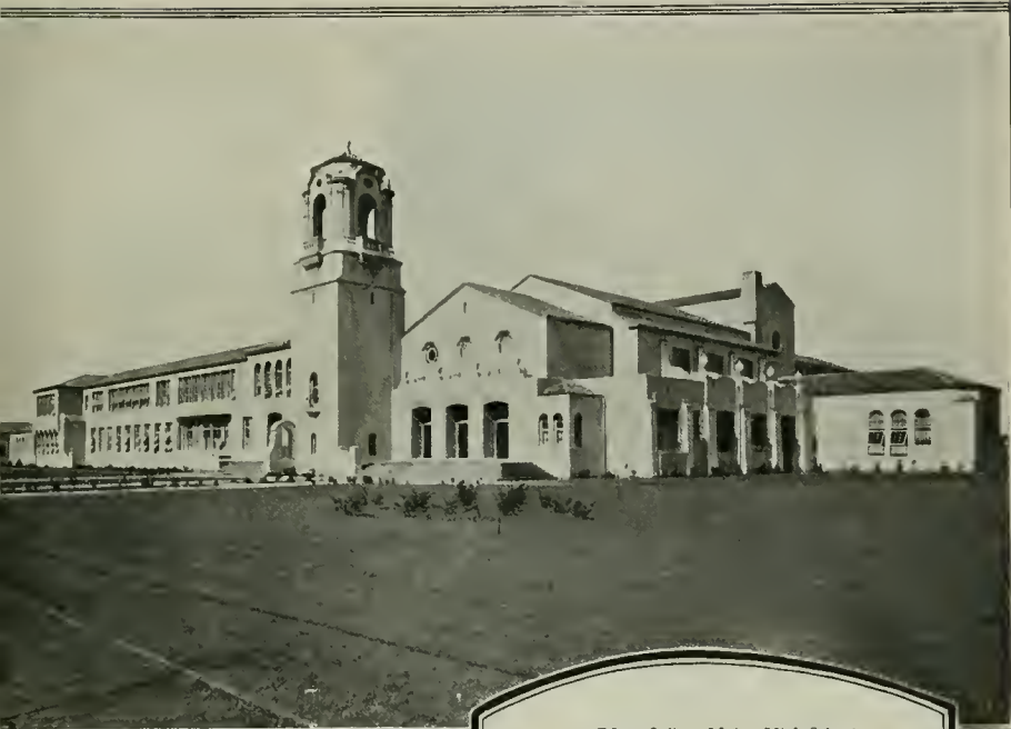
New Salinas Union High School Covered with a PABCO 20-Year Roof.
