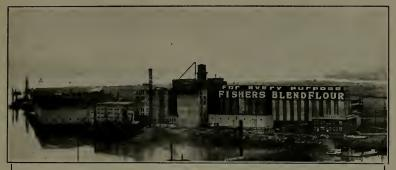
Fisher Flonring Mill, Seattle, Wash. 125 tons of black and galvanized Armeo Iron used for rooling, ventilators, bins, hoppers and chutes.
