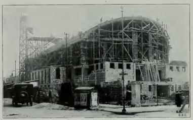
FIG. 7—FRONT AND WEST ELEVATIONS OF CHICAGO HEBREN INSTITUTE, SHOWING CONCRETE PLANT AND FORMS IN PLACE
