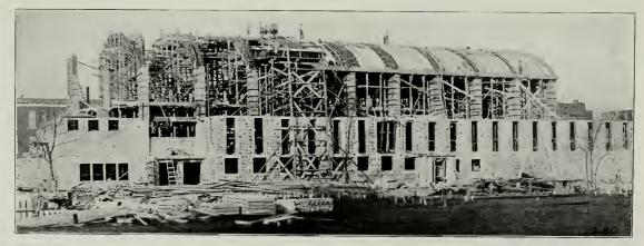
FIG. 6—EAST ELEVATION OF CHICAGO HEBREW INSTITUTE SHOWING ARCH AND ROOF-SLAB FORMS AND STAGING—VIEW ALSO SHOW'S MATERIAL CARRIAGE HOIST
