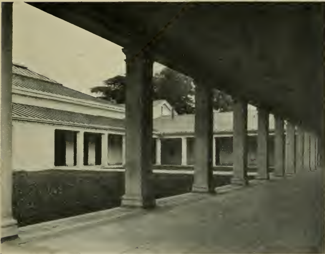
LOCKWOOD SCHOOL, SHOWING COURT, OAKLAND John J. Donovan and Lewis P. Hobart, Associate Architects
