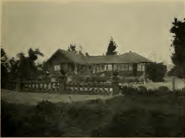
BUNGALOW OF MR. JOHN W. EDMINSON, PASADENA, CALIFORNIA B. Cooper Corbett, Architect
