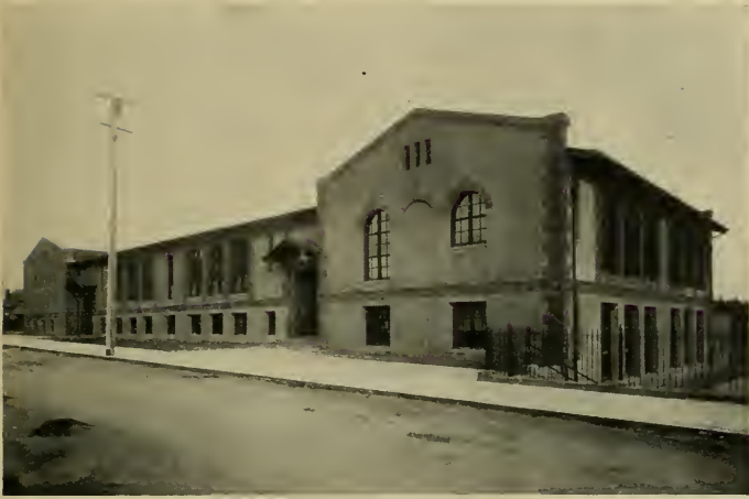
FRONT VIEW OF McCHESNEY SCHOOL, OAKLAND John J. Donovan, Architect
