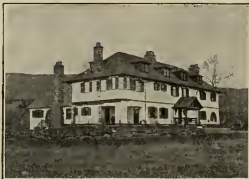
Residence of Thomas Shields Clarke, Esq., Lenox. Stained with Cabot's Shingle Stains and lined with Cabot's Sheathing Quilt for warmth. Wilson Eyre, Architect, Philadelphia.
