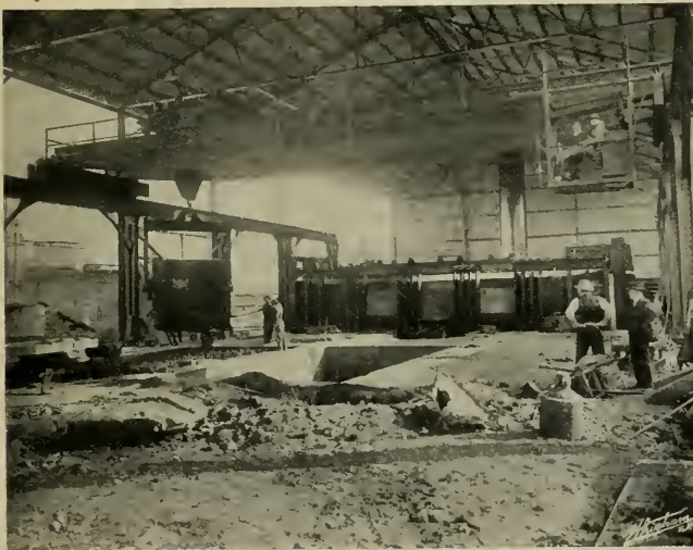
TWO VIEWS OF JUDSON MANUFACTURING COMPANY'S OPEN HEARTH FURNACES
