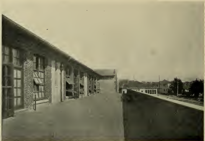
TERRACE, MCHESNEY SCHOOL, OAKLAND John J. Donovan, Architect
