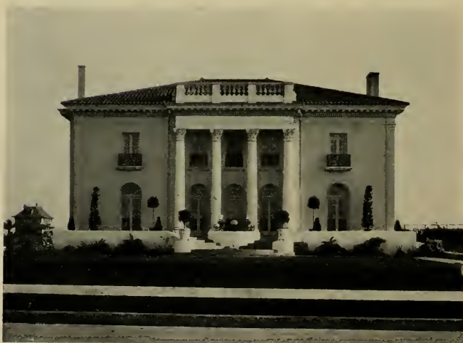
HOUSE OF MRS. LOUISE DENKER, LOS ANGELES B. Cooper Corbett, Architect
