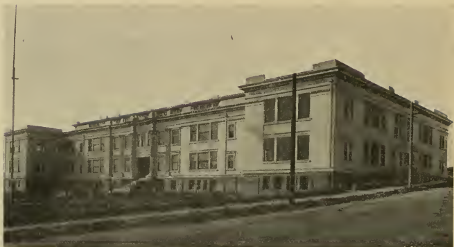
FREMONT HIGH SCHOOL, OAKLAND John J. Donovan, Architect
