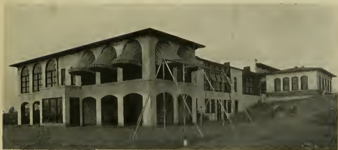
REAR VIEW OF CLEVELAND SCHOOL, OAKLAND John J. Donovan and Shafer & Wilde, Associate Architects
