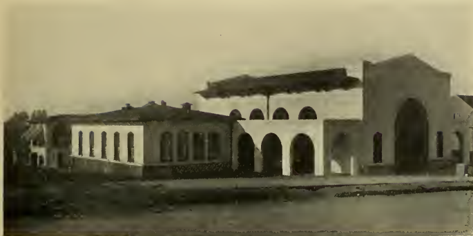
FRONT VIEW, CLEVELAND SCHOOL, OAKLAND John J. Donovan and Shafer & Wilde, Associate Architects
