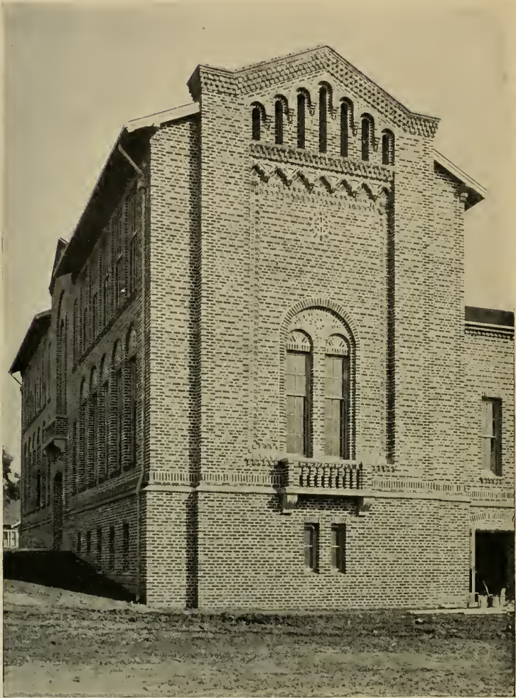
MALABAR SCHOOL—END DETAIL SHOWING EFFECTIVE BRICKWORK WITHEY & DAVIS, INC., ARCHITECTS
