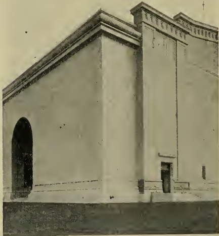
SECTION OF FRONT AND SIDE, OAKLAND AUDITORIUM From a photograph taken February 10th
