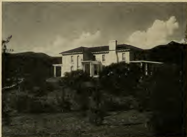
HOUSE OF MR. C. F. PERRY, HOLLYWOOD, CALIFORNIA B. Cooper Corbett, Architect
