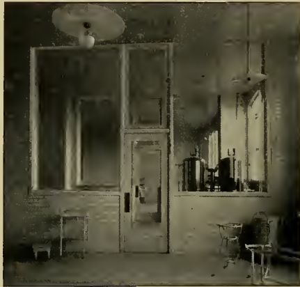
METAL DOORS AND TRIM IN SISTERS' HOSPITAL, BUFFALO, N. Y.
