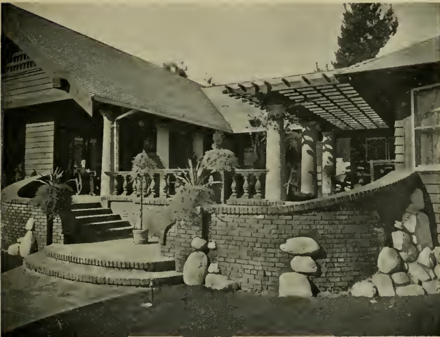
BRICK STEPS AND PORCH, EDMINSON BUNGALOW B. Cooper Corbett, Architect
