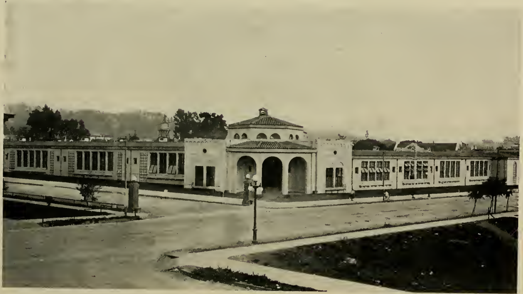
CLAREMONT SCHOOL, OAKLAND JOHN J. DONOVAN and } ASSOCIATE WALTER D. REED } ARCHITECTS
