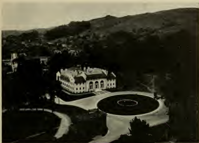
HEARST MEMORIAL MINING BUILDING, UNIVERSITY OF CALIFORNIA View from Sather Tower
