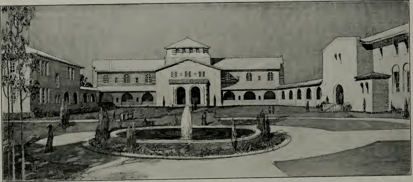
LIBRARY BUILDING—FRONT VIEW—CALIFORNIA STATE NORMAL SCHOOL, LOS ANGELES. ALLISON & ALLISON, ARCHITECTS
