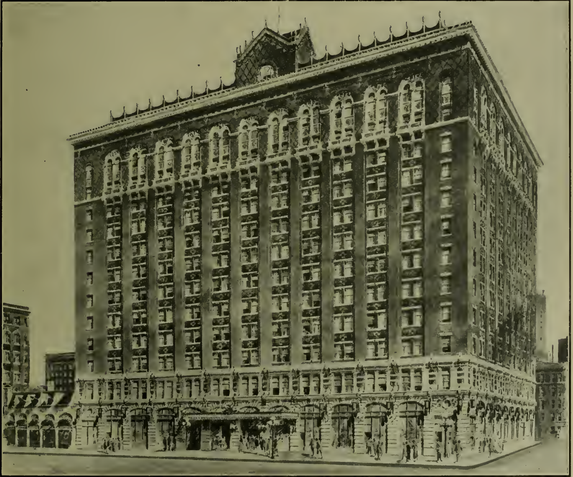
NEW DAVENPORT HOTEL, SPOKANE, WASHINGTON The First Two Stories of Boise Sandstone.
