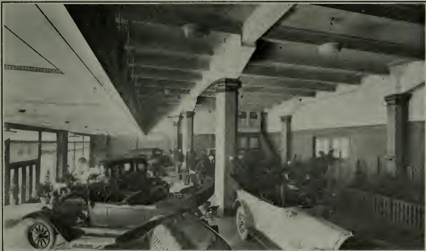
BUILDING FOR LOCOMOBILE COMPANY, SAN FRANCISCO Showing Heavy Concrete Beam and Girder Construction
