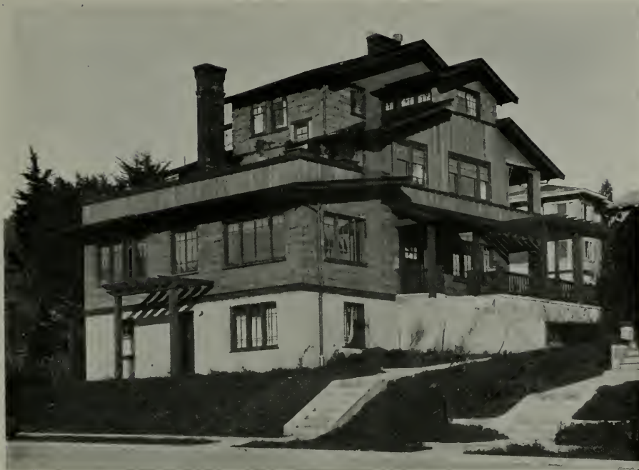
CONCRETE AND RUSTIC HOME, BERKELEY, CALIFORNIA Hughson & Donnelly, Builders
