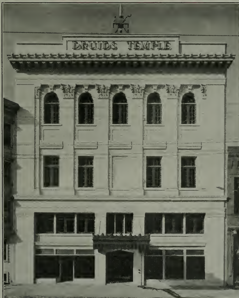
DRUIDS' TEMPLE, Page St., nr. Market, SAN FRANCISCO. E. P. Antonovich, Architect
