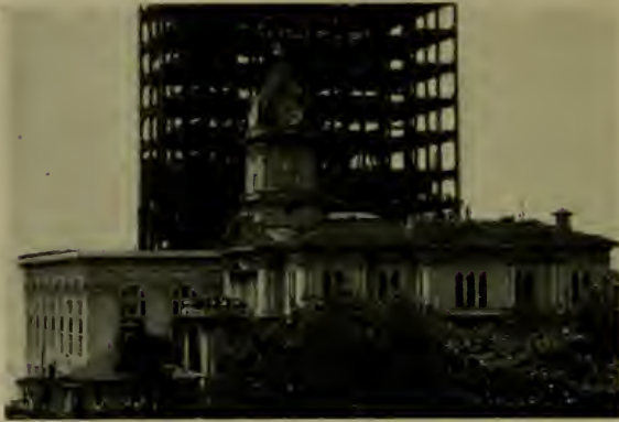
THE OLD OAKLAND CITY HALL, WITH STEEL FRAME OF NEW BUILDING IN BACKGROUND
