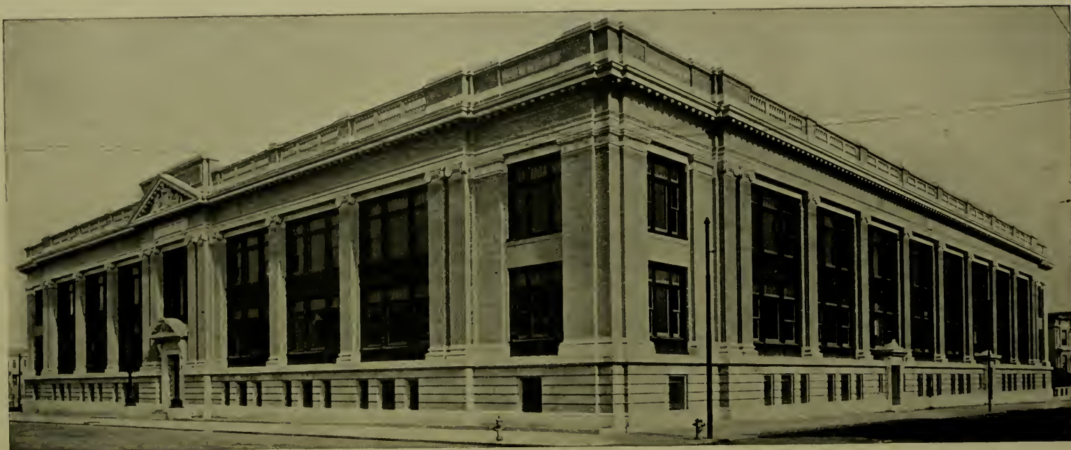
Built of semi-glazed architectural terra cotta and buff-colored brick.
