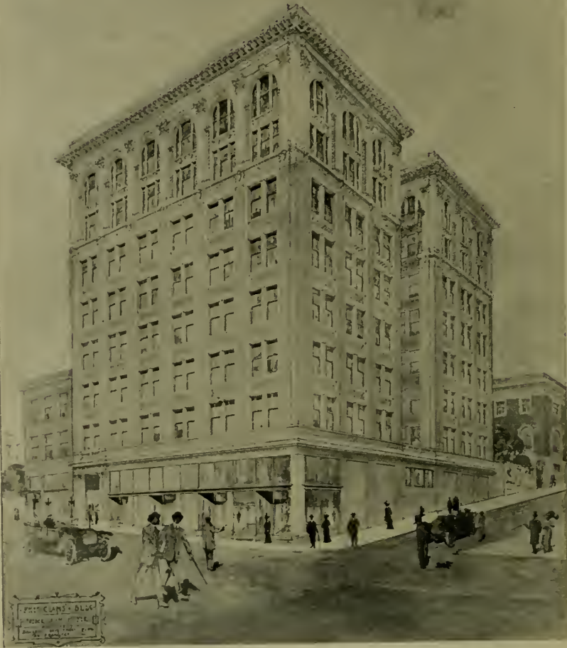
PHYSICIANS' BUILDING, SUTTER & POWELL STS., SAN FRANCISCO FREDERICK H. MEYER, Architect McLERAN & PETERSON, Contractors
