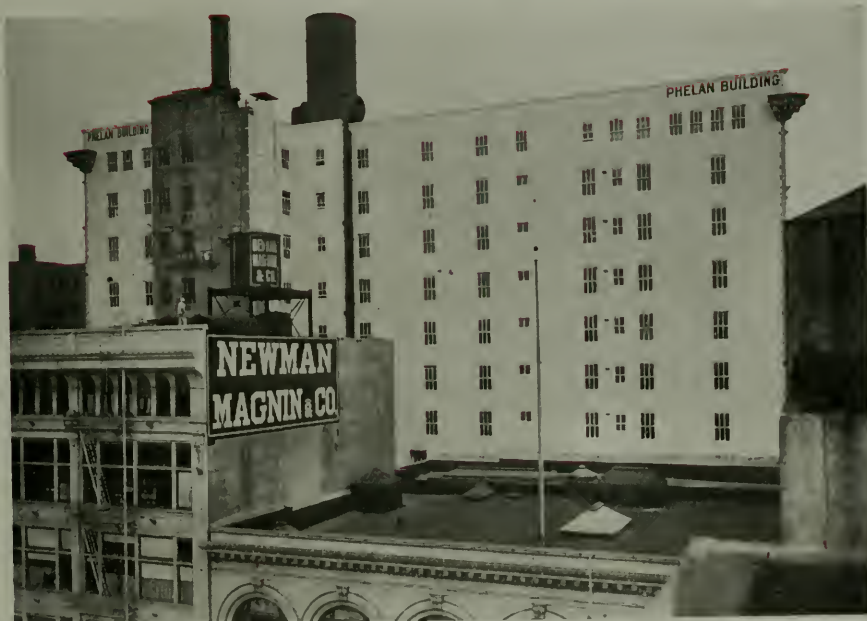
WEST WALL PHELAN BUILDING, SAN FRANCISCO Wm. Curlett & Son, Architects
