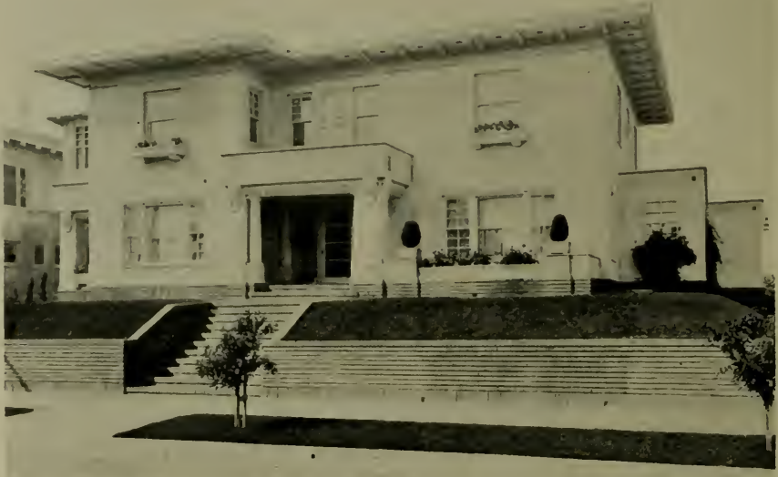
RESIDENCE OF ARCHITECT R. A. HEROLD, SACRAMENTO, CALIFORNIA
