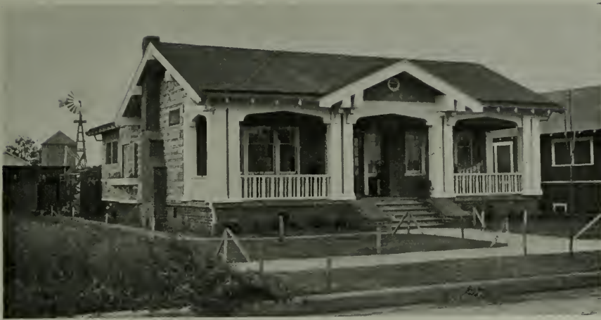
BUNGALOW FOR MR. J. M. SOUSA, MERCED, CALIFORNIA E. P. Antonovich, Architect
