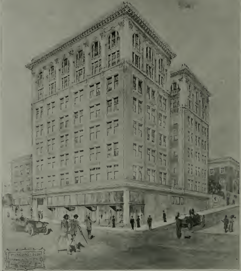
PHYSICIANS' BUILDING, SUTTER & POWELL STS., SAN FRANCISCO FREDERICK H. MEYER, Architect McLERAN & PETERSON, Contractors
