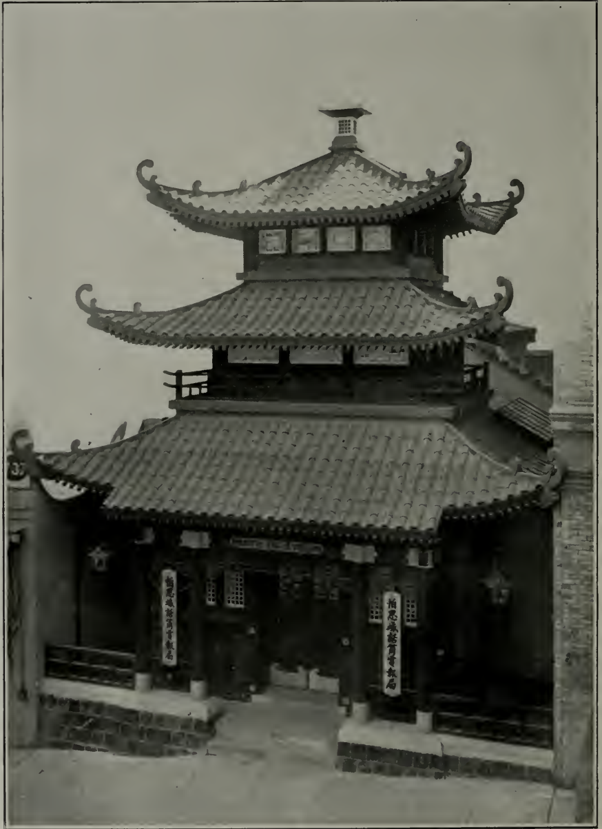
PACIFIC TELEPHONE COMPANY'S ORIENTAL EXCHANGE IN CHINATOWN, SAN FRANCISCO ENGINEERING DEPARTMENT, ARCHITECTS
