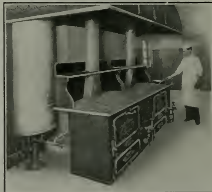
Crude Oil Burners Operating Kitchen Ranges in Government Barracks at Fort Winfield Scott
