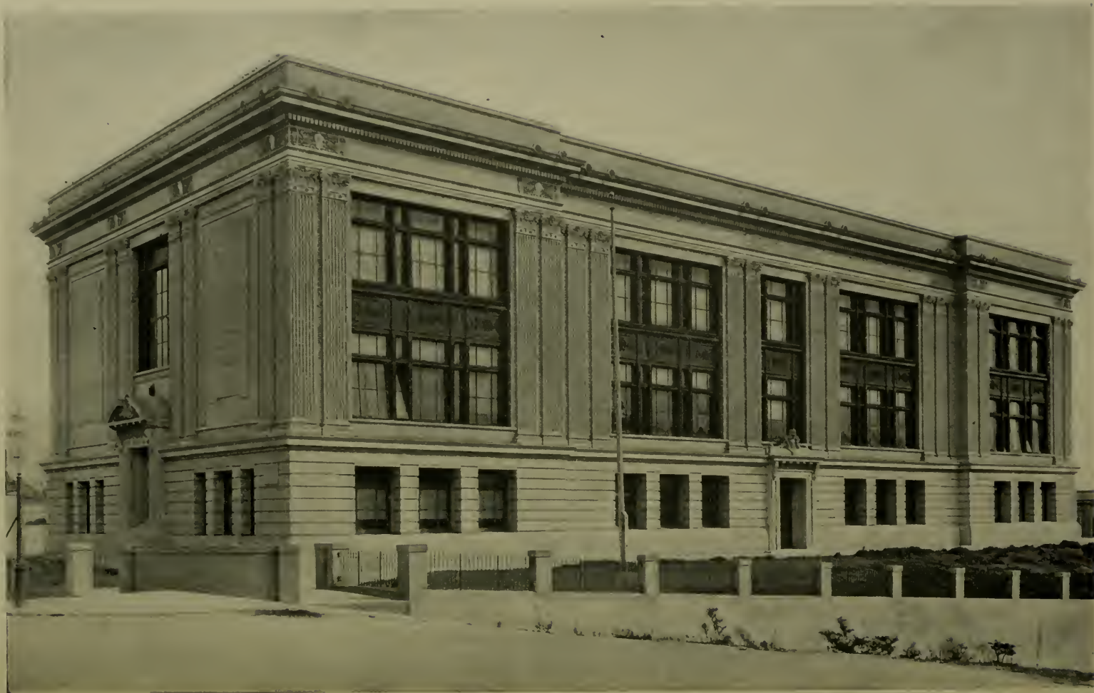
DENMAN SCHOOL BUILDING, SAN FRANCISCO DESIGNED BY THE CITY ARCHITECTS
