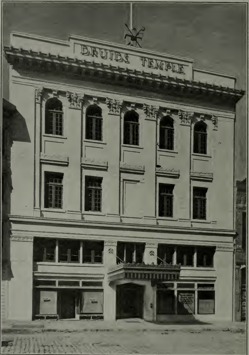
DRUIDS' TEMPLE, SAN FRANCISCO E. P. ANTONOVICH, ARCHITECT Golden Gate Cement Used
