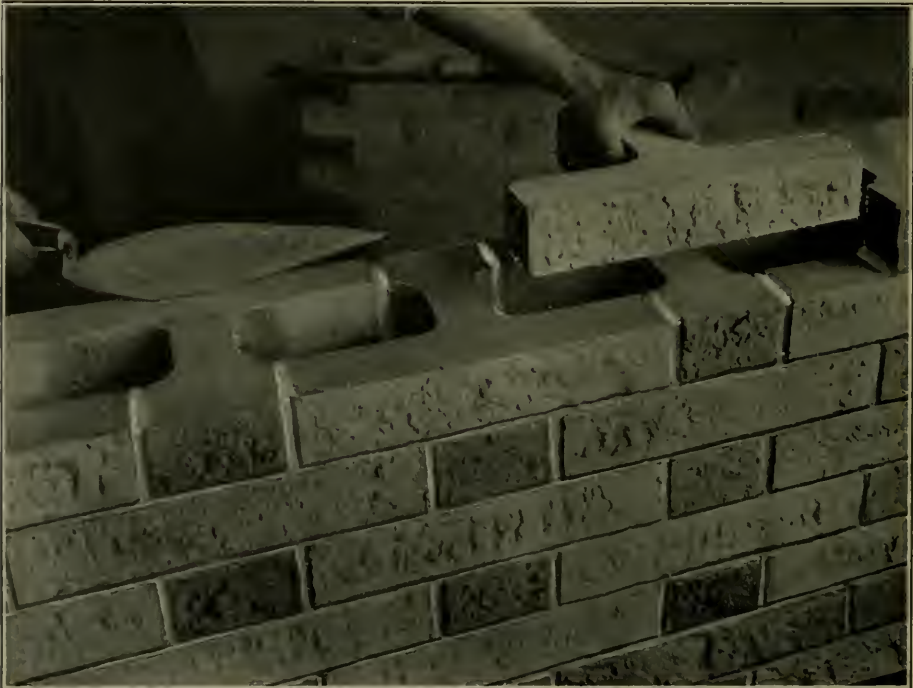
Fig. 13.—"An interesting version of an old well balanced Flemish bond." Can be laid twice as fast as ordinary Flemish walls.
