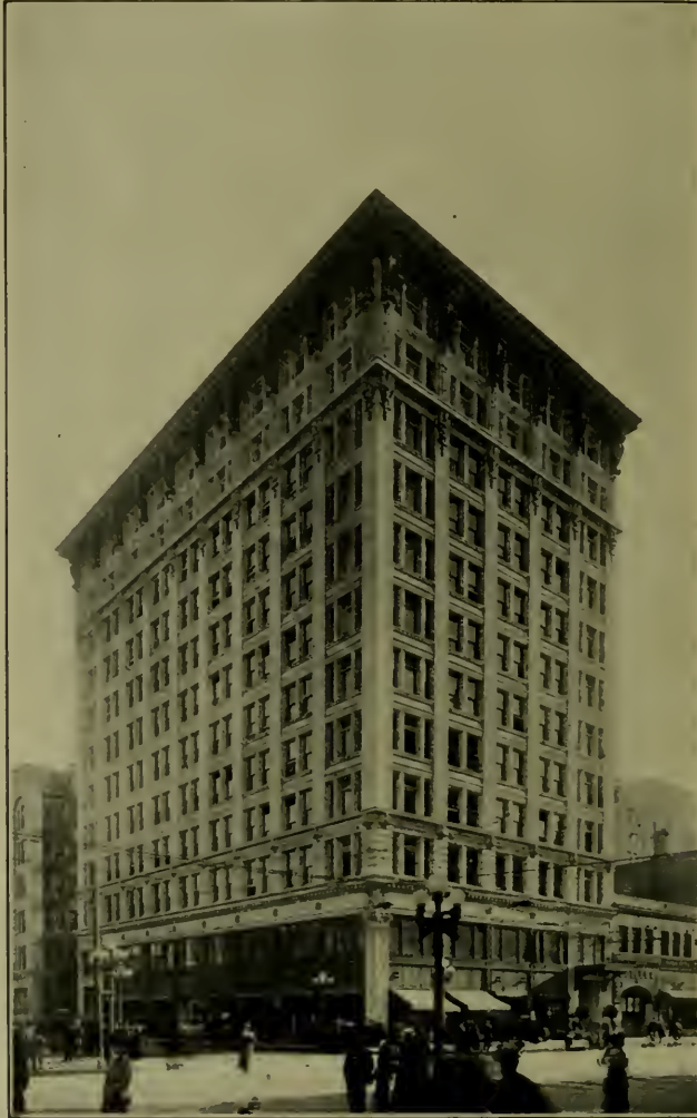
W. I. HOLLINGSWORTH BUILDING, LOS ANGELES MORGAN, WALLS & MORGAN, ARCHITECTS Faced with Los Angeles Pressed Brick Company's Enamel Brick.
