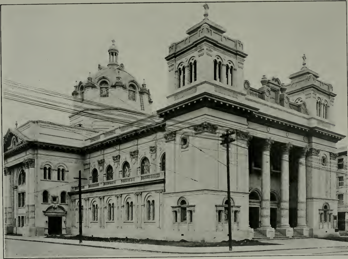
FIRST METHODIST CHURCH, OAKLAND, EXTERIOR FACED WITH SACRAMENTO SANDSTONE BRICK. NORMAN F. MARSH, ARCHITECT
