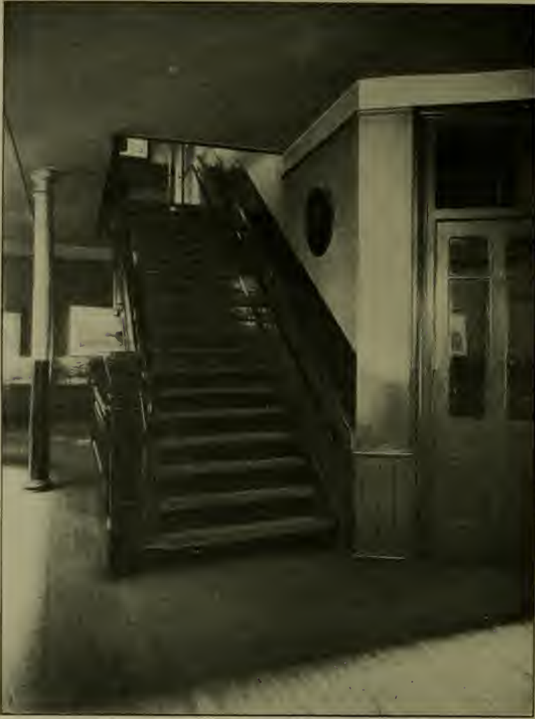
A TYPICAL SCHOOL STAIRWAY EQUIPPED WITH UNIVERSAL SAFETY TREADS
