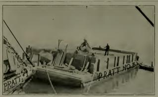
Unloading part of a 5,000 yard (equal to 200 car loads) order of washed gravel with clam shell bucket at Bolinas Boy for the J. G. White Engineering Corporation
