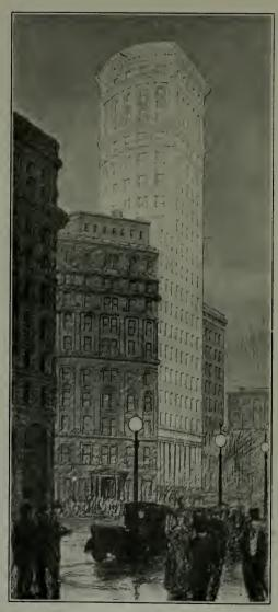
BUILDING FOR THE HOBART ESTATE, SAN FRANCISCO, WILLIS POLK & CO . ARCHITECTS. THIS WILL BE SAN FRANCISCO'S TALLEST OFFICE BUILDING-HEIGHT 22 STORIES, EQUAL TO 278 FEET. OVER 1800 TONS OF STRUCTURAL STEEL WILL BE USED. THERE WILL BE 310 OFFICES THE EXTERIOR WILL BE OF GRANITE. TERRA COTTA AND BRICK AND THE ESTIMATED COST IS \$1.000,000.
